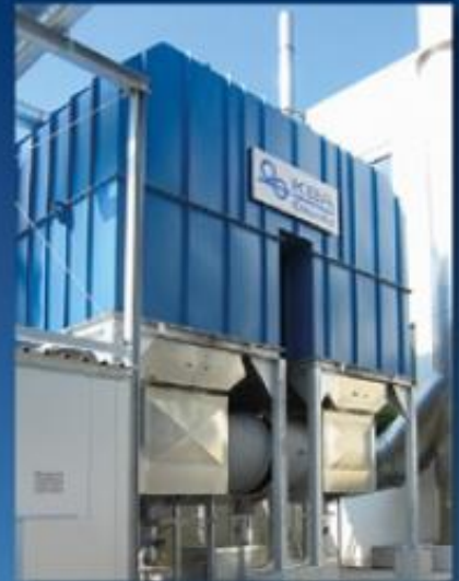
Automotive industry: RTO 50 000/2X for 8 spray booths.
