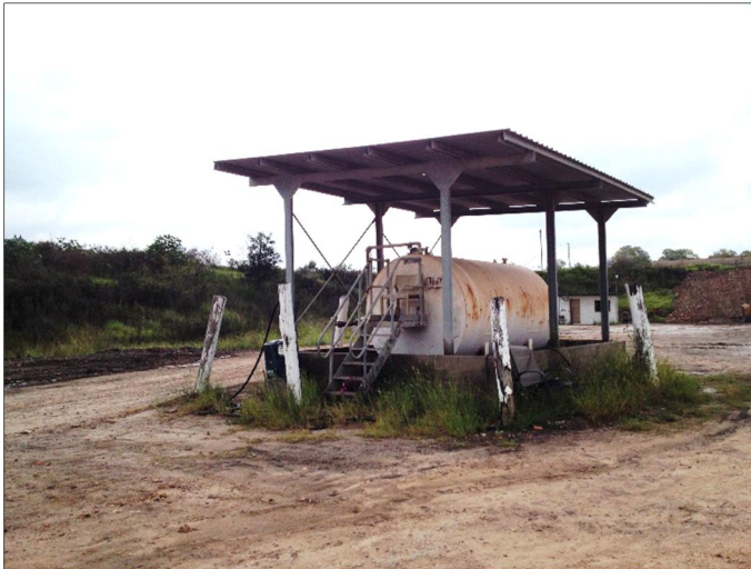
Photograph indicating the diesel tank within the proposed new stockpiles area.
