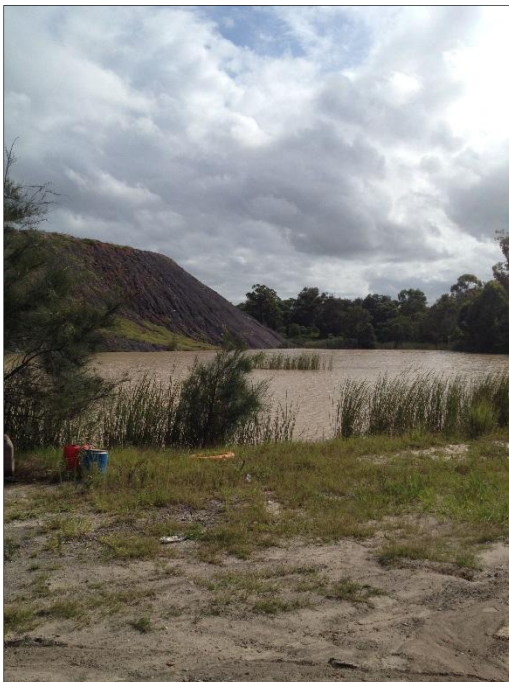
Photograph looking west across the detention basin showing the large stockpile (approx. 30m high) located to the south of the basin.
