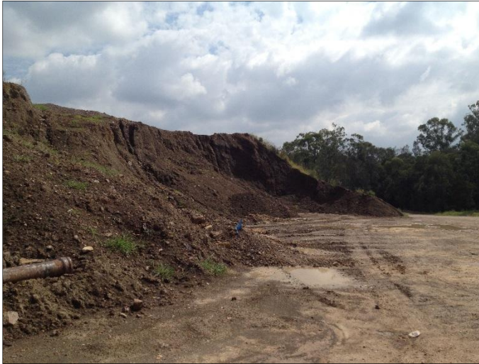
Photograph looking north at the road and stockpile in the vicinity of the proposed roadways, truck loading, staff office, carpark and truck parking area.
