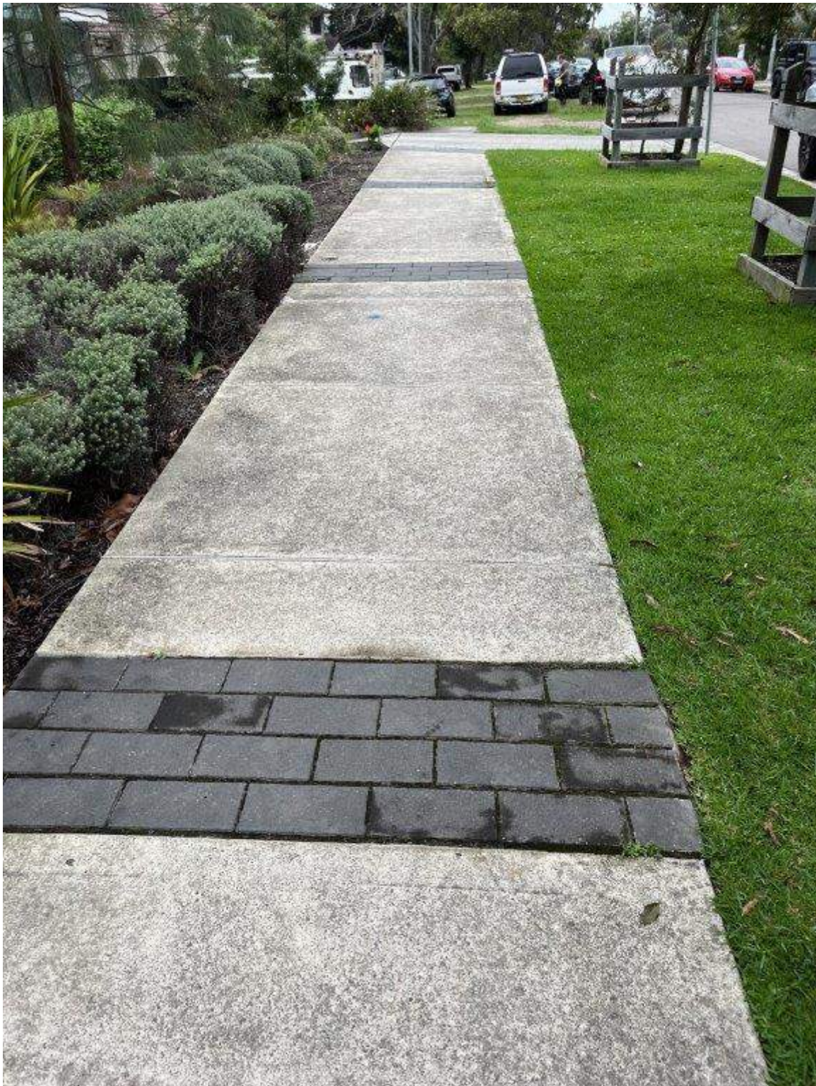
Photo 14 - Hinkler Avenue - Existing condition of pavement and vegetation
