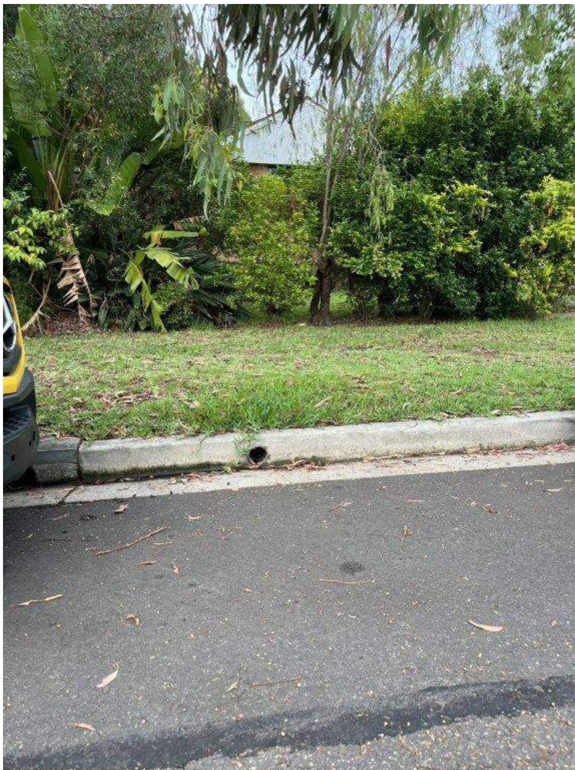
Photo 173 - Taren Point Road - Existing condition of pavement and vegetation
