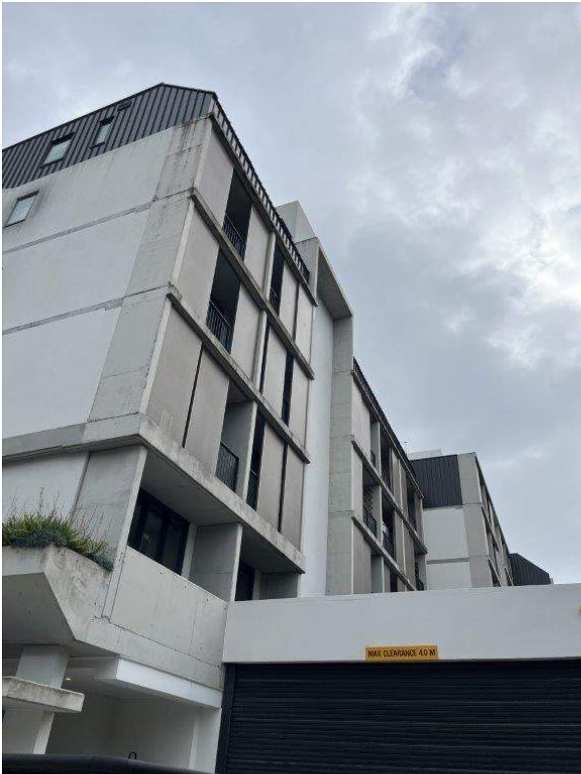
Photo 1 - Hinkler Avenue - Existing condition of external facade
