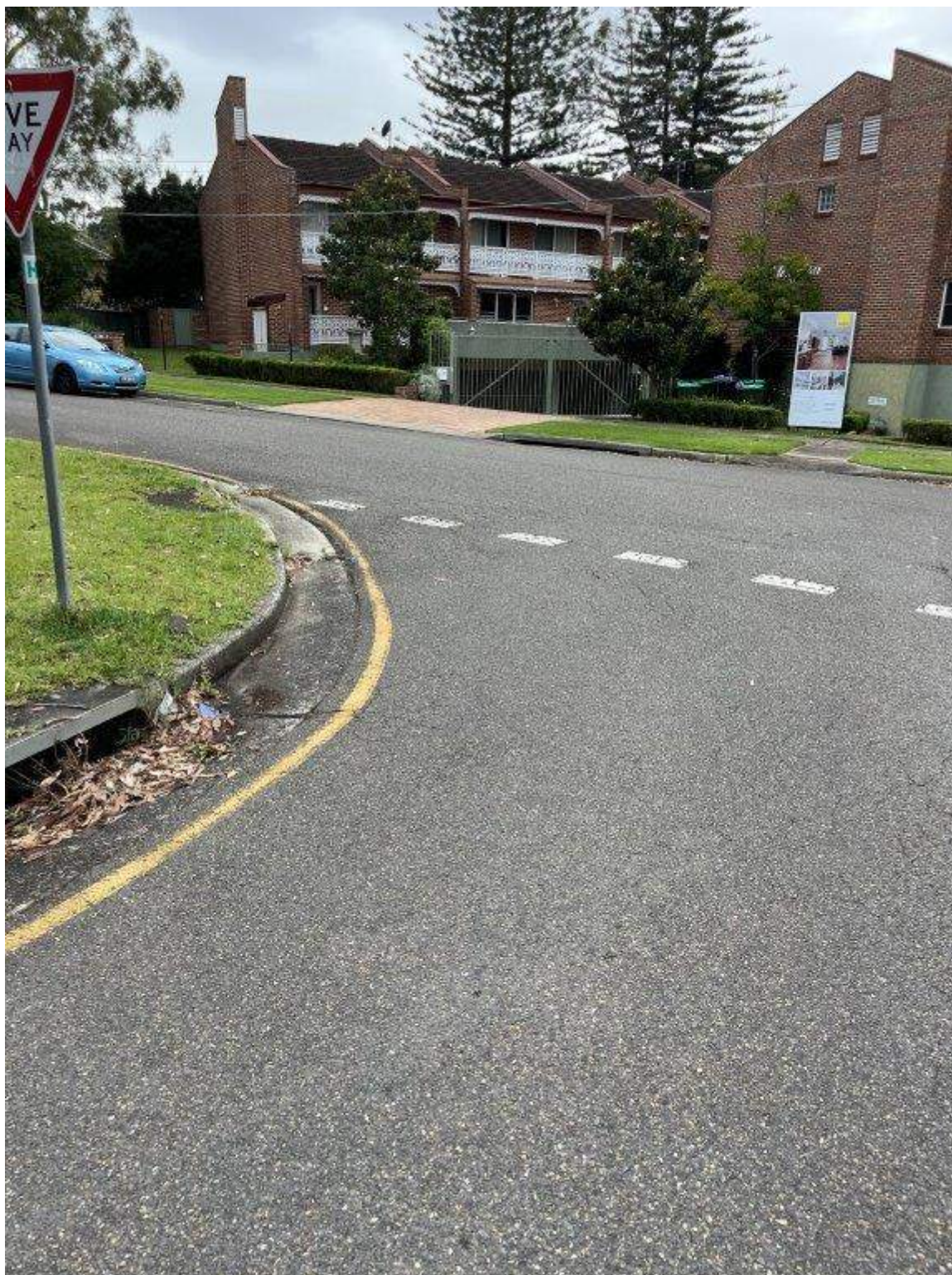
Photo 139 - Hinkler Avenue - Existing condition of pavement and vegetation
