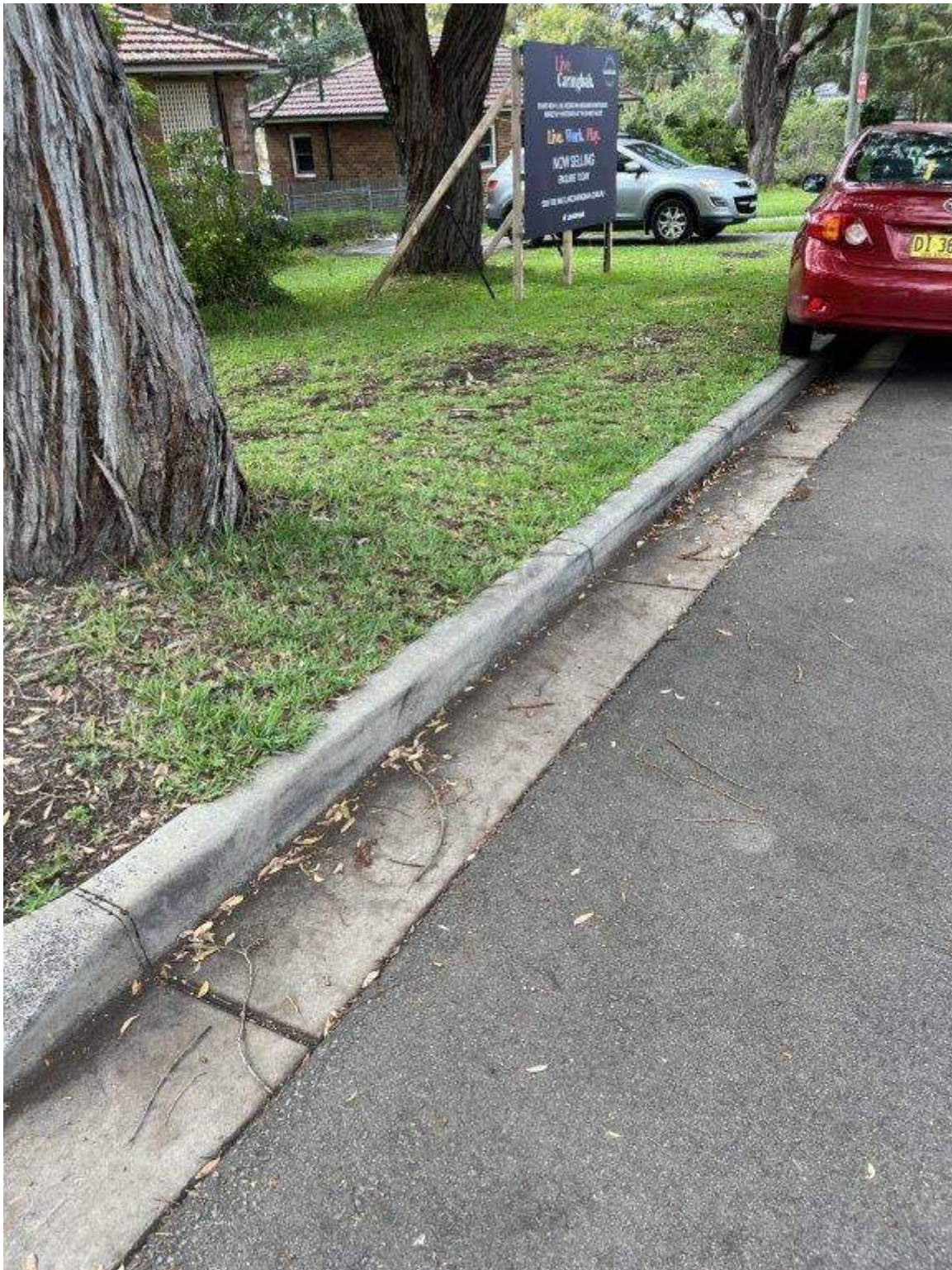
Photo 95 - Hinkler Avenue - Existing condition of pavement and vegetation
