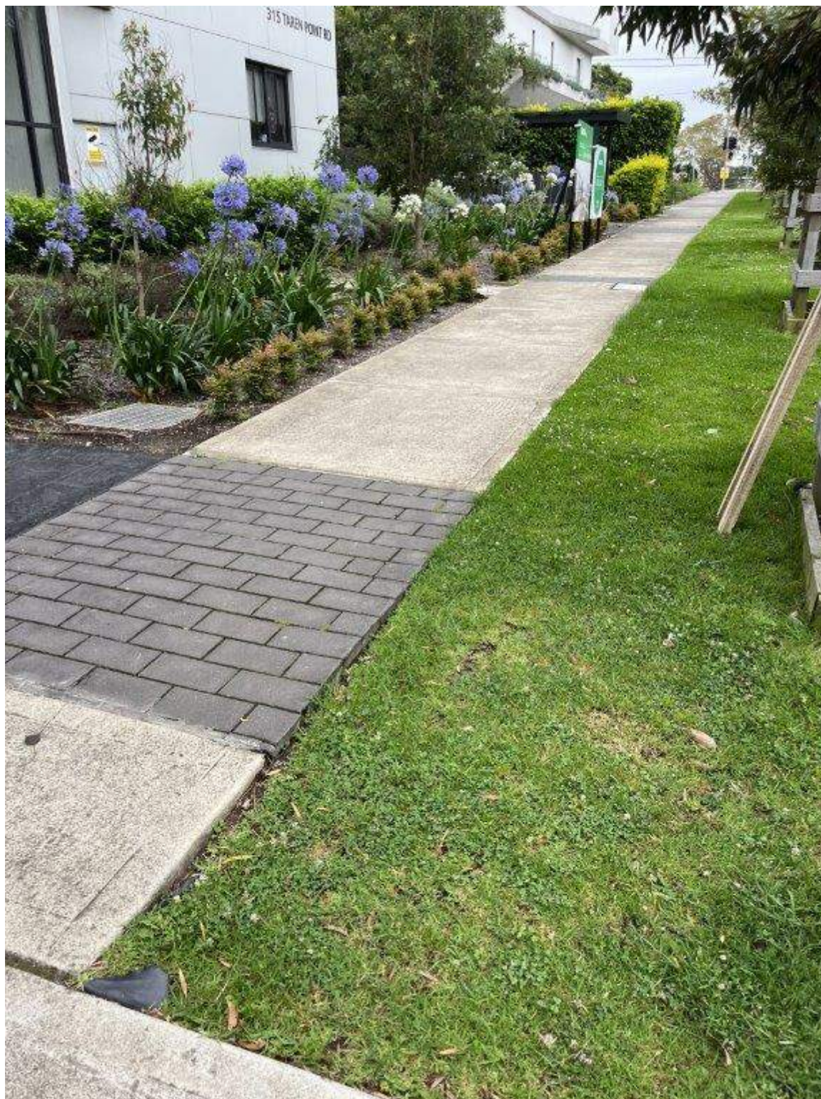
Photo 244 - Taren Point Road - Existing condition of pavement and vegetation
