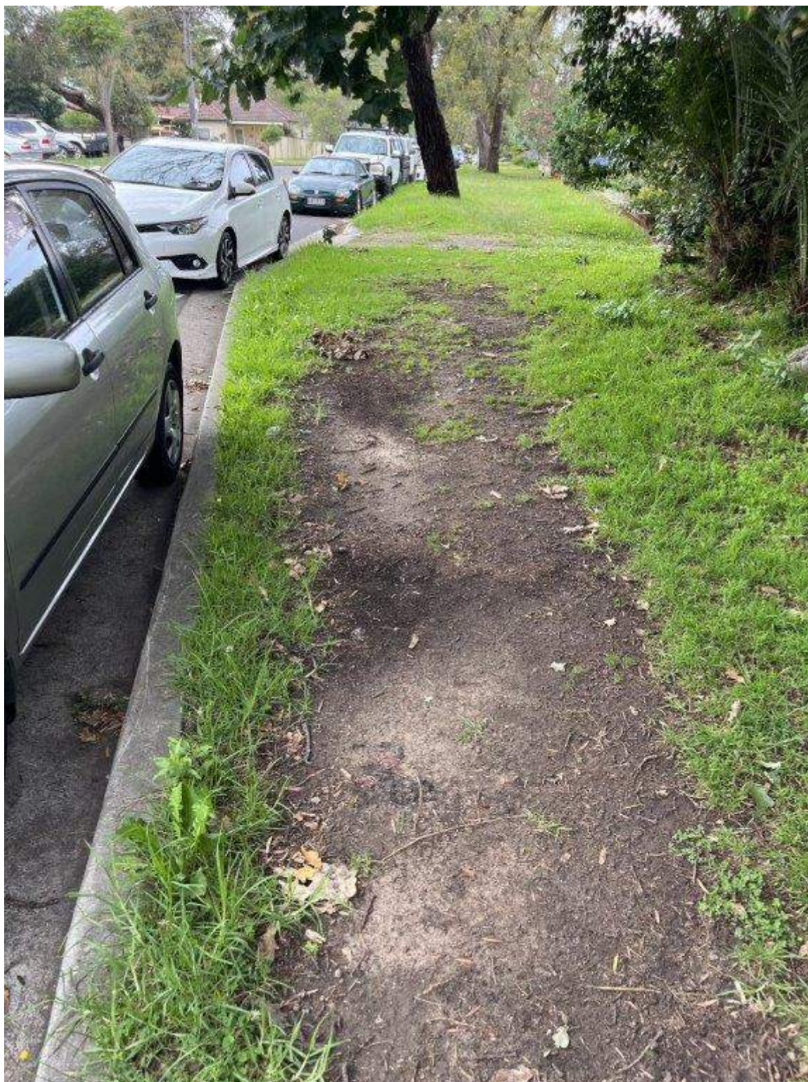
Photo 253 - Taren Point Road - Existing condition of vegetation
