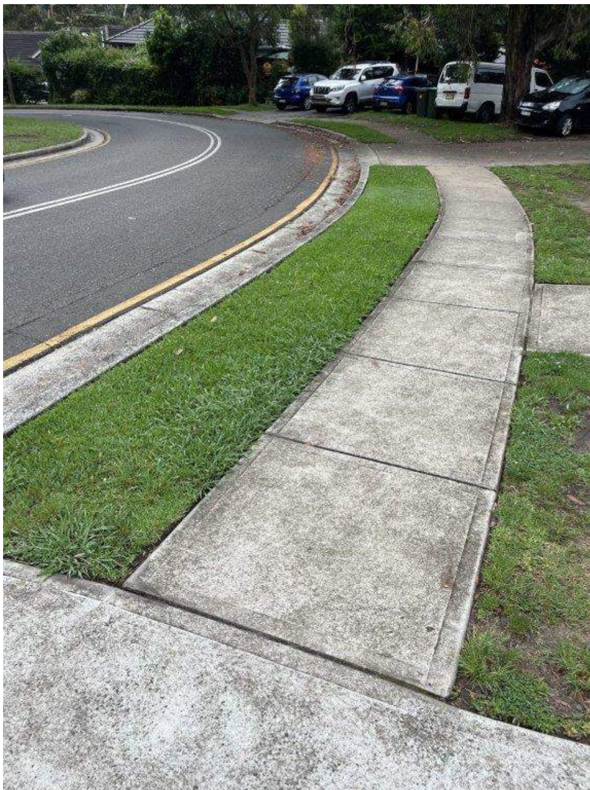
Photo 107 - Hinkler Avenue - Existing condition of pavement and vegetation
