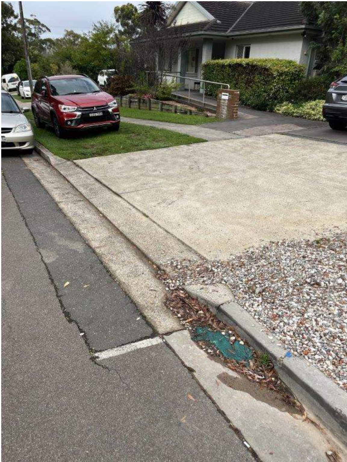
Photo 87 - Hinkler Avenue - Existing condition of pavement
