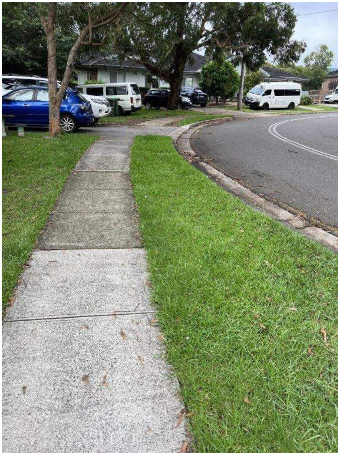
Photo 126 - Hinkler Avenue - Existing condition of pavement and vegetation
