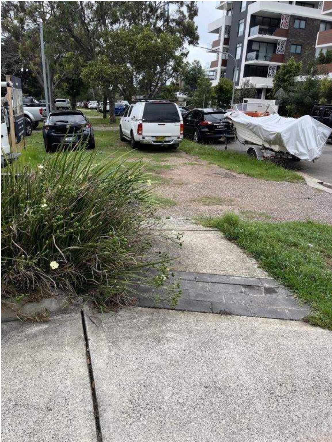
Photo 27 - Hinkler Avenue - Existing condition of pavement and vegetation
