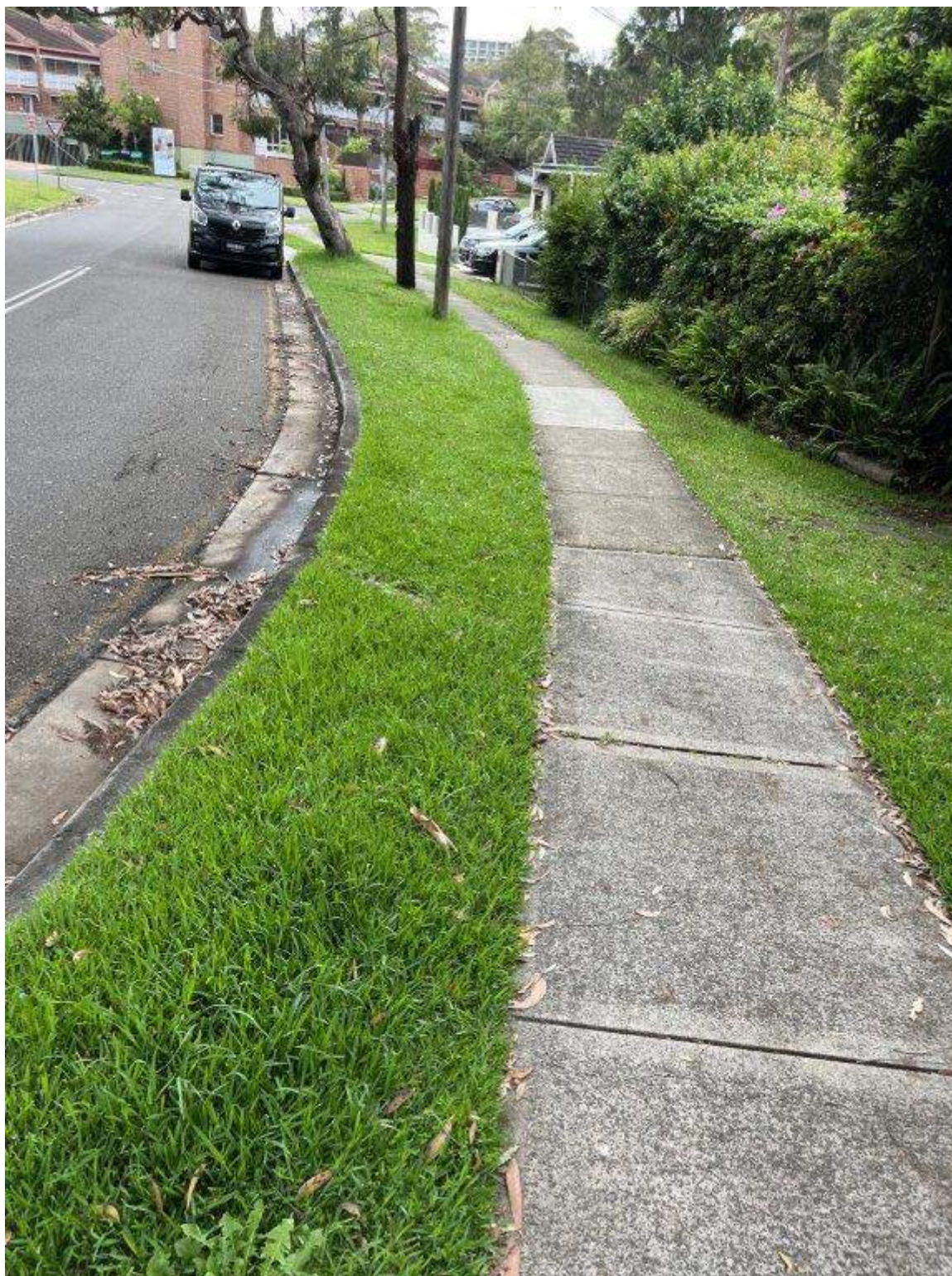
Photo 119 - Hinkler Avenue - Existing condition of pavement and vegetation
