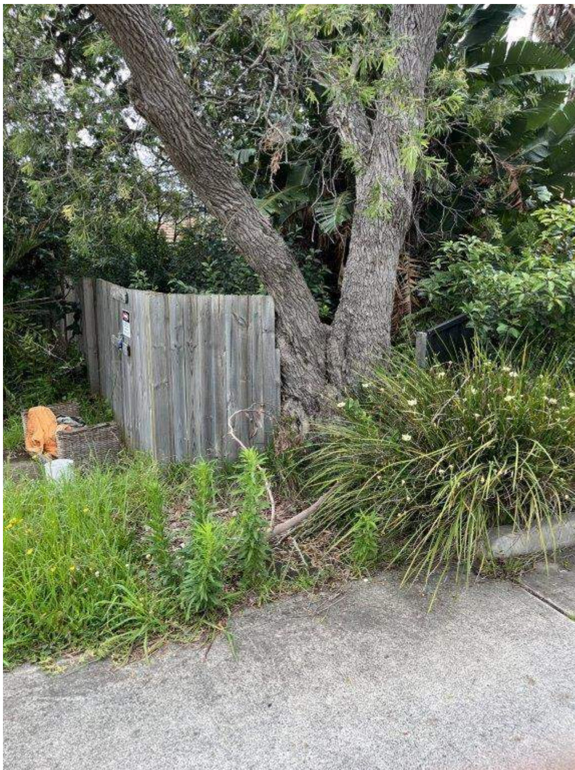
Photo 248 - Taren Point Road - Existing condition of pavement and vegetation
