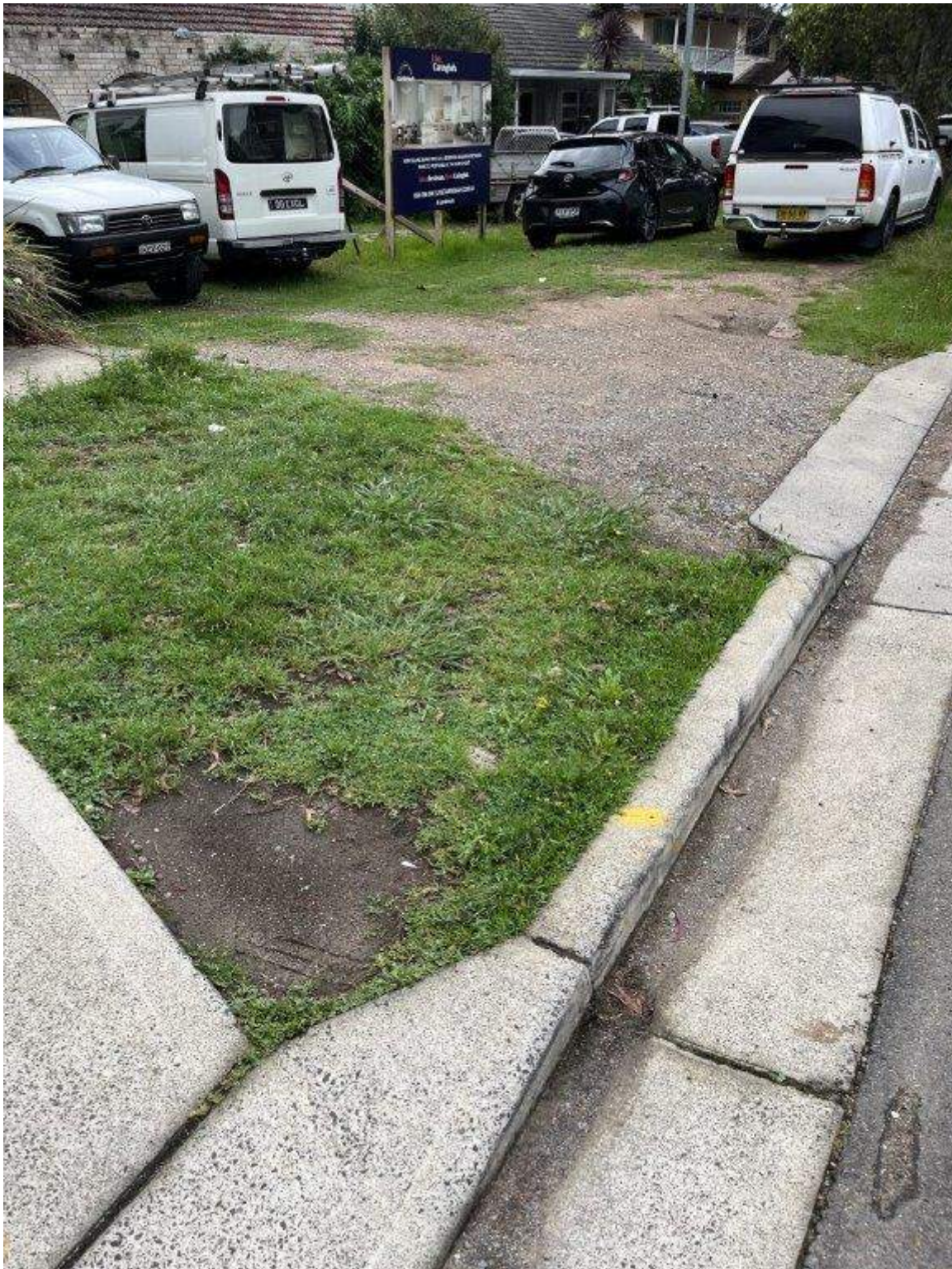
Photo 21 - Hinkler Avenue - Existing condition of pavement and vegetation
