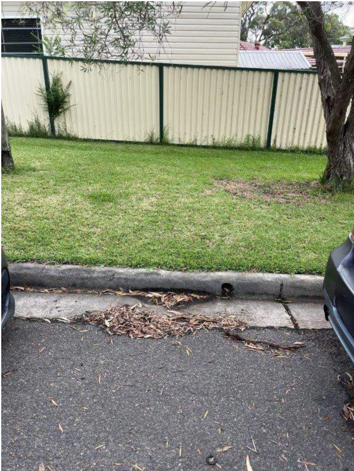
Photo 178 - Taren Point Road - Existing condition of pavement and vegetation
