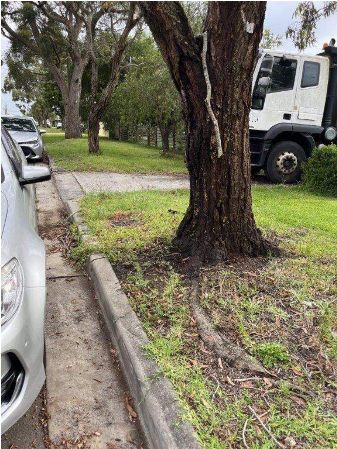
Photo 83 - Hinkler Avenue - Existing condition of pavement and vegetation
