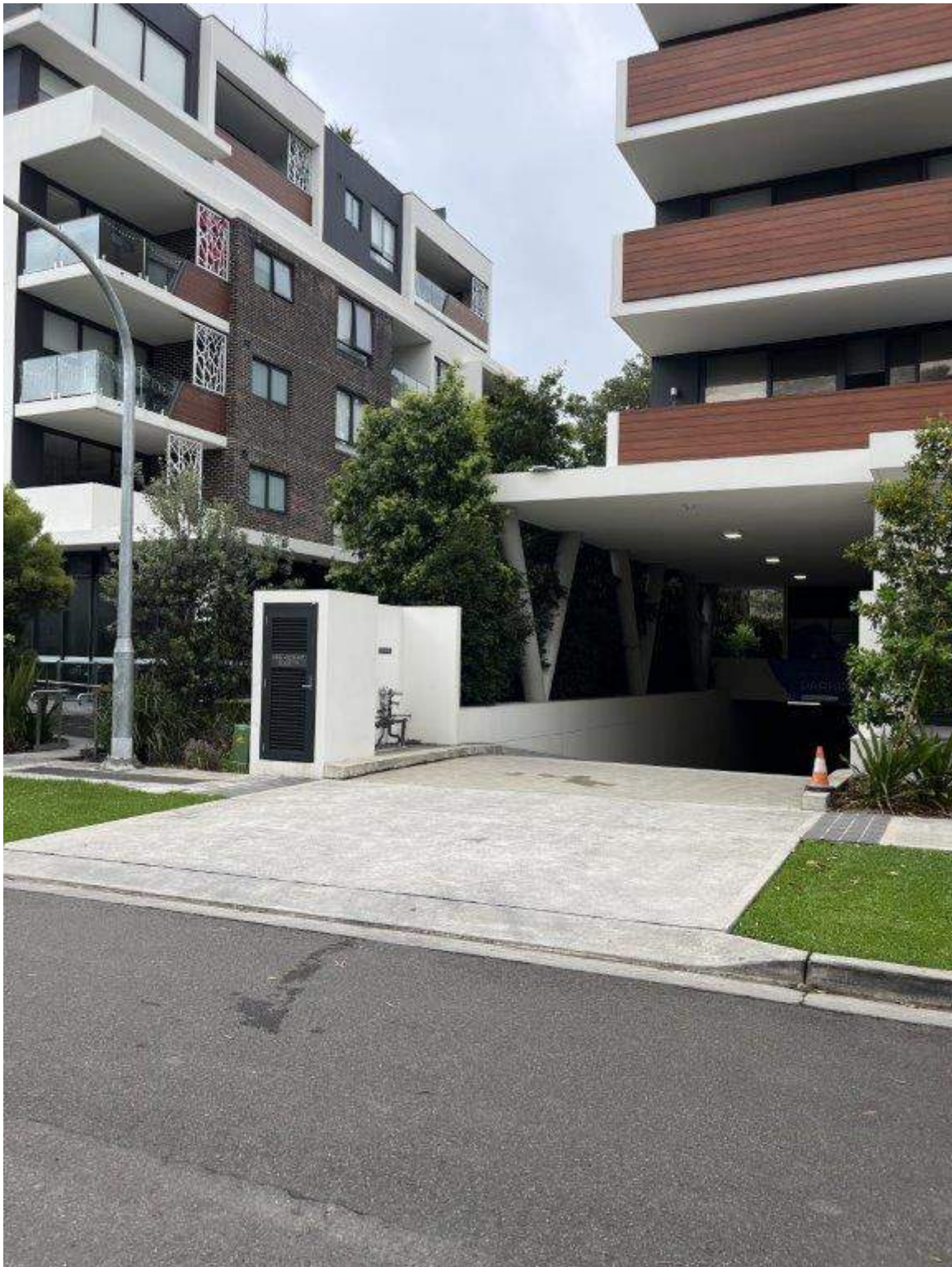
Photo 36 - Hinkler Avenue - Existing condition of pavement
