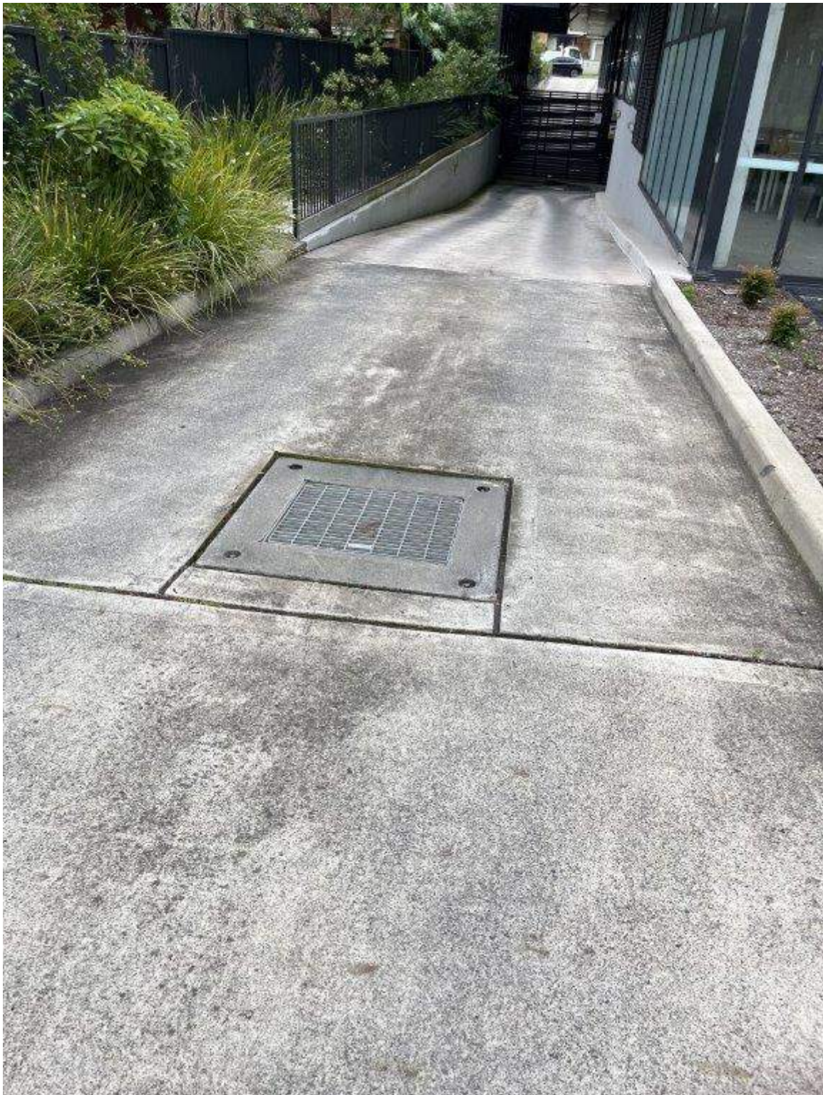
Photo 247 - Taren Point Road - Existing condition of pavement and steel grate
