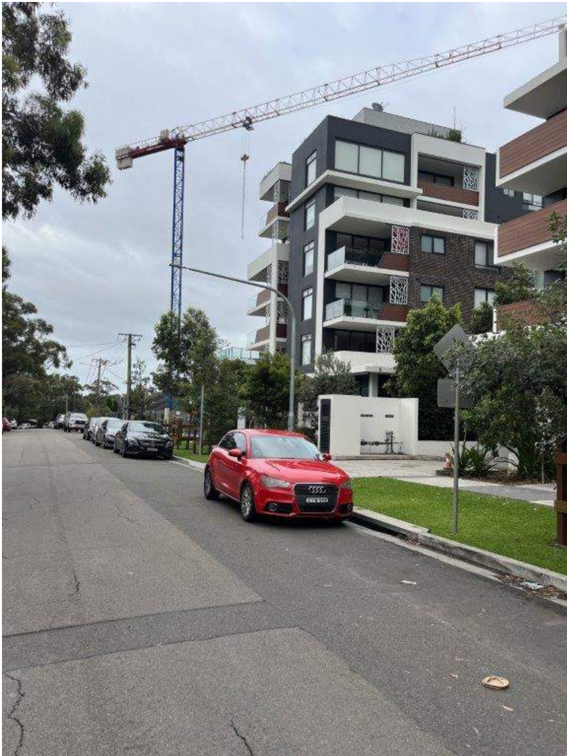
Photo 30 - Hinkler Avenue – Existing condition of pavement
