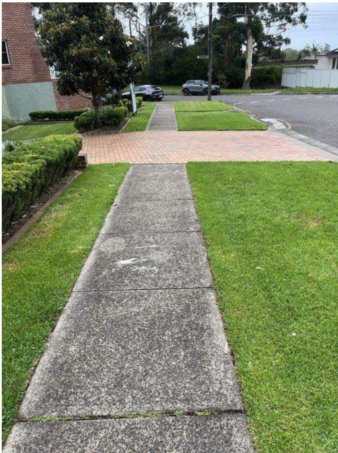
Photo 155 - Taren Point Road - Existing condition of pavement and vegetation
