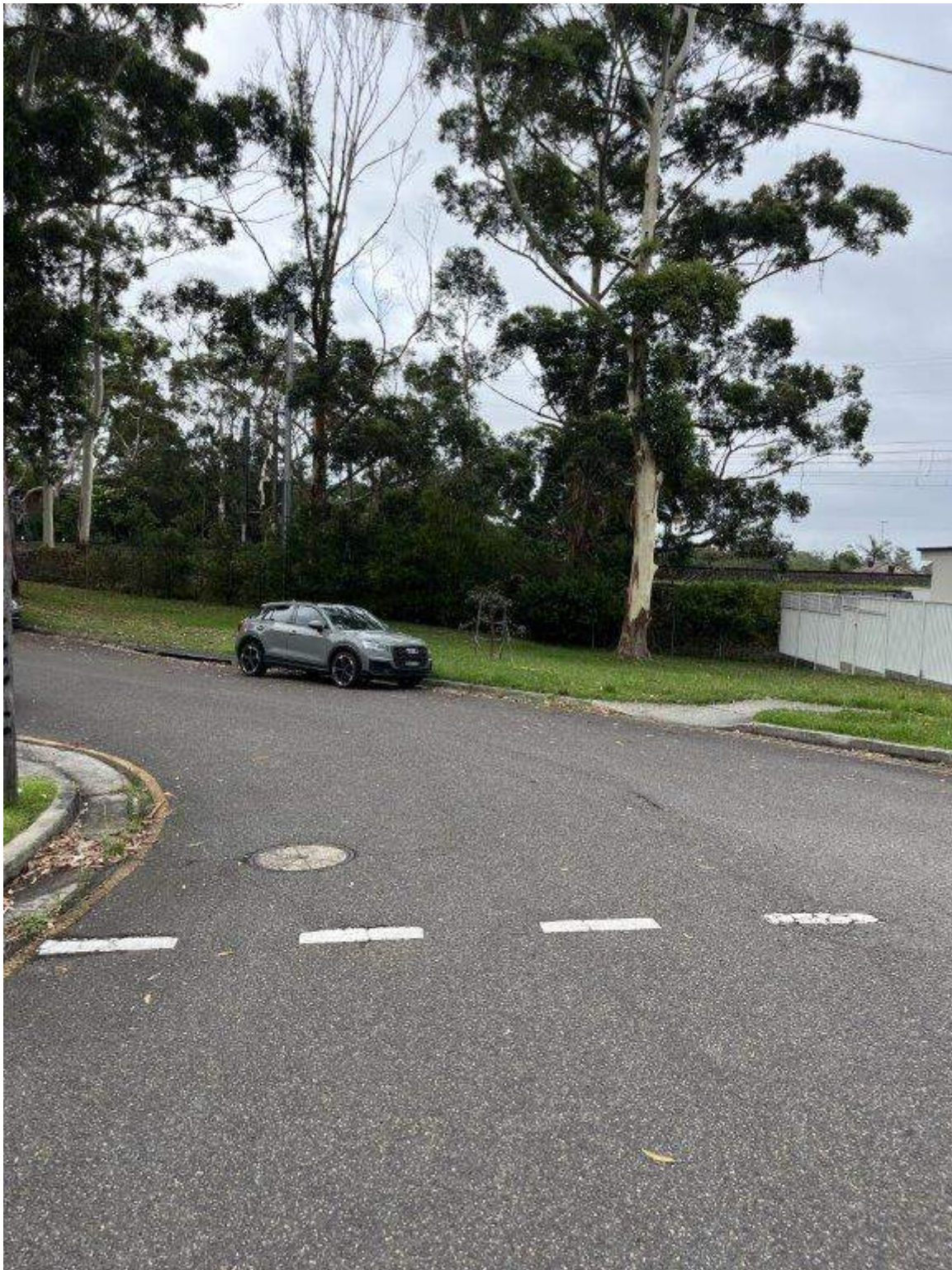
Photo 142 - Taren Point Road - Existing condition of pavement and manhole
