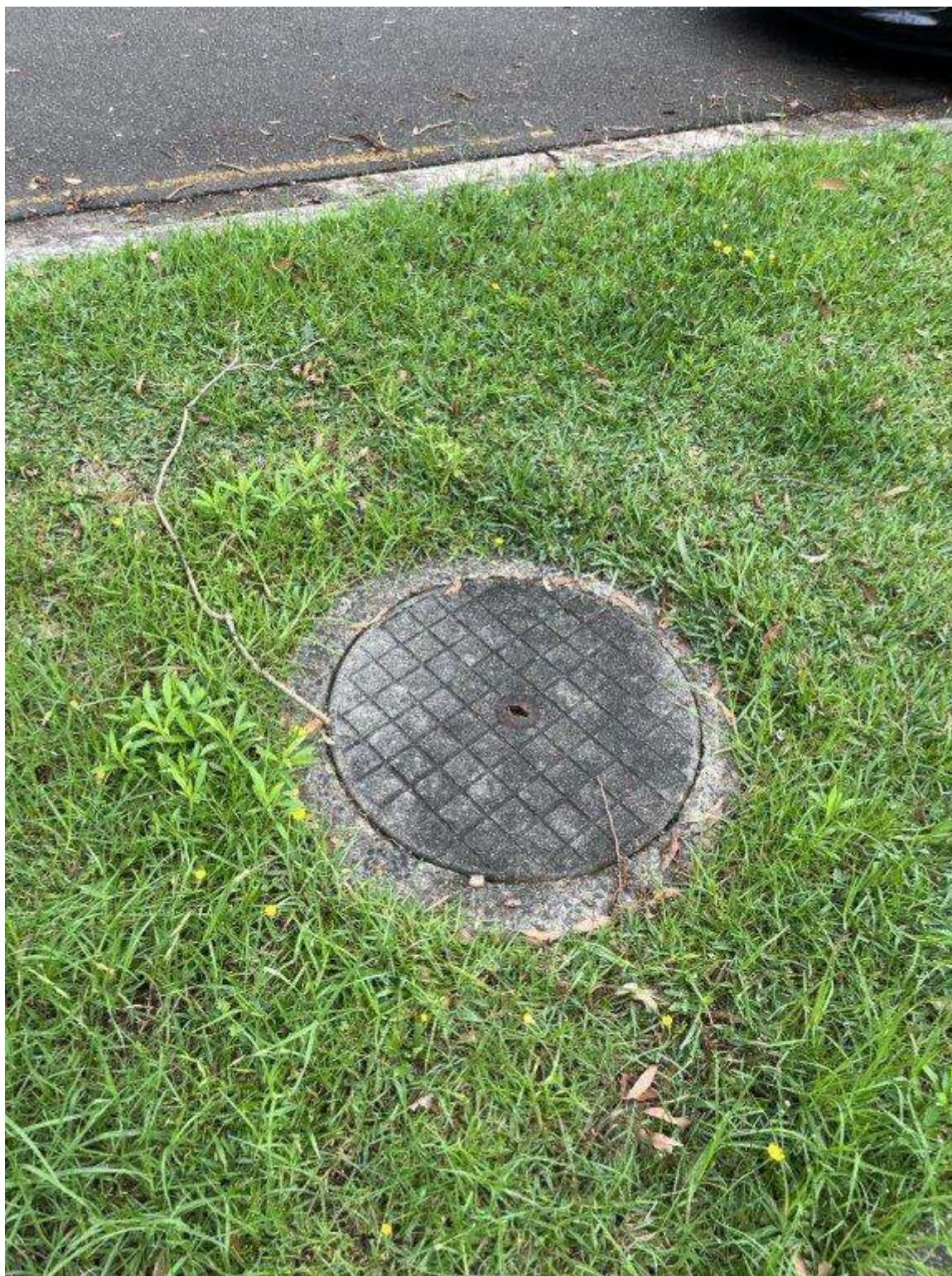
Photo 129 - Hinkler Avenue - Existing condition of manhole
