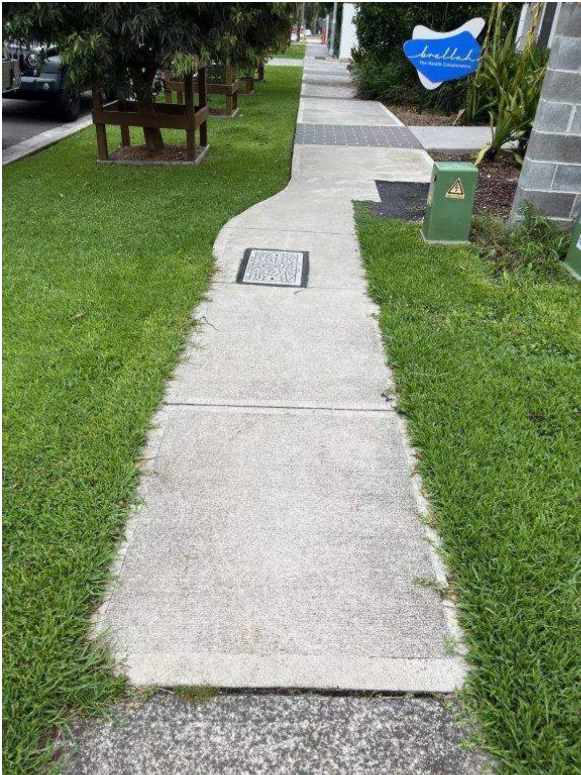
Photo 45 - Hinkler Avenue - Existing condition of pavement and vegetation
