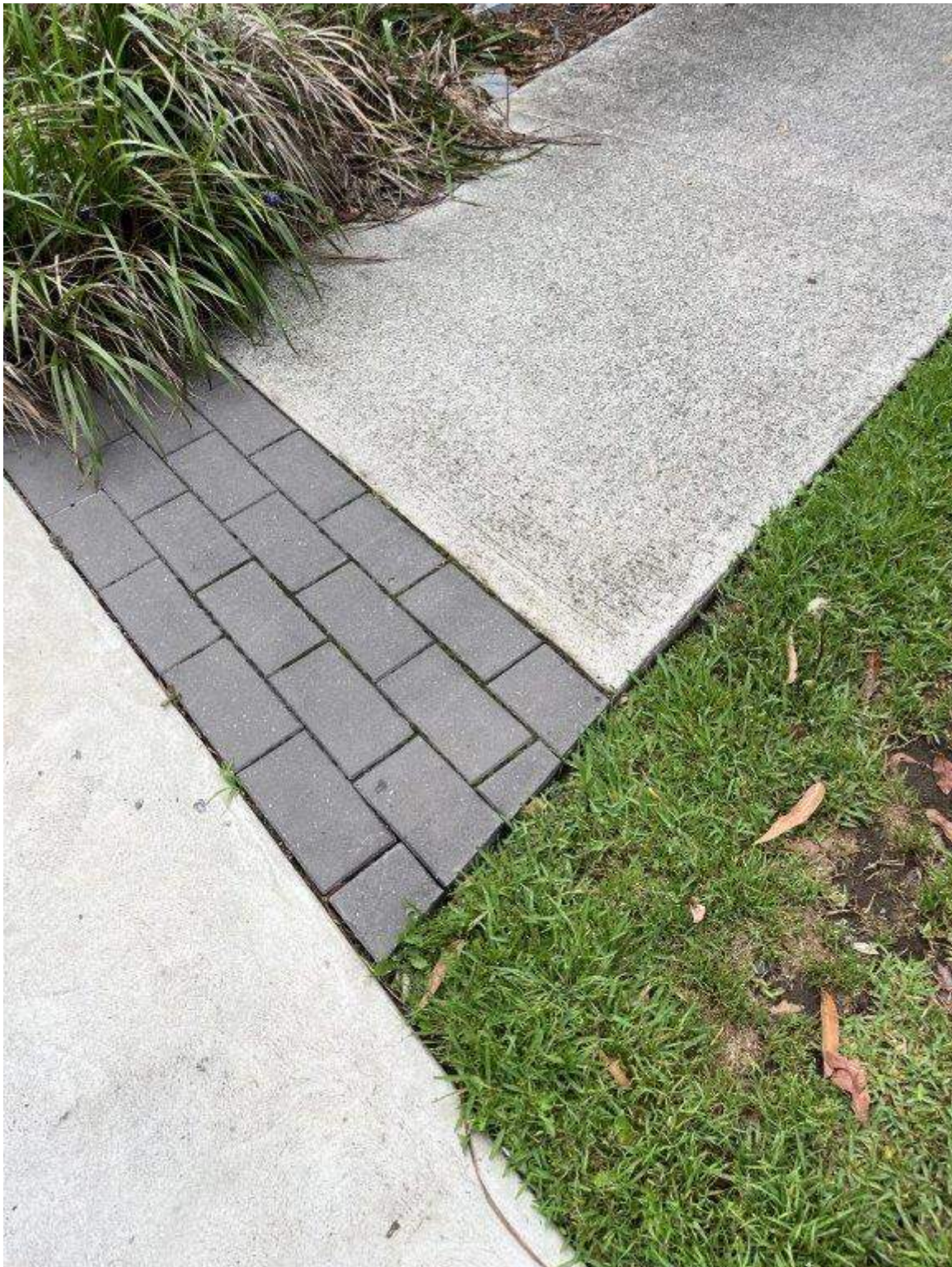
Photo 4 - Hinkler Avenue - Existing condition of pavement
