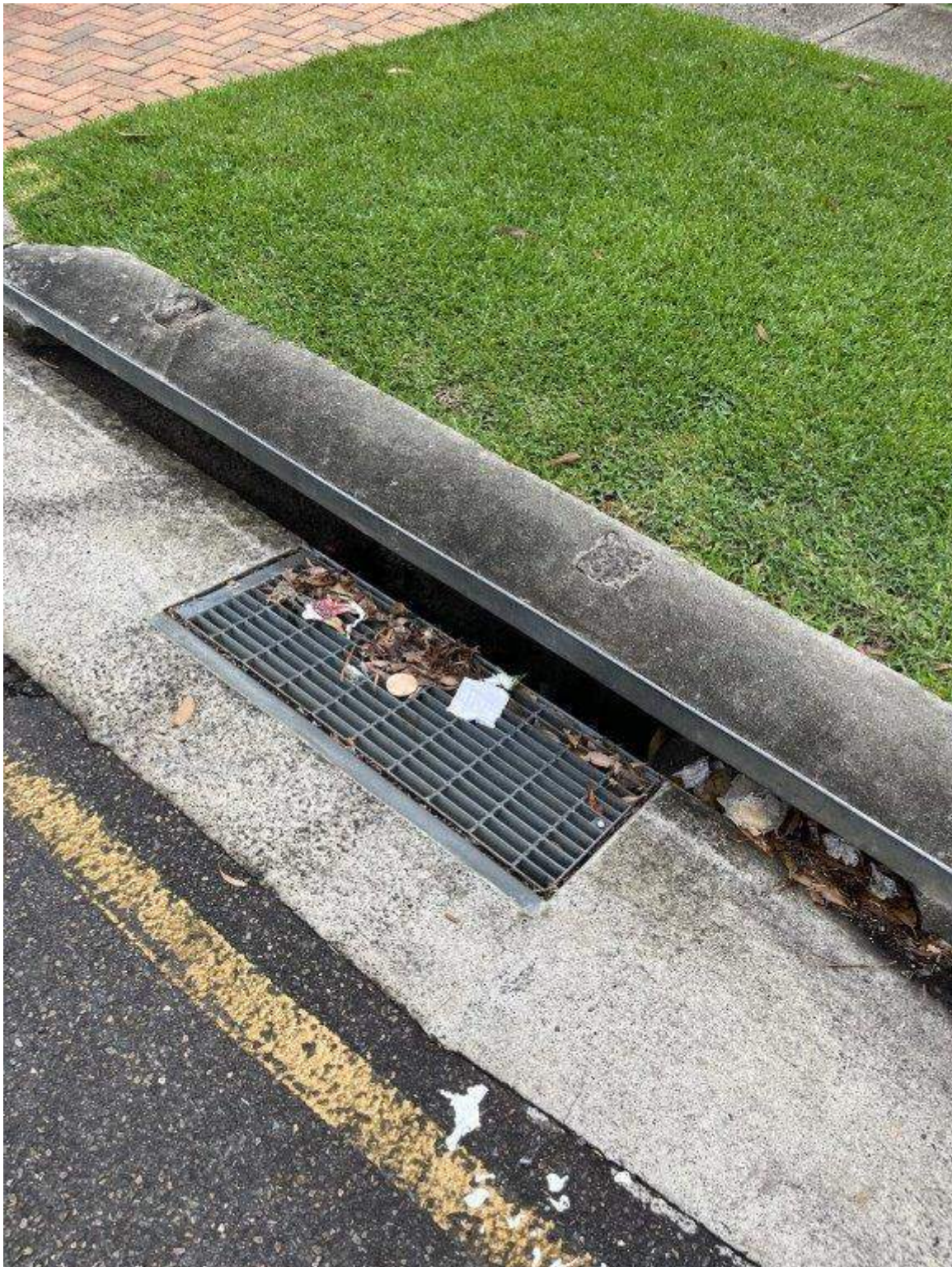
Photo 146 - Taren Point Road - Existing condition of steel grate
