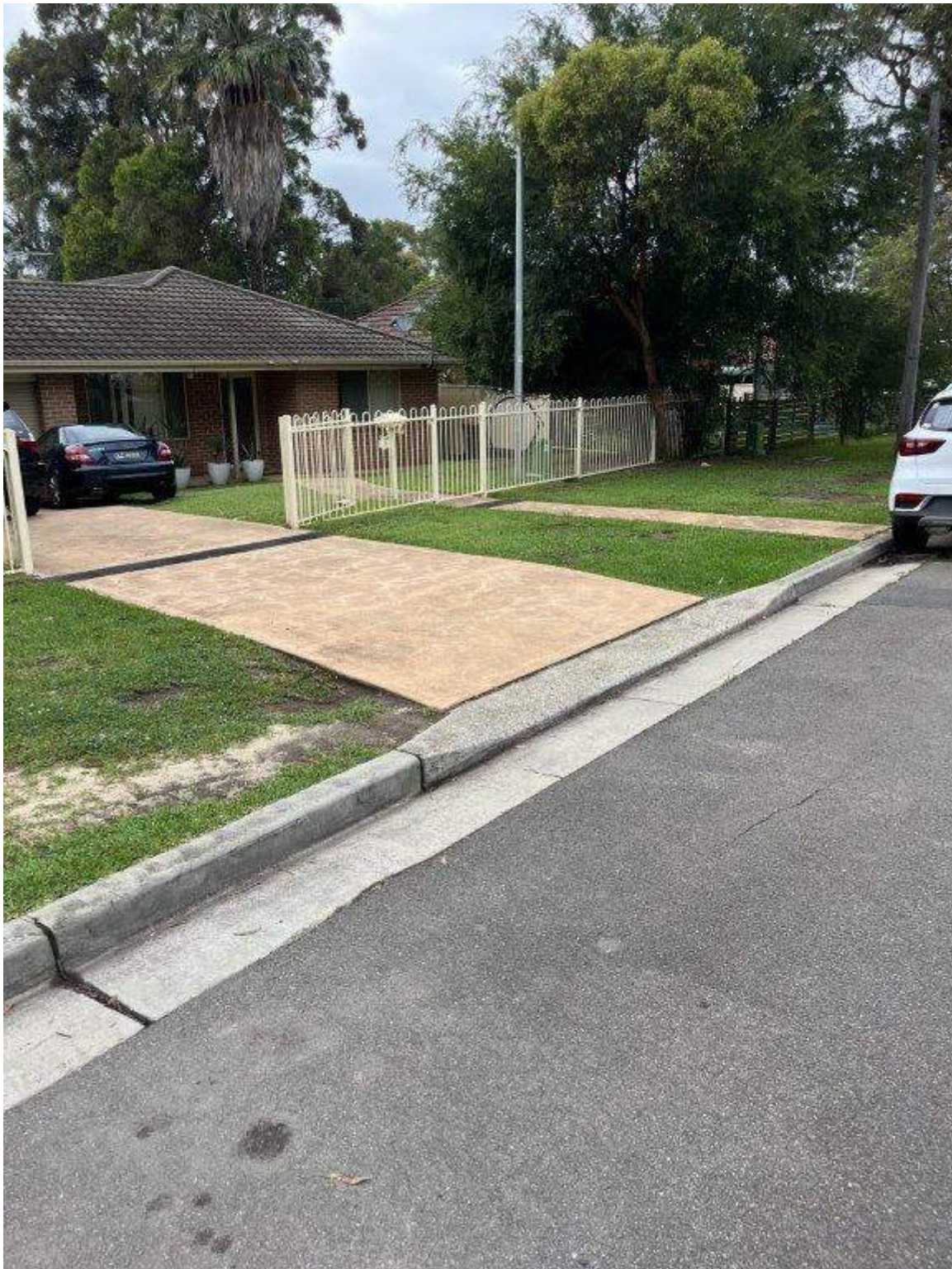
Photo 62 - Hinkler Avenue - Existing condition of pavement and vegetation
