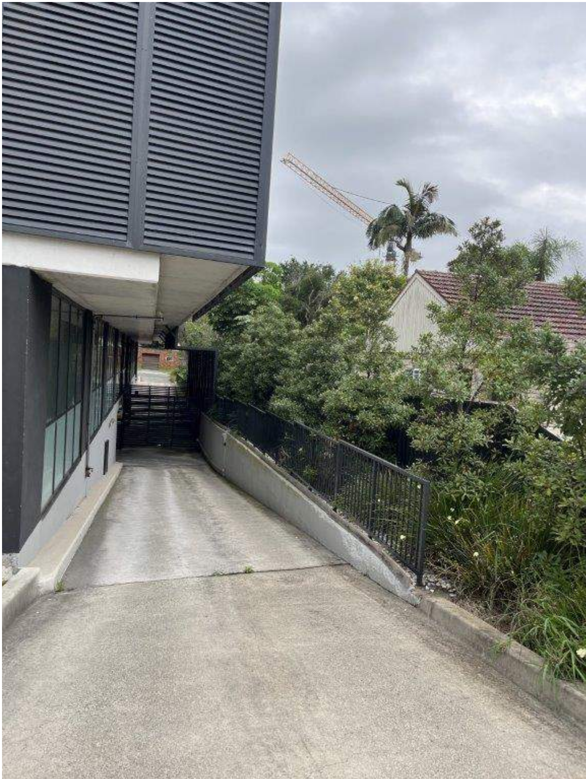
Photo 24 - Hinkler Avenue - Existing condition of pavement
