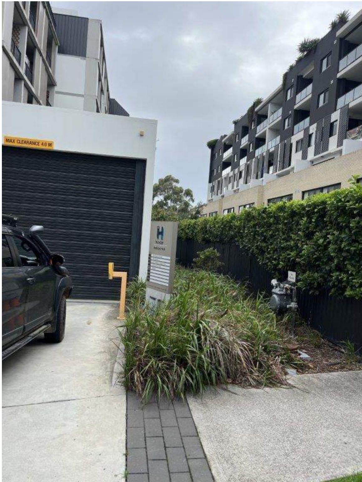
Photo 2 - Hinkler Avenue - Existing condition of pavement and external facade
