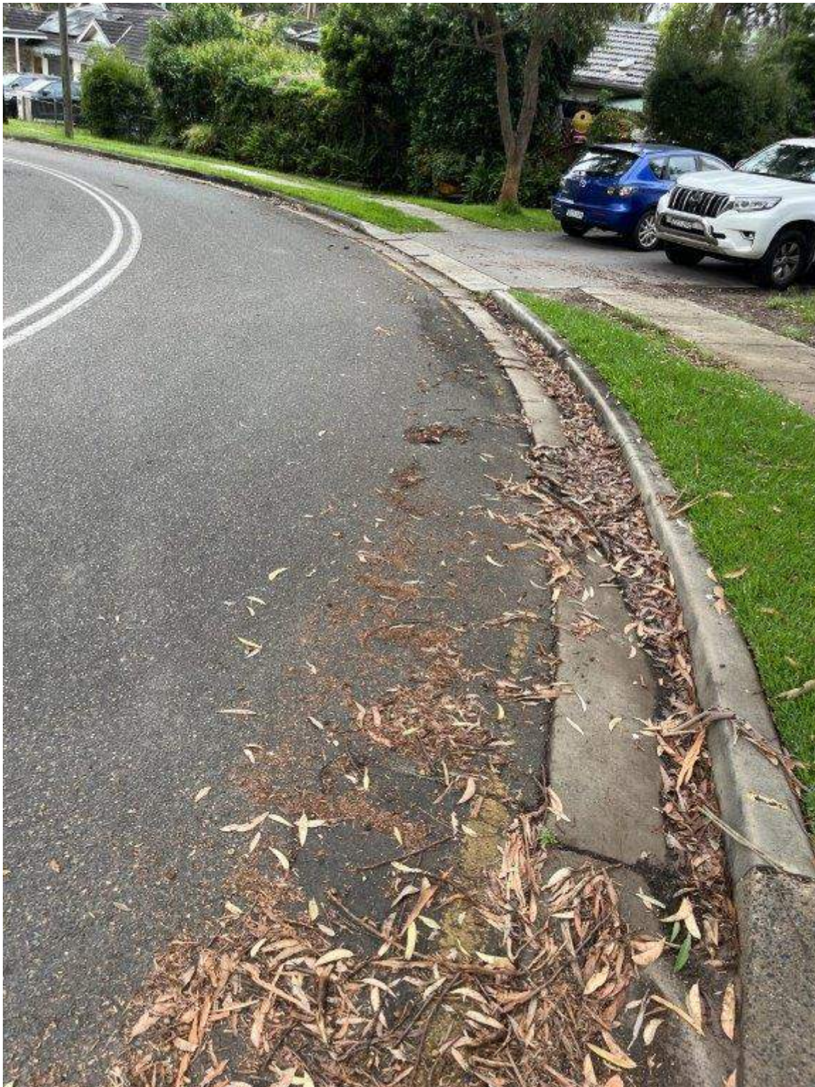
Photo 111 - Hinkler Avenue - Existing condition of pavement
