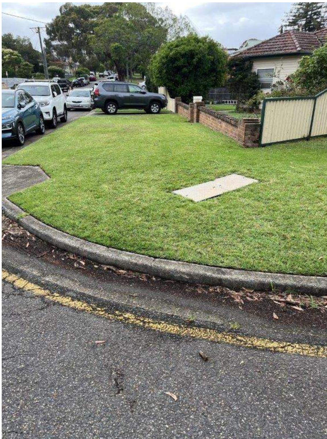
Photo 190 - Taren Point Road - Cracking of pavement
