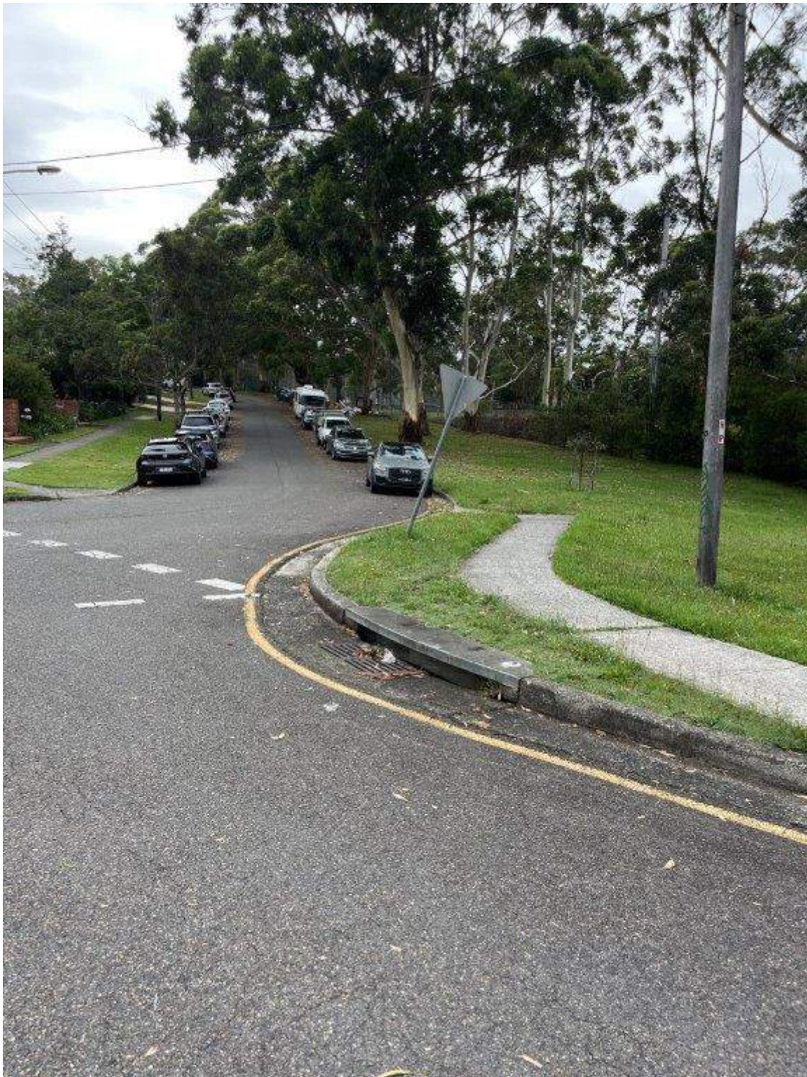
Photo 137 - Hinkler Avenue - Existing condition of pavement and vegetation
