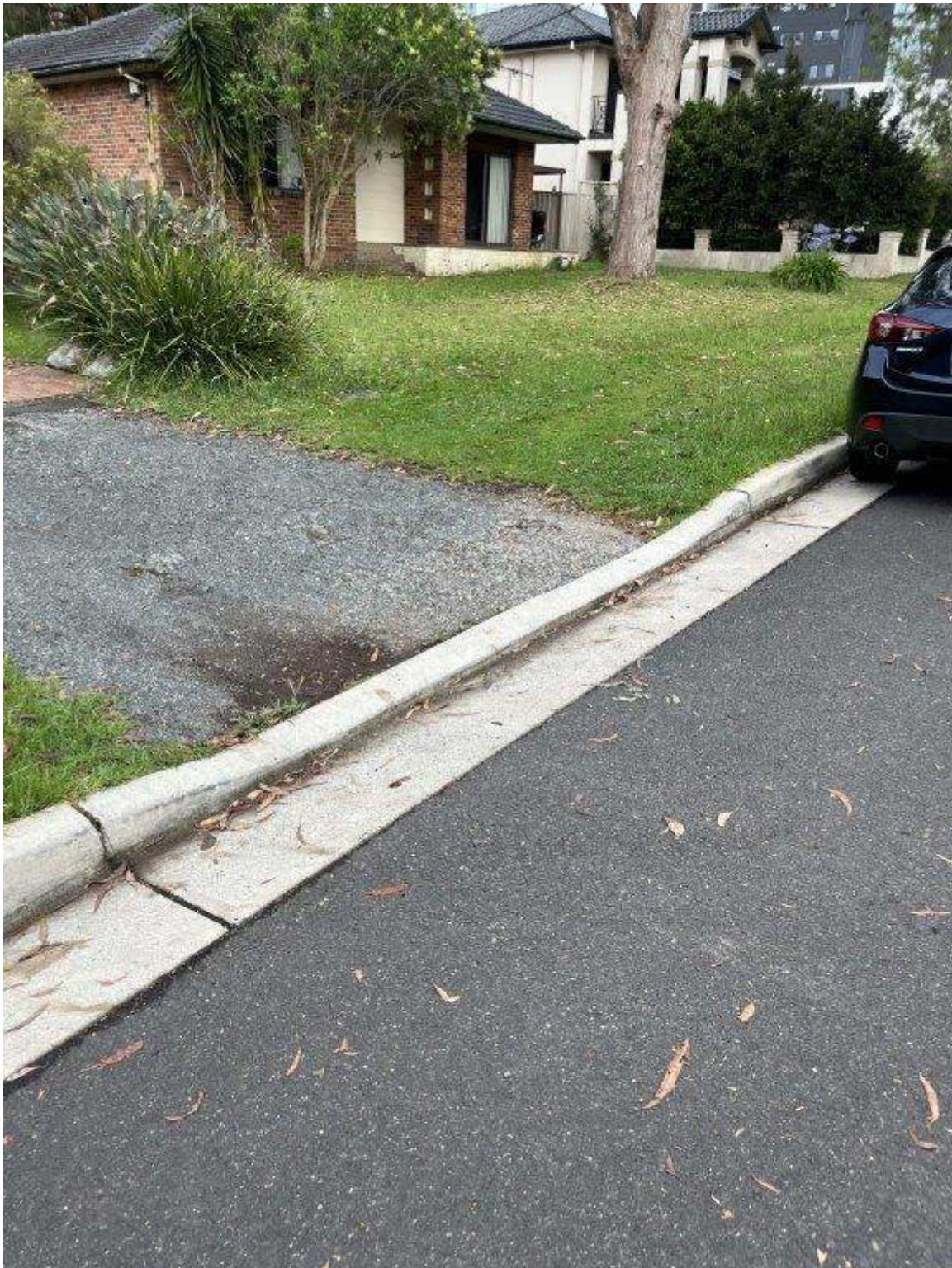
Photo 176 - Taren Point Road - Existing condition of pavement and vegetation
