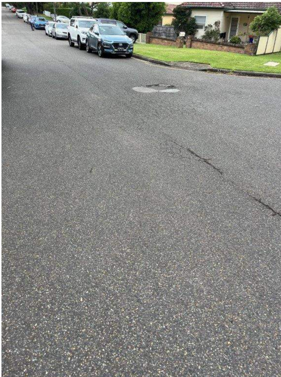
Photo 201 - Taren Point Road – Patching of pavement
