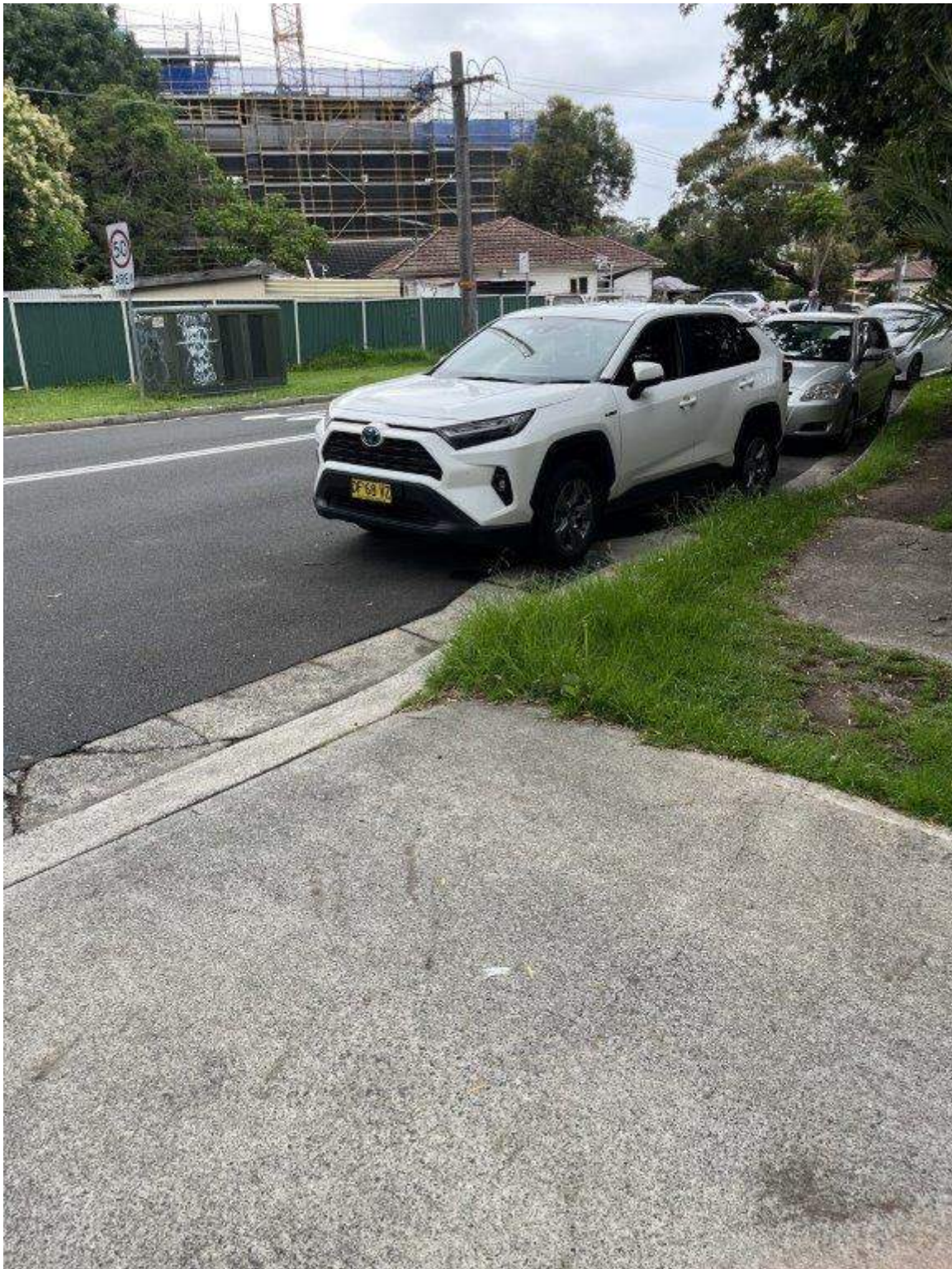
Photo 250 - Taren Point Road - Cracking of pavement
