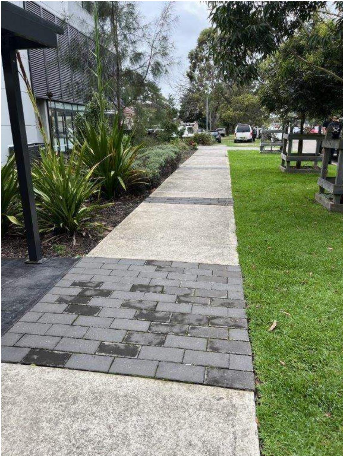
Photo 12 - Hinkler Avenue - Existing condition of pavement and vegetation
