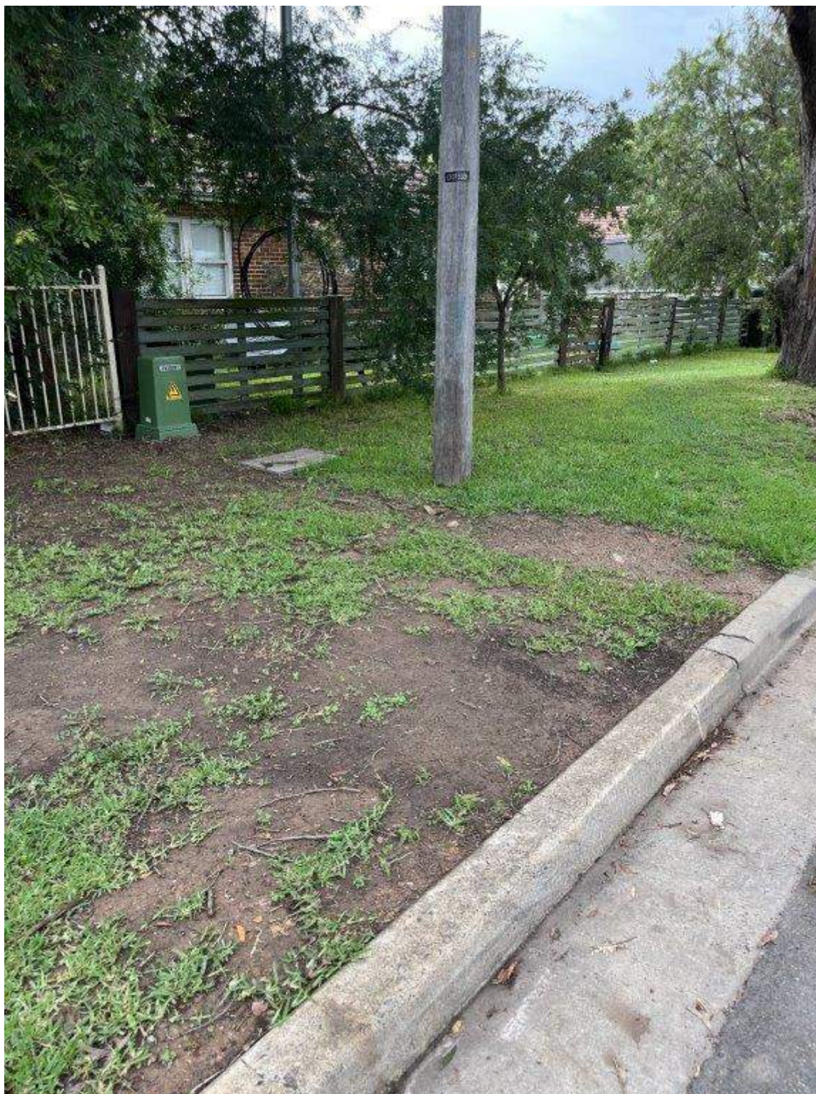
Photo 70 - Hinkler Avenue - Existing condition of pavement, post and vegetation
