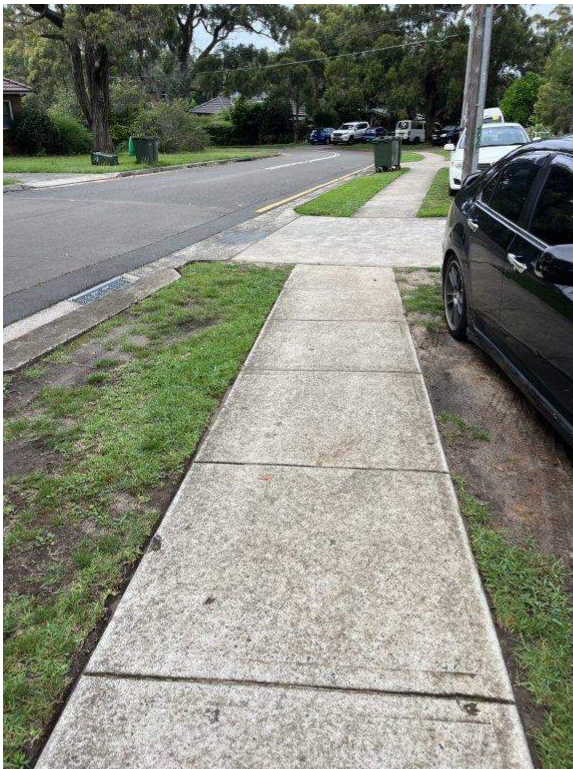
Photo 97 - Hinkler Avenue - Existing condition of pavement
