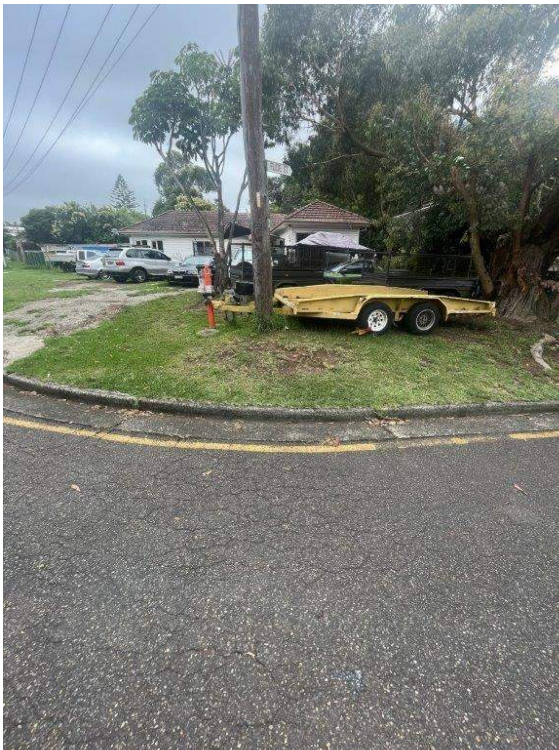
Photo 199 - Taren Point Road - Cracking of pavement
