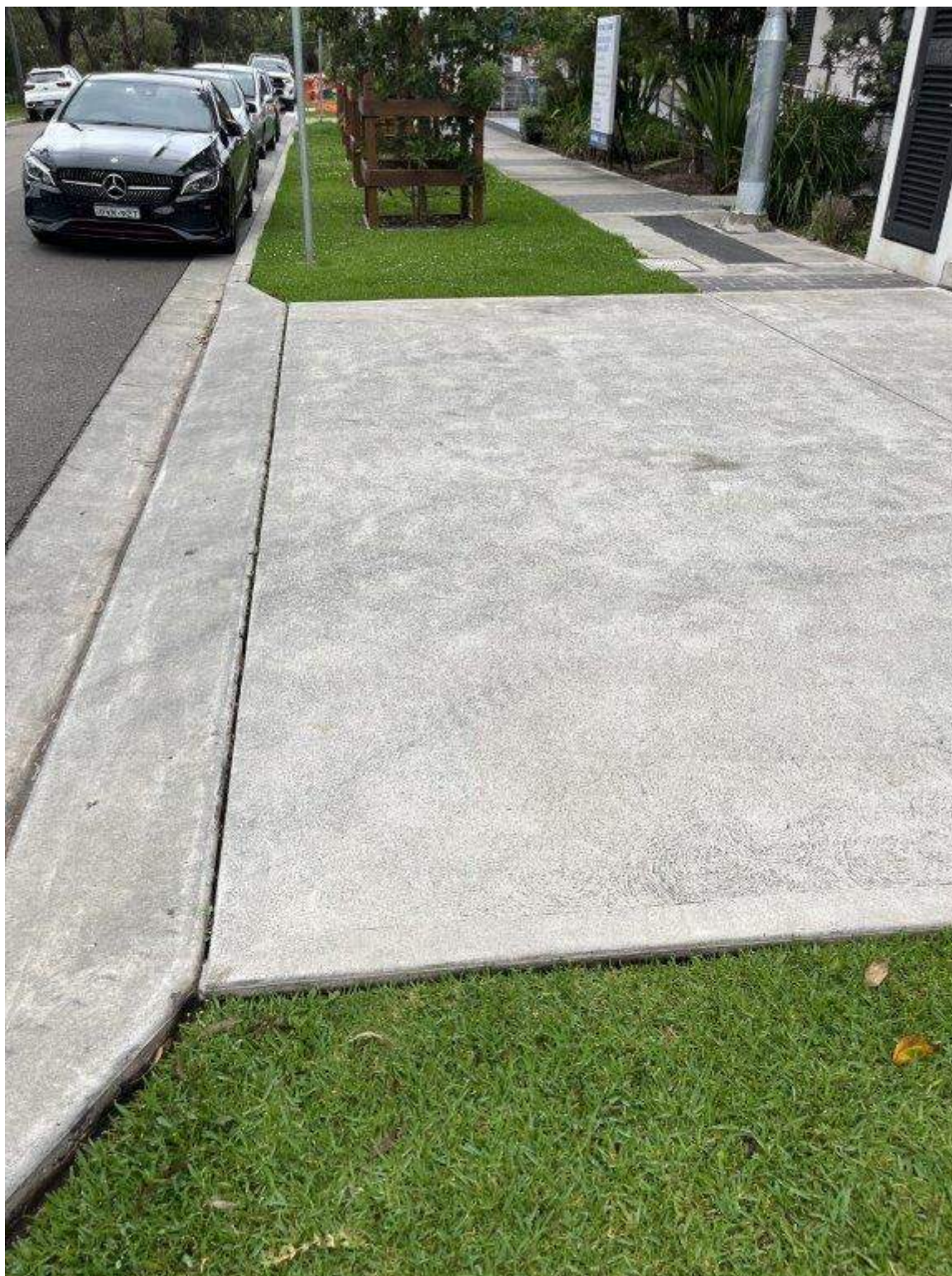
Photo 49 - Hinkler Avenue - Existing condition of pavement
