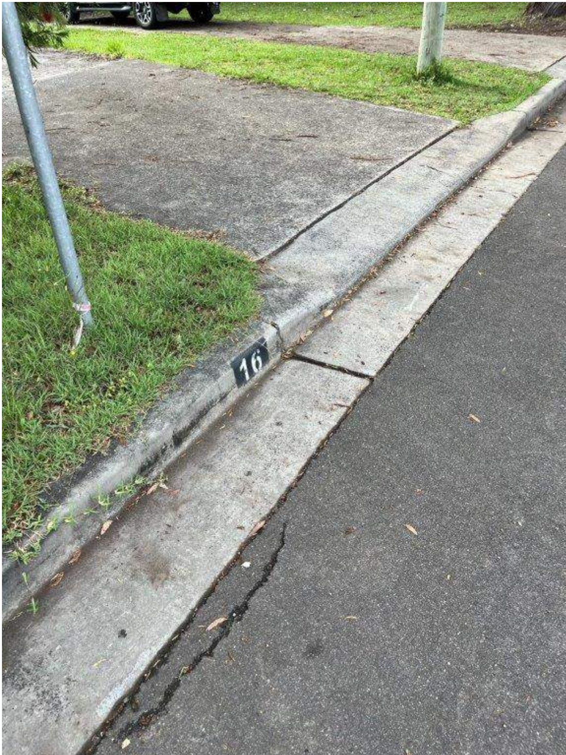
Photo 86 - Hinkler Avenue - Existing condition of pavement
