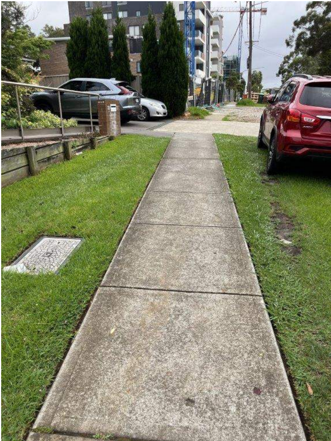
Photo 96 - Hinkler Avenue - Existing condition of pavement
