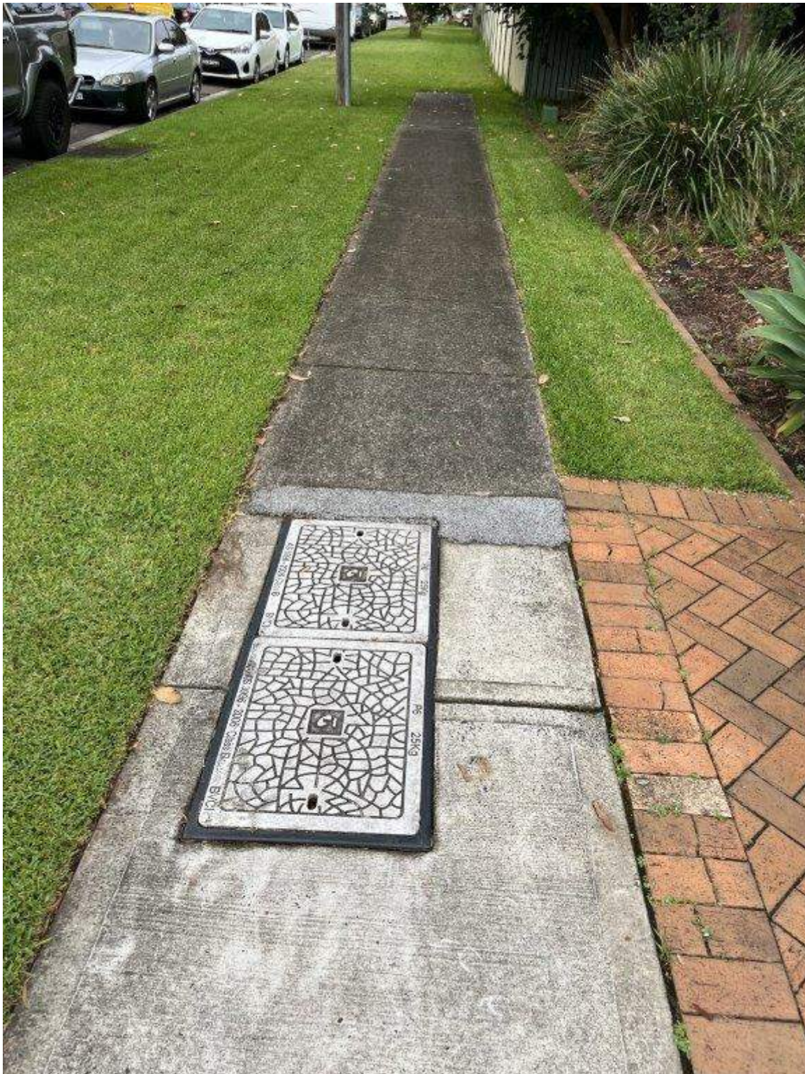
Photo 157 - Taren Point Road - Existing condition of pavement and service pit
