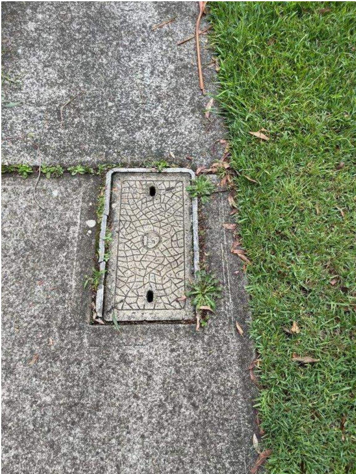
Photo 128 - Hinkler Avenue - Existing condition of service pit
