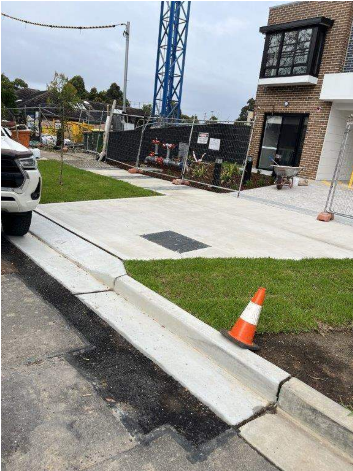
Photo 69 - Hinkler Avenue - Existing condition of pavement
