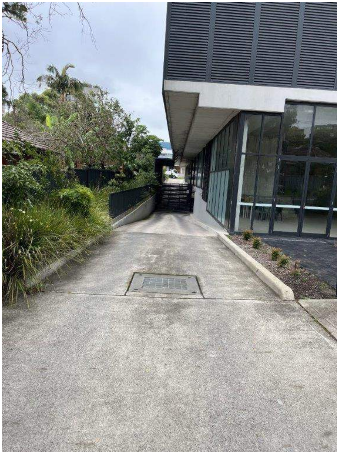
Photo 243 - Taren Point Road - Existing condition of pavement and steel grate
