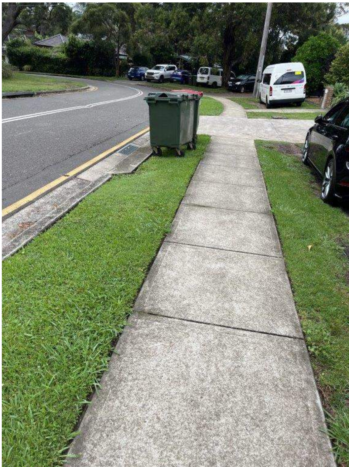
Photo 103 - Hinkler Avenue - Existing condition of pavement and vegetation
