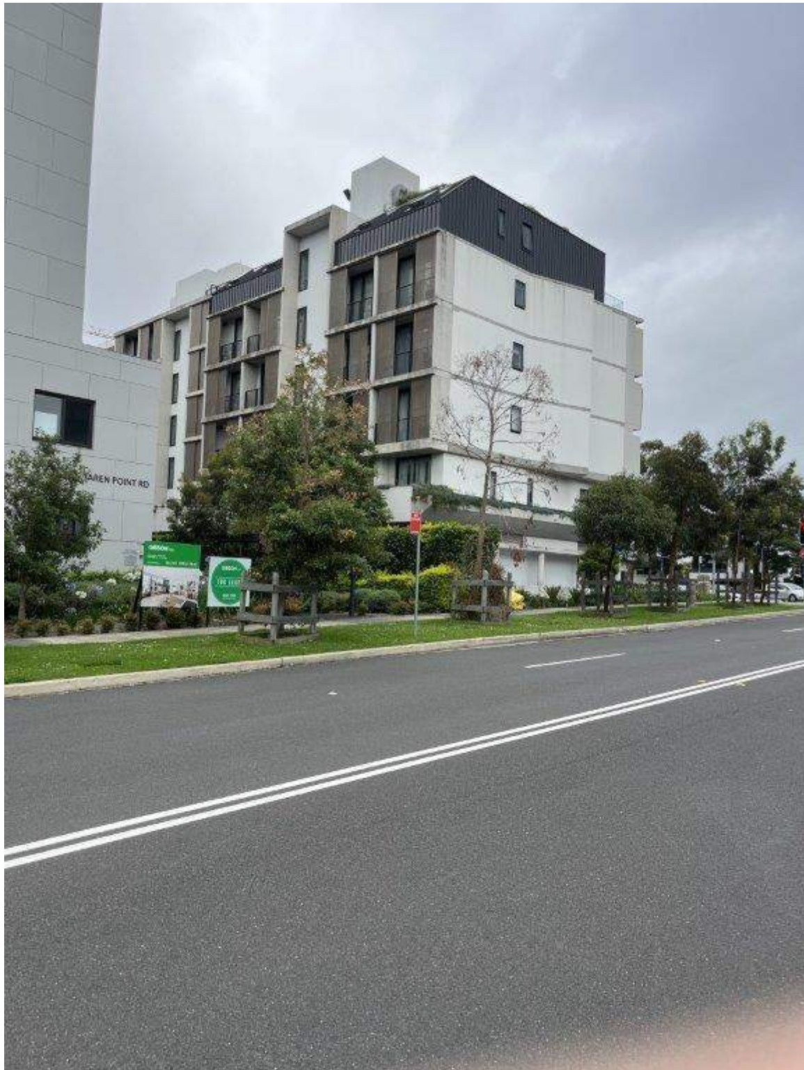
Photo 232 - Taren Point Road - Existing condition of external façade and pavement
