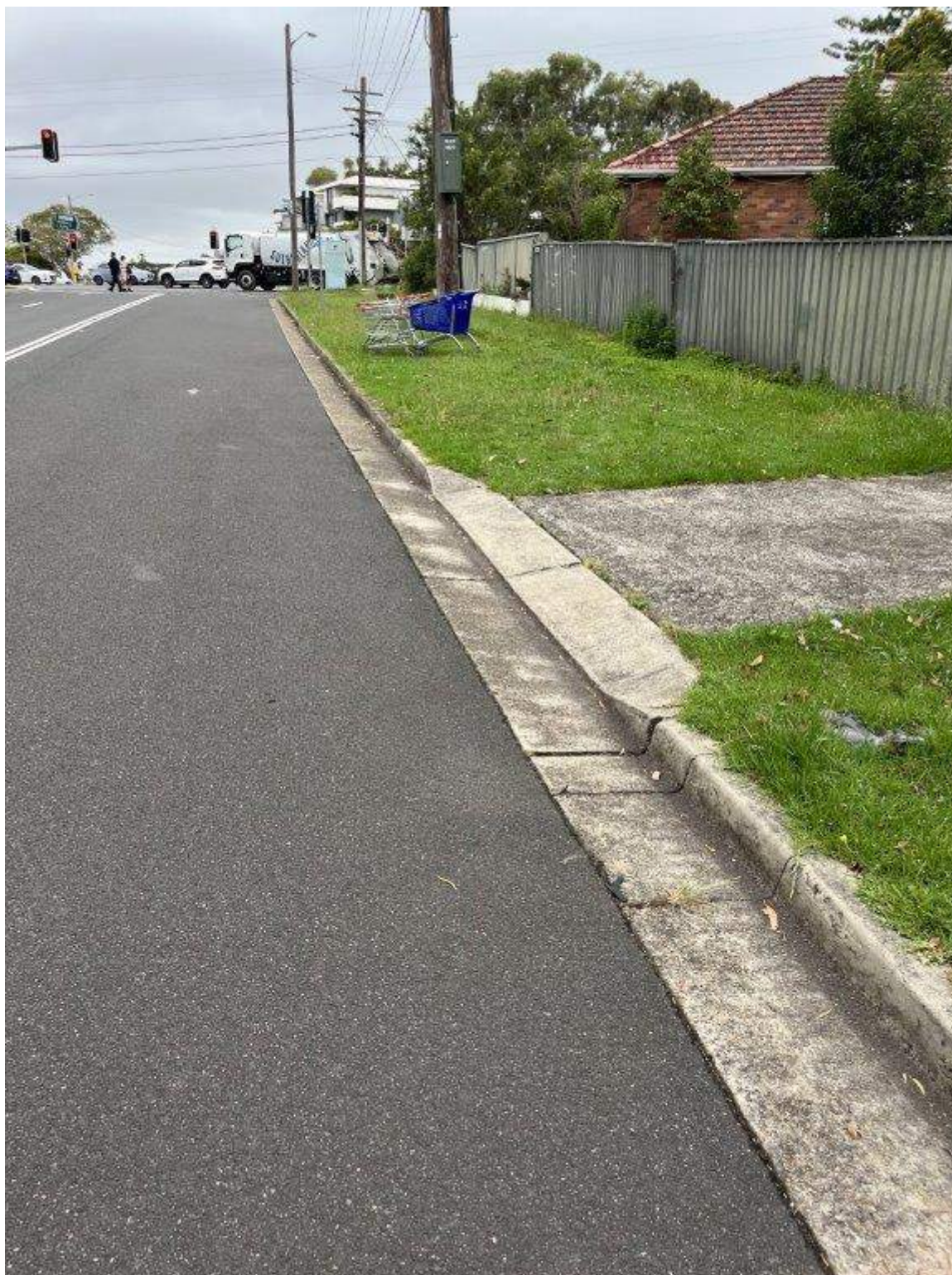
Photo 226 - Taren Point Road - Existing condition of pavement and vegetation
