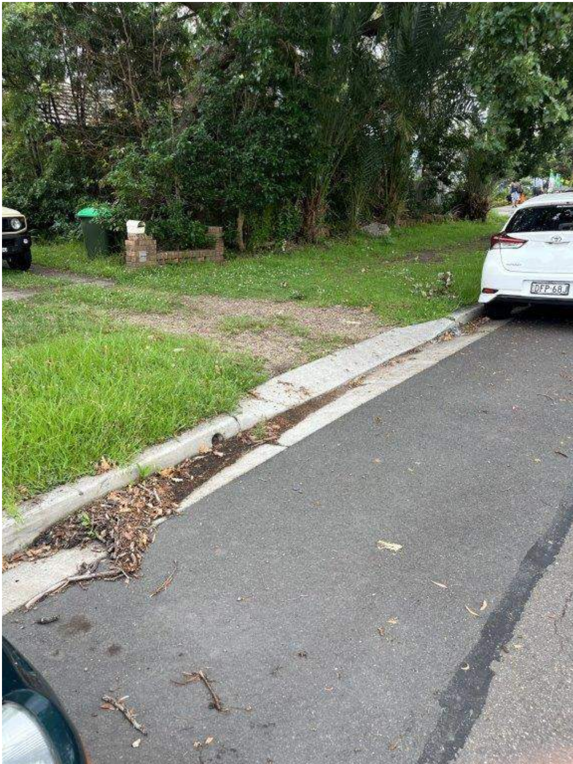
Photo 219 - Taren Point Road - Existing condition of pavement and vegetation
