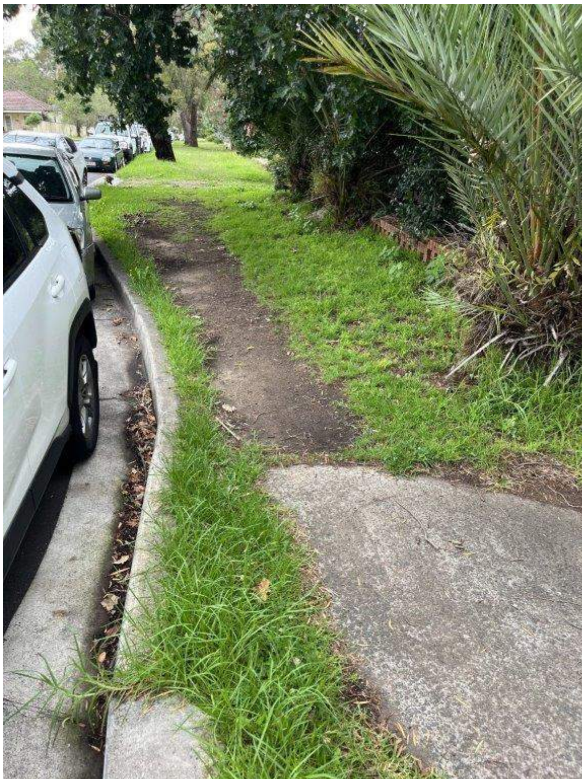
Photo 252 - Taren Point Road - Existing condition of pavement and vegetation
