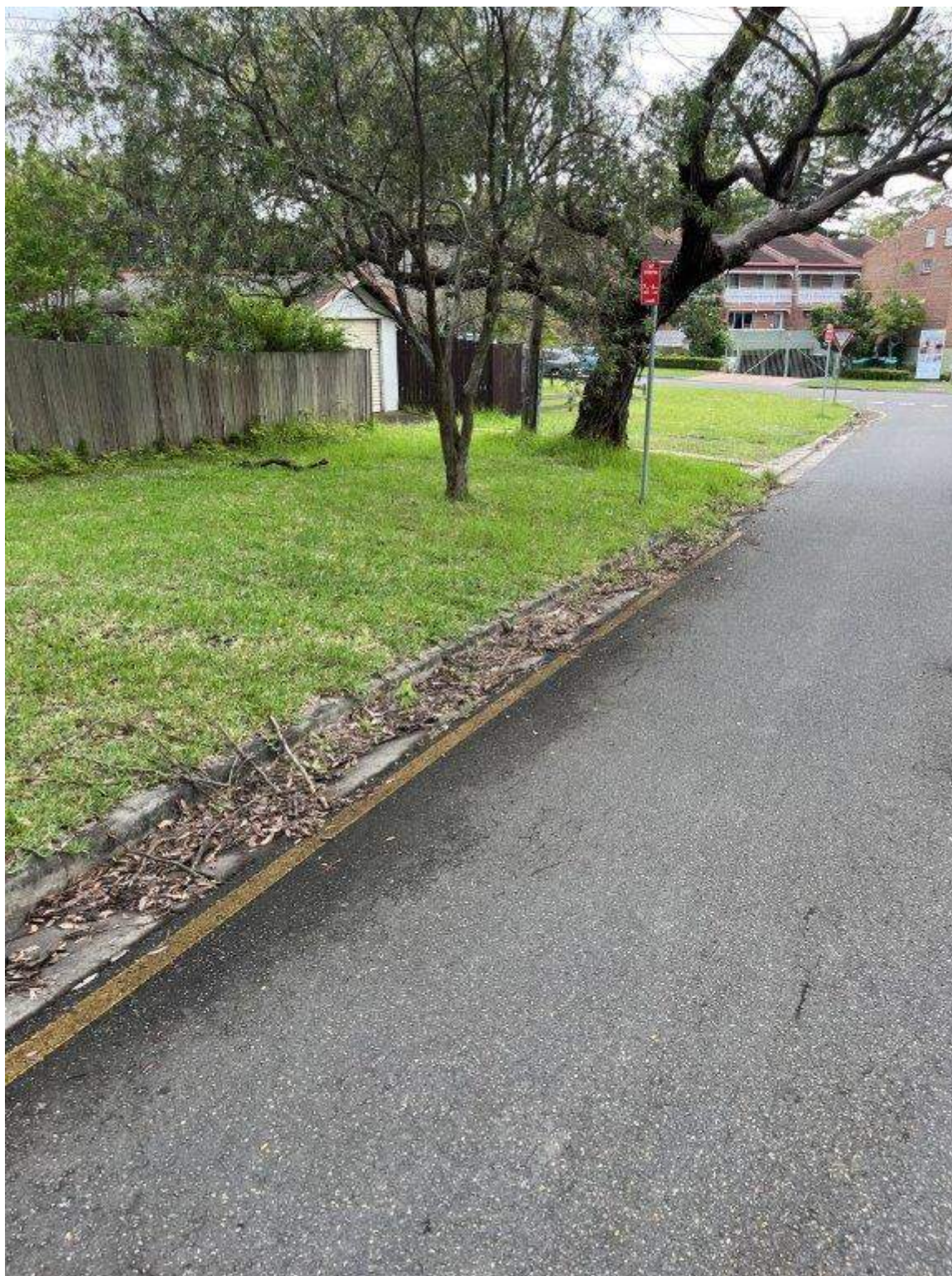
Photo 123 - Hinkler Avenue - Existing condition of pavement and vegetation
