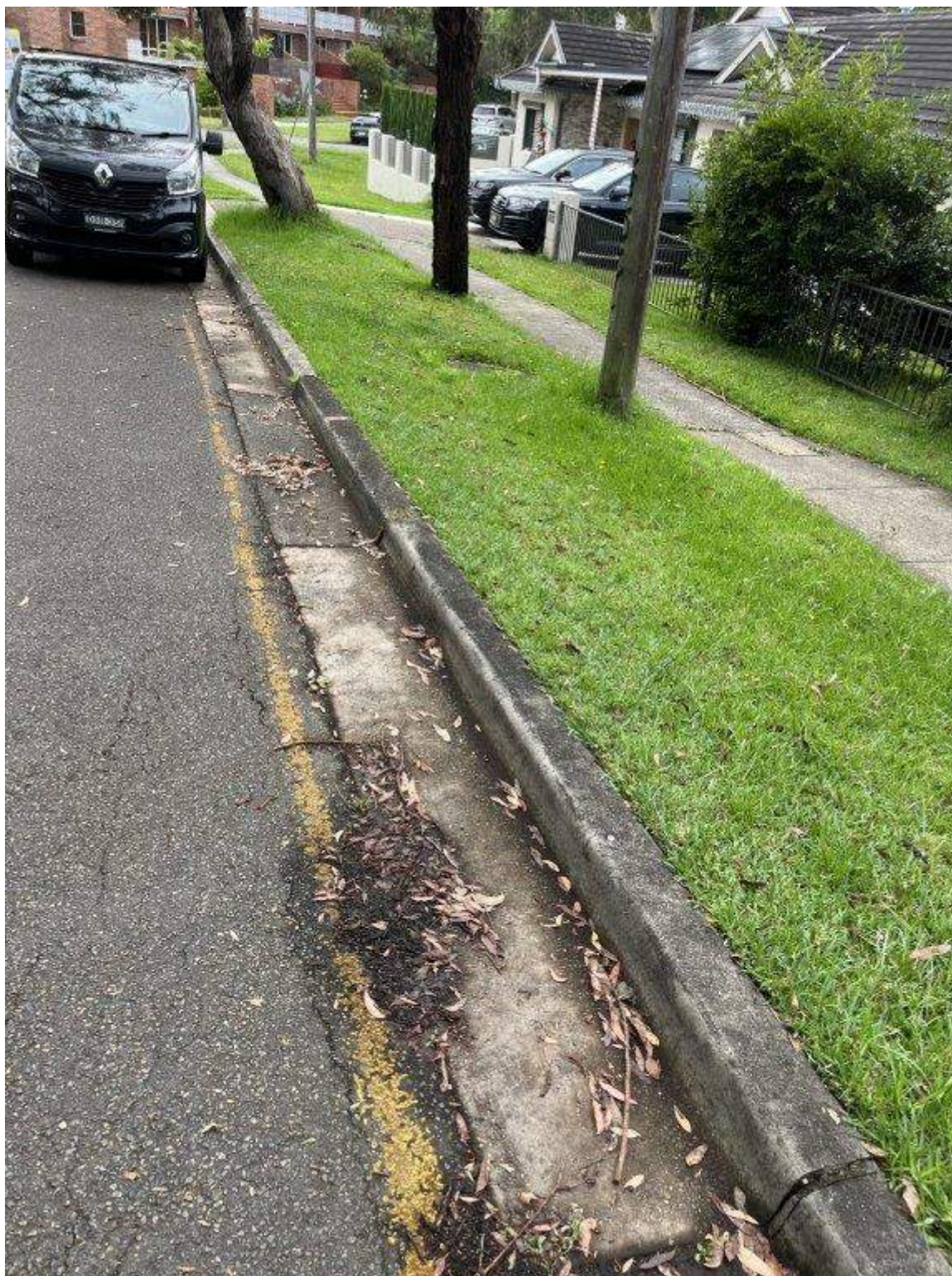
Photo 125 - Hinkler Avenue - Existing condition of pavement and vegetation
