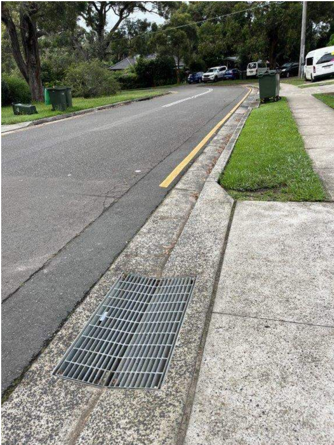
Photo 98 - Hinkler Avenue - Existing condition of steel grate and pavement
