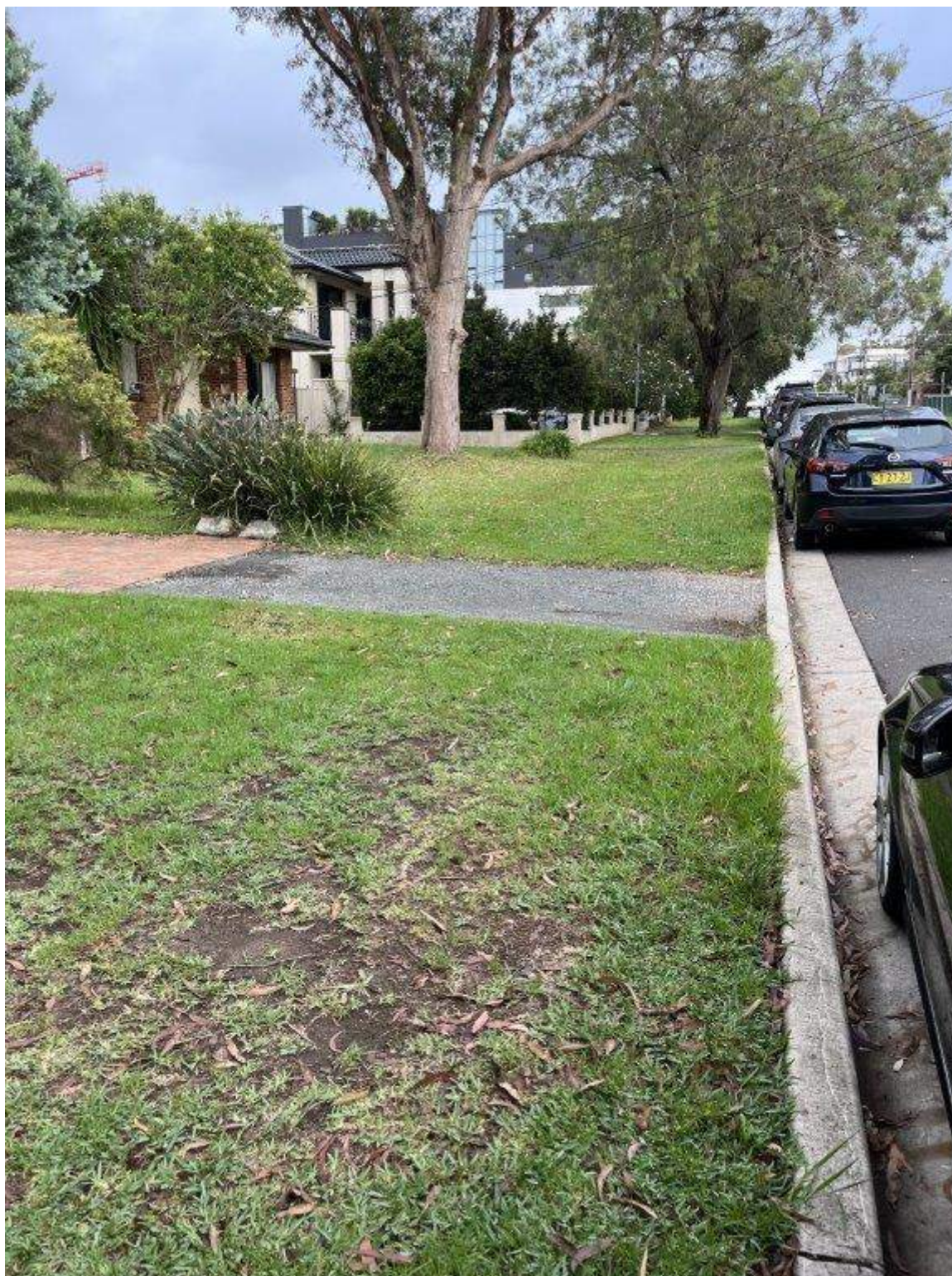
Photo 175 - Taren Point Road - Existing condition of pavement and vegetation
