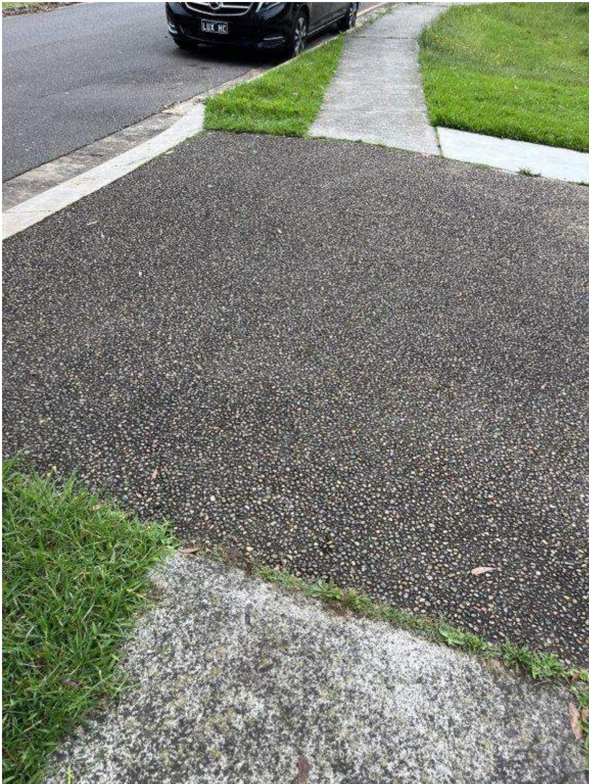
Photo 130 - Hinkler Avenue - Existing condition of pavement
