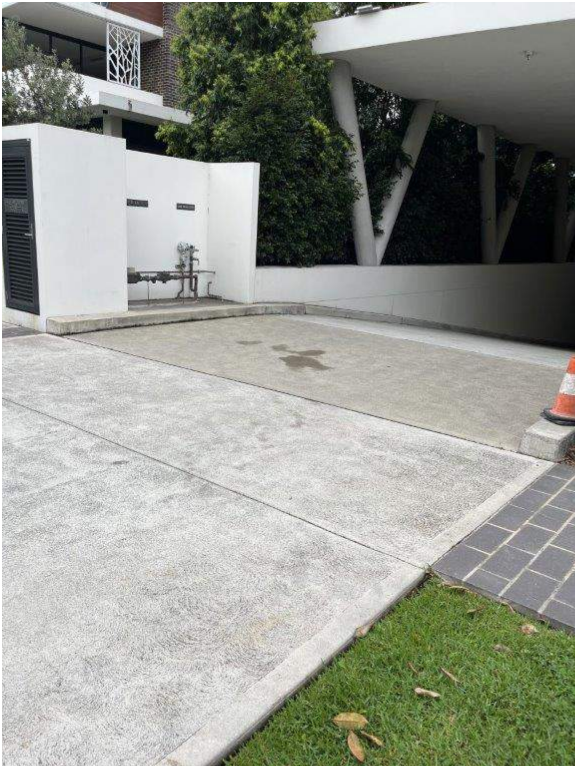
Photo 48 - Hinkler Avenue - Existing condition of pavement
