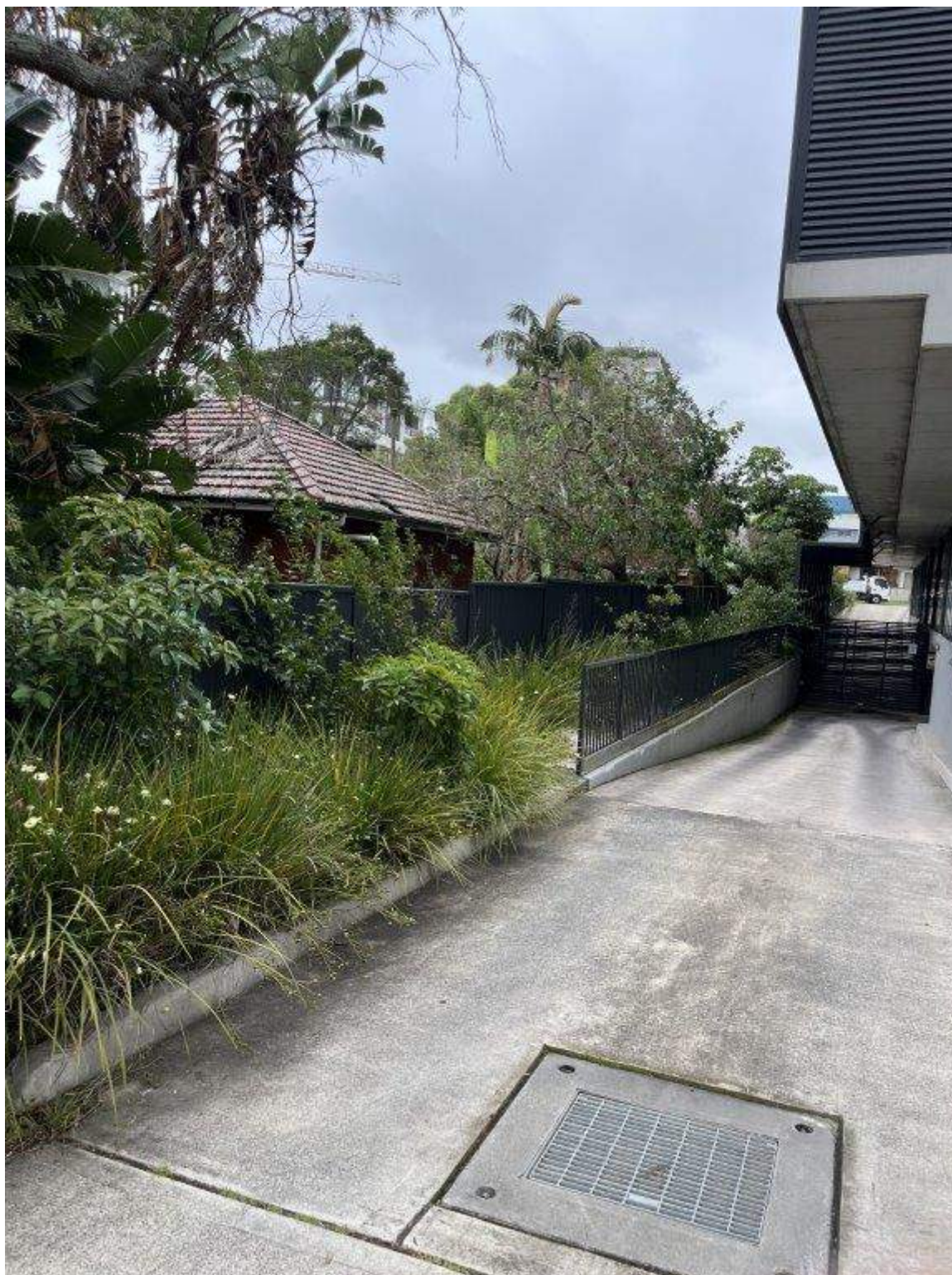
Photo 246 - Taren Point Road - Existing condition of pavement and steel grate
