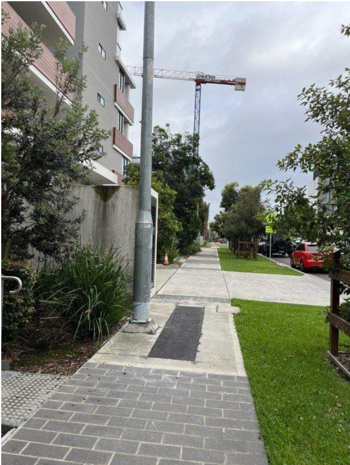
Photo 56 - Hinkler Avenue - Existing condition of pavement and post
