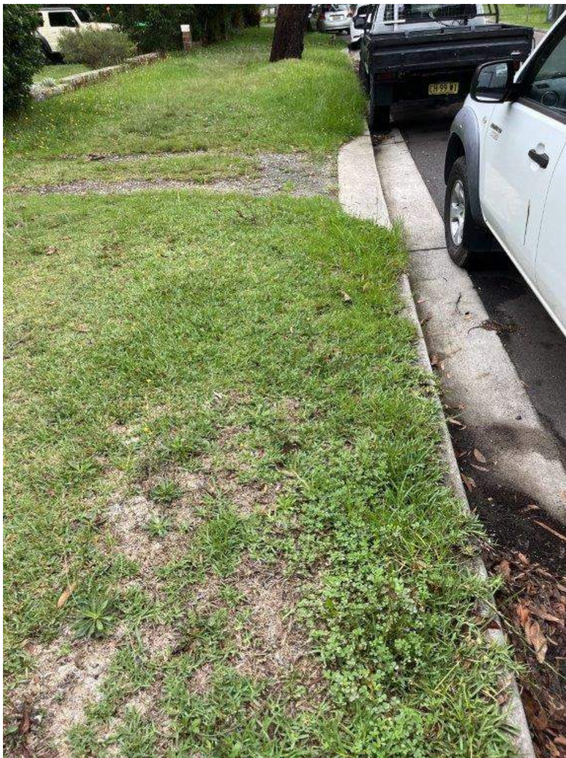
Photo 211 - Taren Point Road - Existing condition of pavement and vegetation
