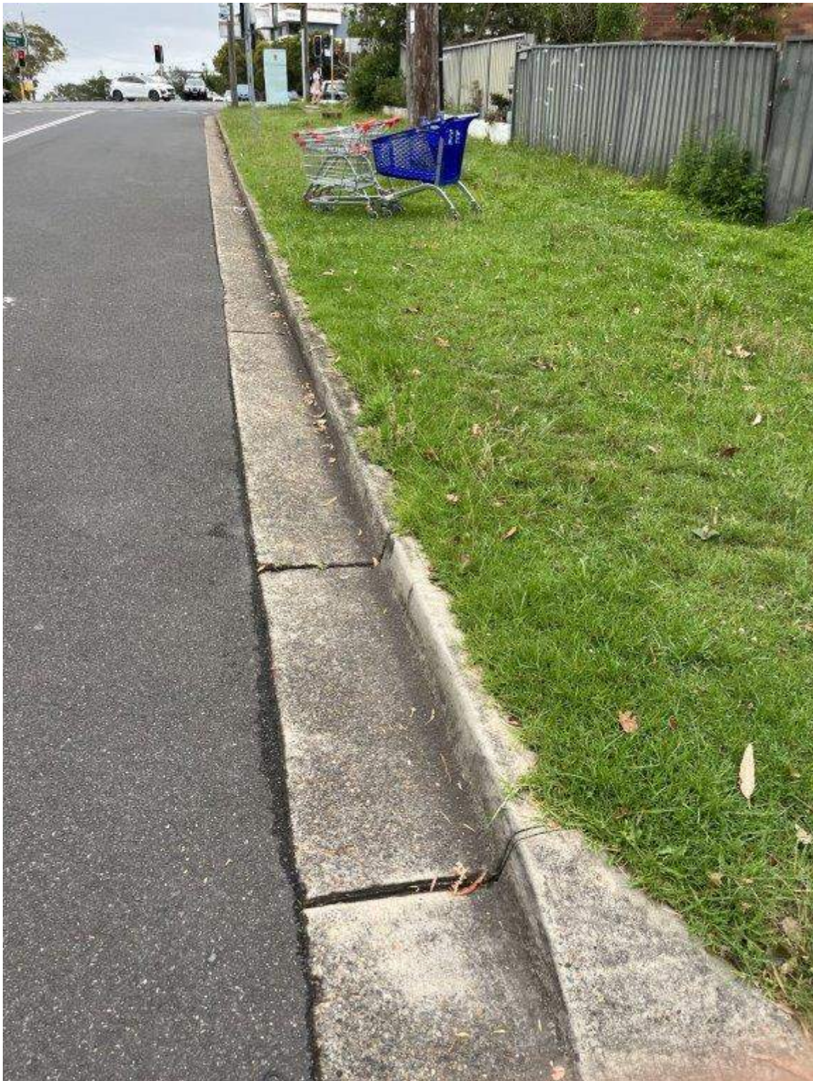
Photo 229 - Taren Point Road - Existing condition of pavement and vegetation
