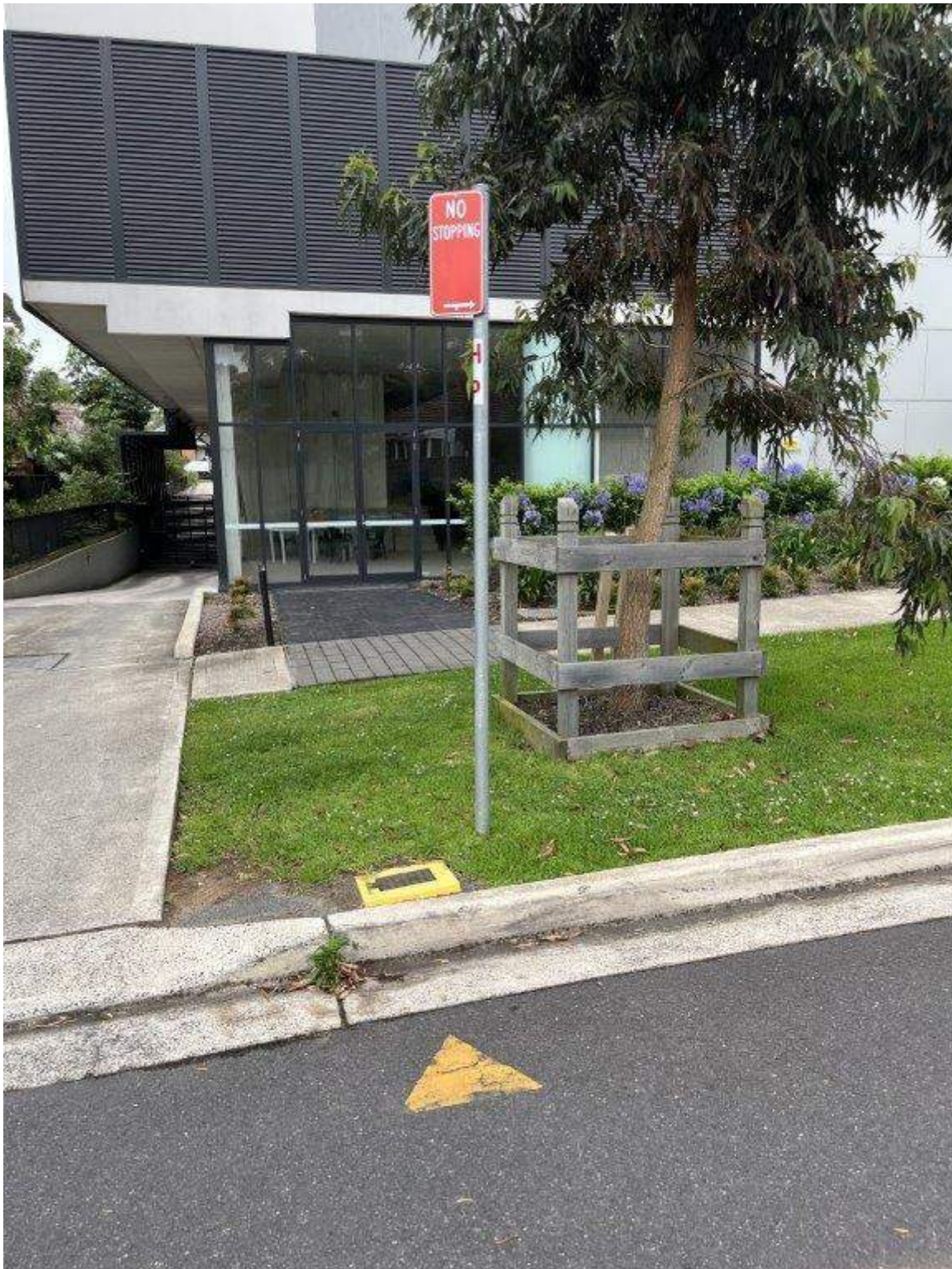
Photo 237 - Taren Point Road - Existing condition of pavement and vegetation
