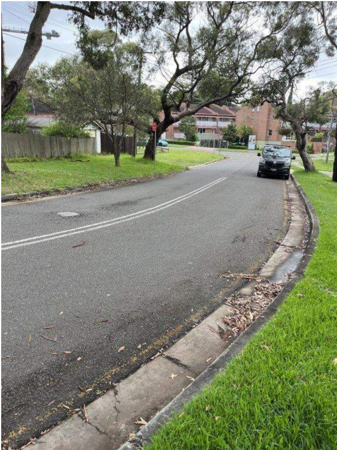
Photo 120 - Hinkler Avenue - Existing condition of pavement
