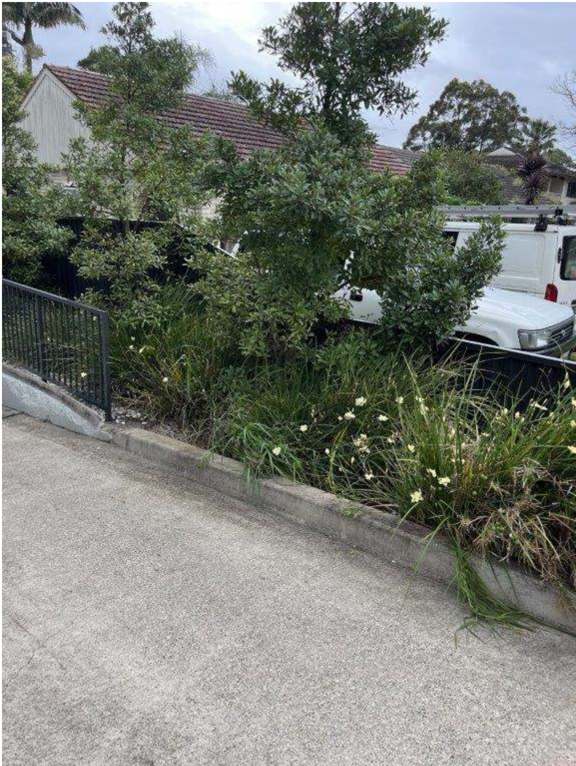
Photo 26 - Hinkler Avenue - Existing condition of pavement and vegetation
