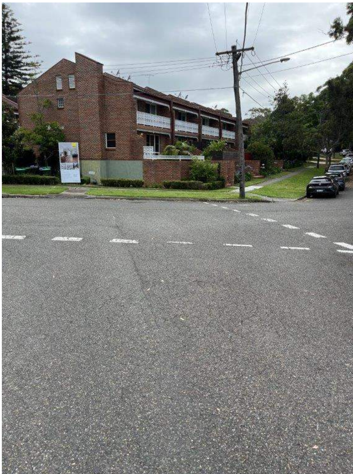
Photo 138 - Hinkler Avenue - Existing condition of pavement and vegetation
