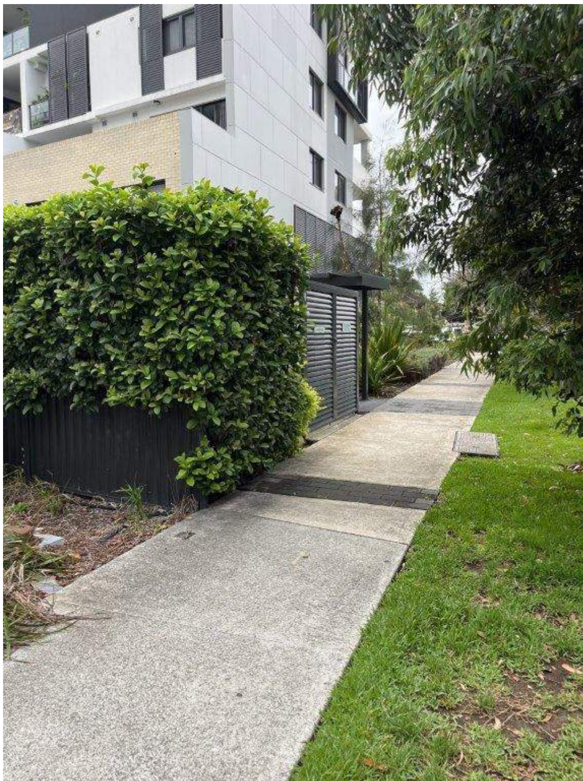
Photo 5 - Hinkler Avenue - Existing condition of pavement and vegetation
