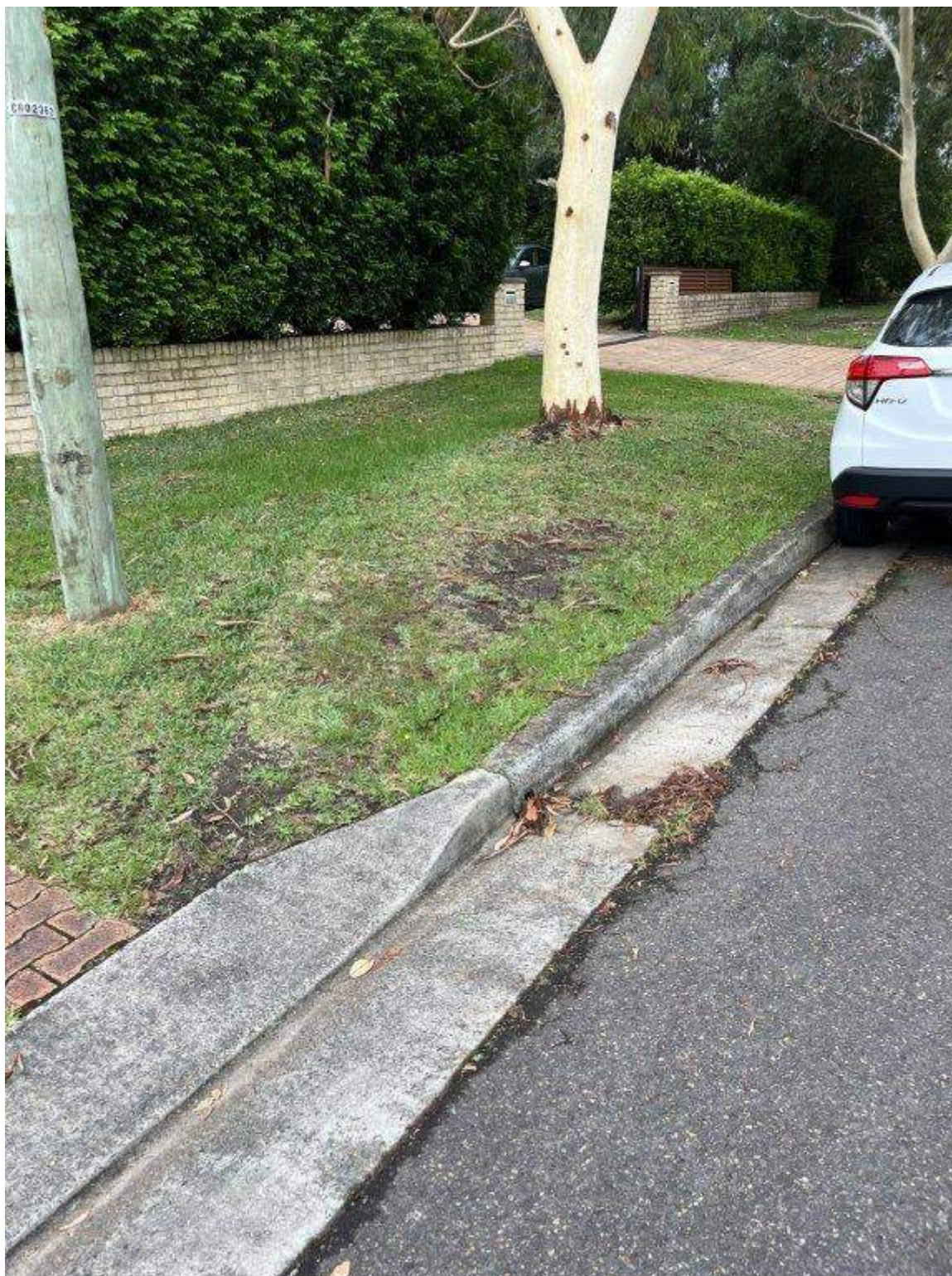
Photo 162 - Taren Point Road - Existing condition of pavement and vegetation
