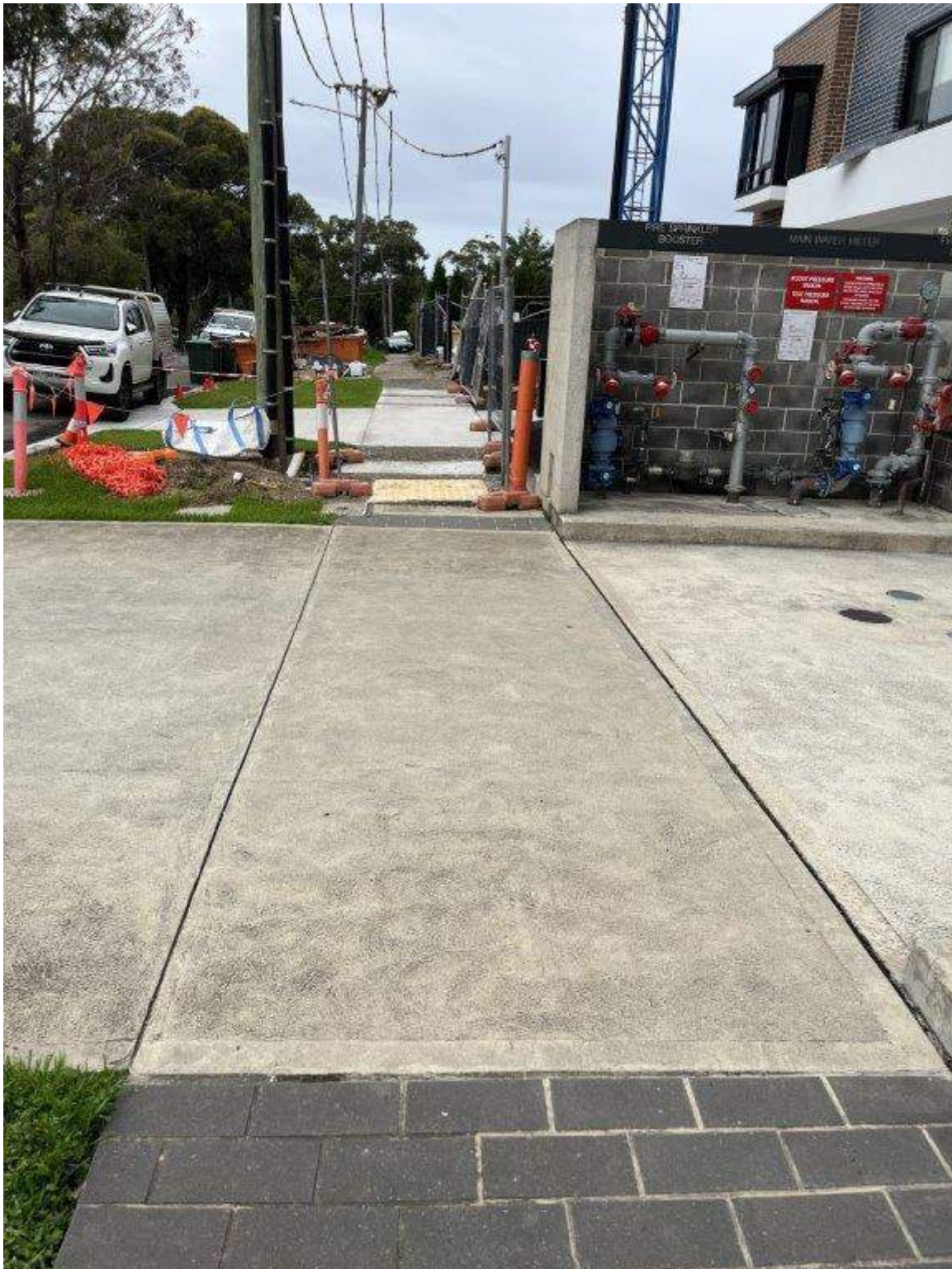
Photo 58 - Hinkler Avenue - Existing condition of pavement
