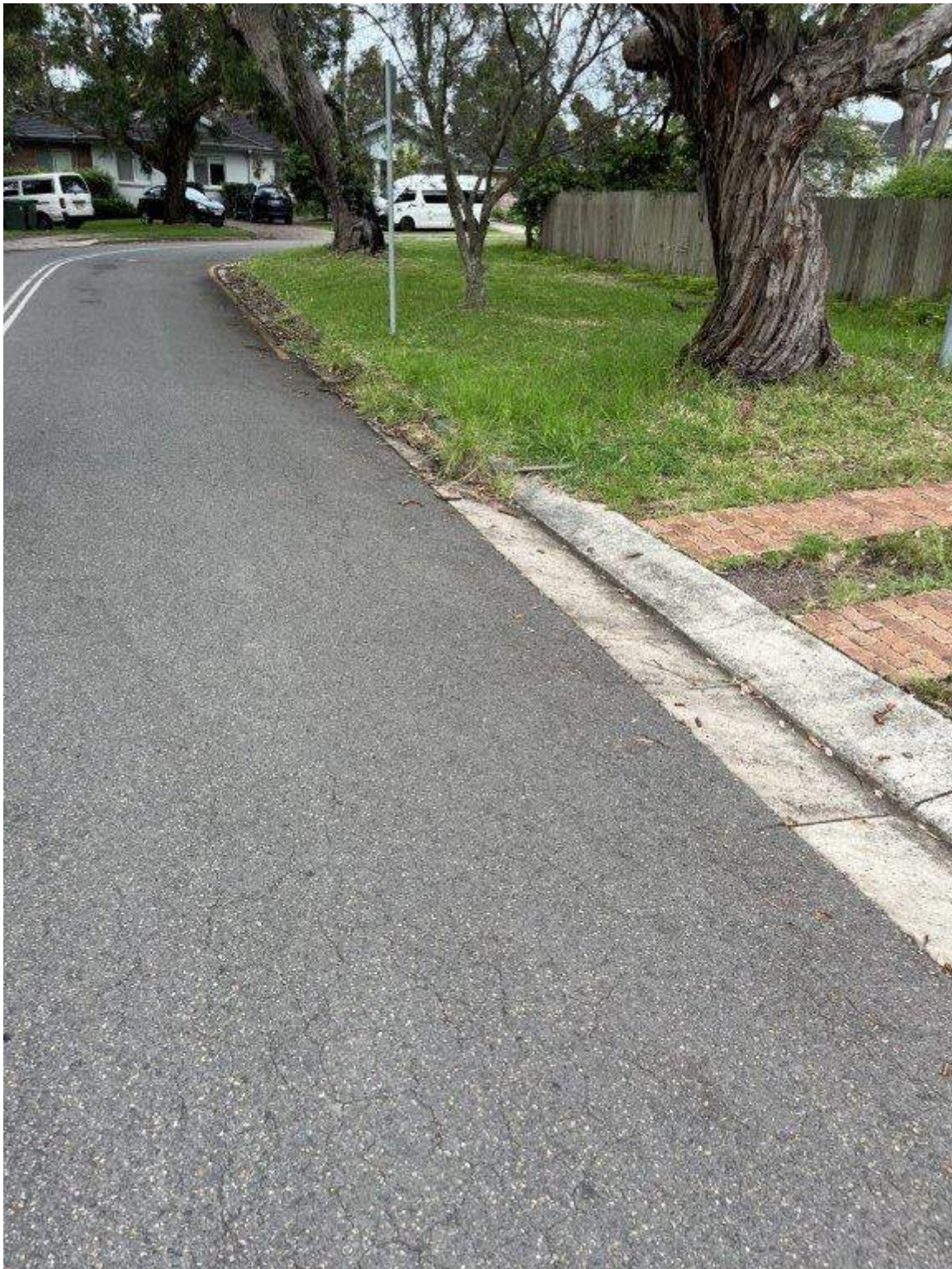
Photo 132 - Hinkler Avenue - Existing condition of pavement and vegetation
