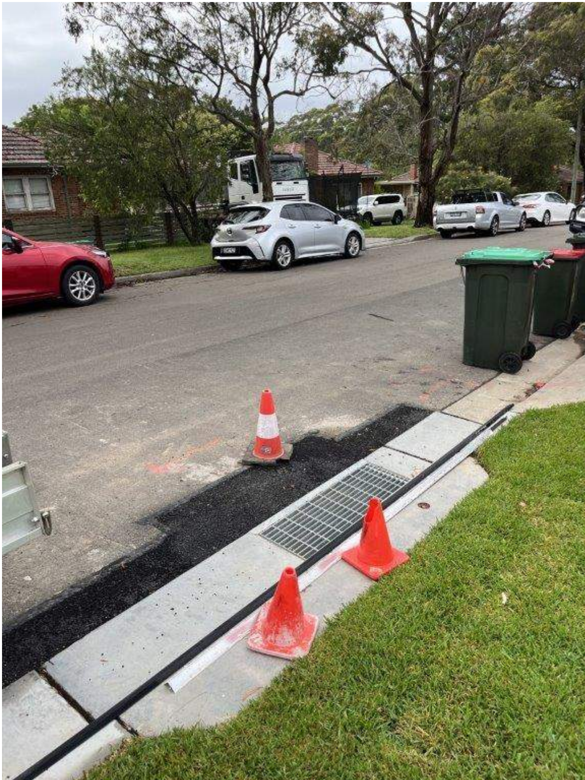
Photo 72 - Hinkler Avenue – Patching of pavement
