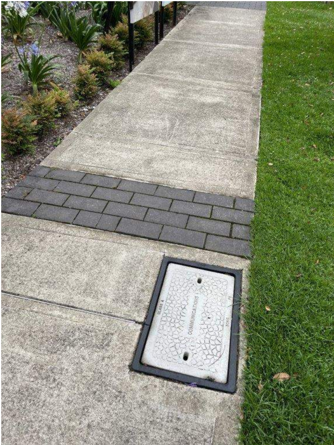
Photo 256 - Taren Point Road - Existing condition of pavement and service pit
