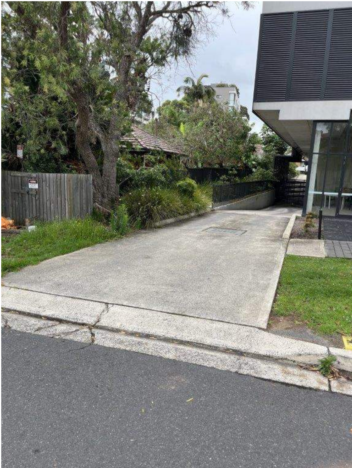
Photo 238 - Taren Point Road - Cracking of pavement
