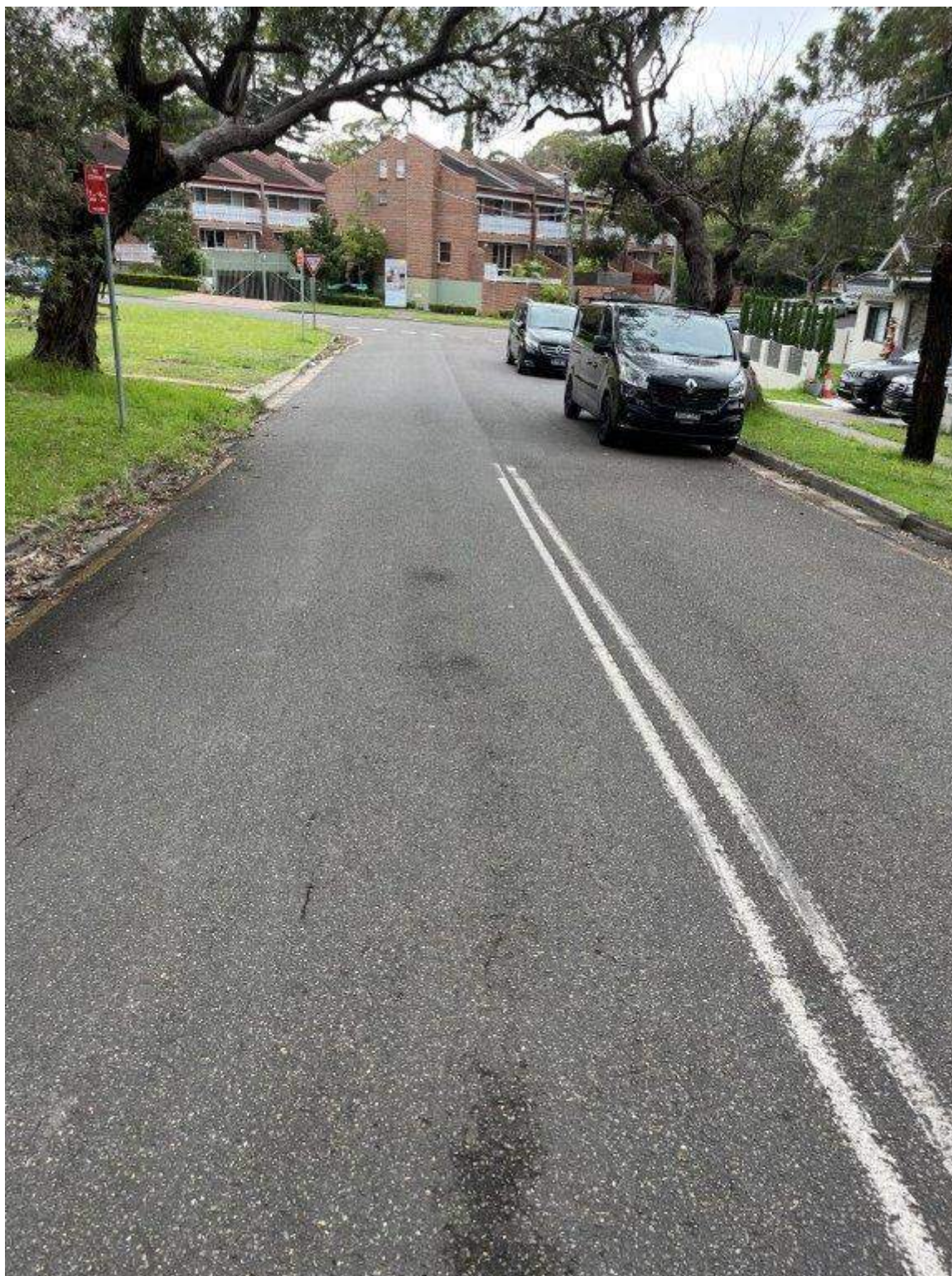
Photo 124 - Hinkler Avenue - Existing condition of pavement
