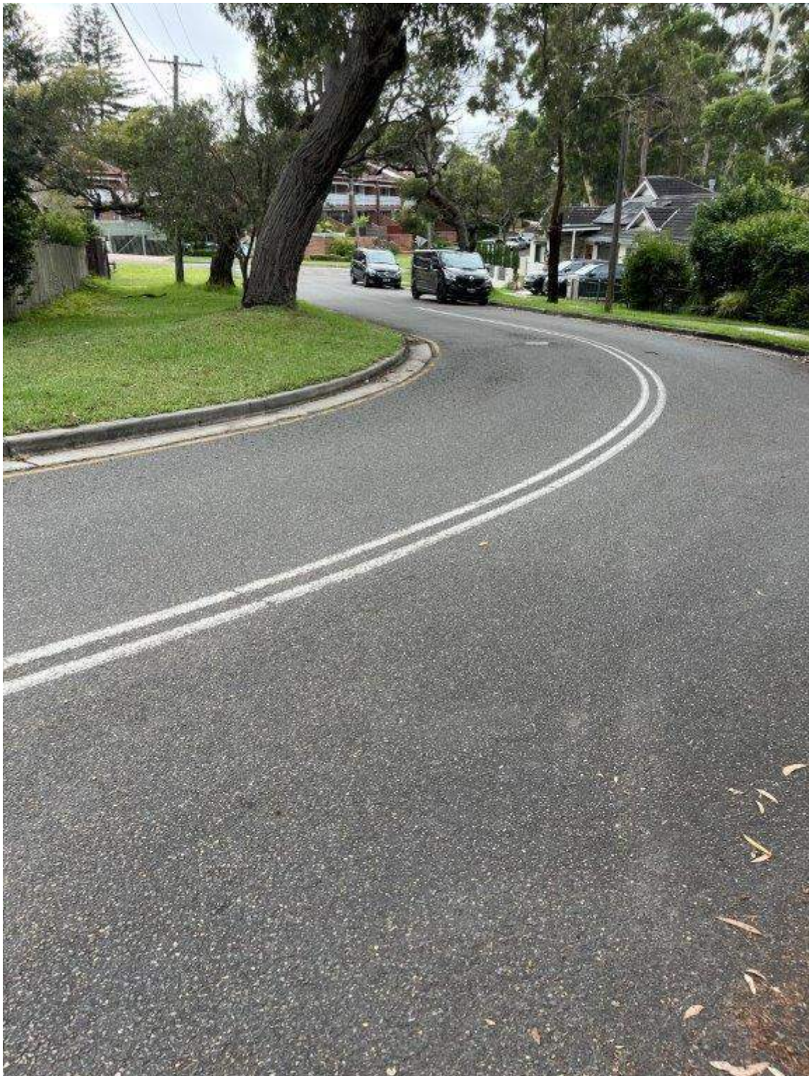
Photo 112 - Hinkler Avenue - Existing condition of pavement
