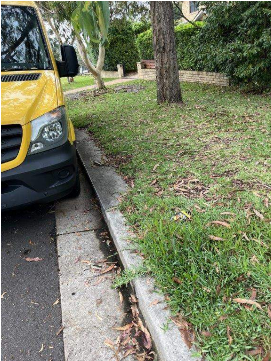
Photo 174 - Taren Point Road - Existing condition of pavement and vegetation
