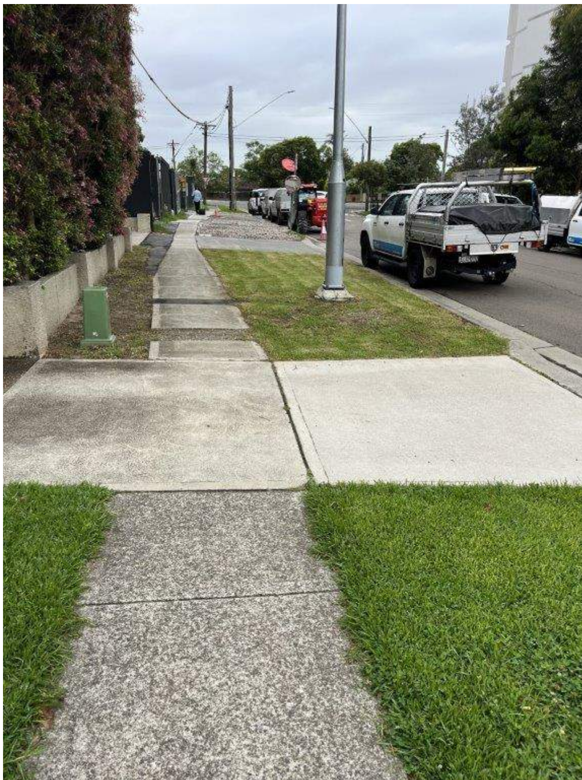
Photo 42 - Hinkler Avenue - Existing condition of pavement and vegetation
