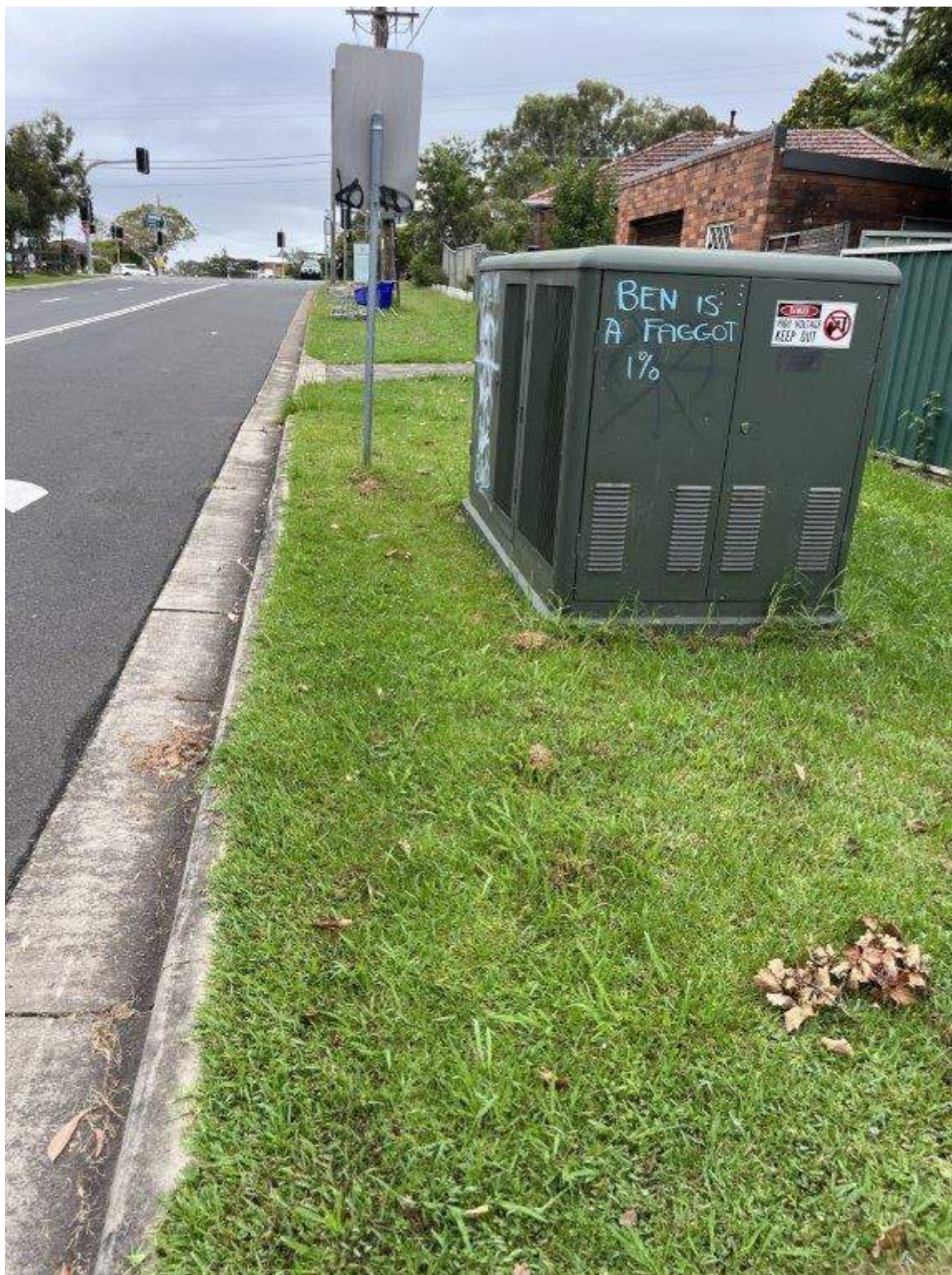
Photo 223 - Taren Point Road - Existing condition of pavement, signpost and vegetation
