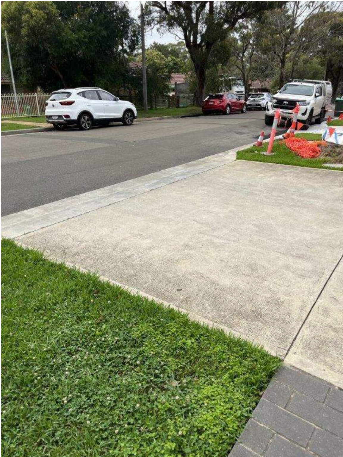
Photo 59 - Hinkler Avenue - Existing condition of pavement
