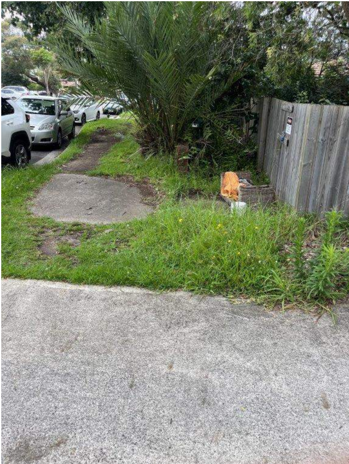
Photo 249 - Taren Point Road - Existing condition of pavement and vegetation
