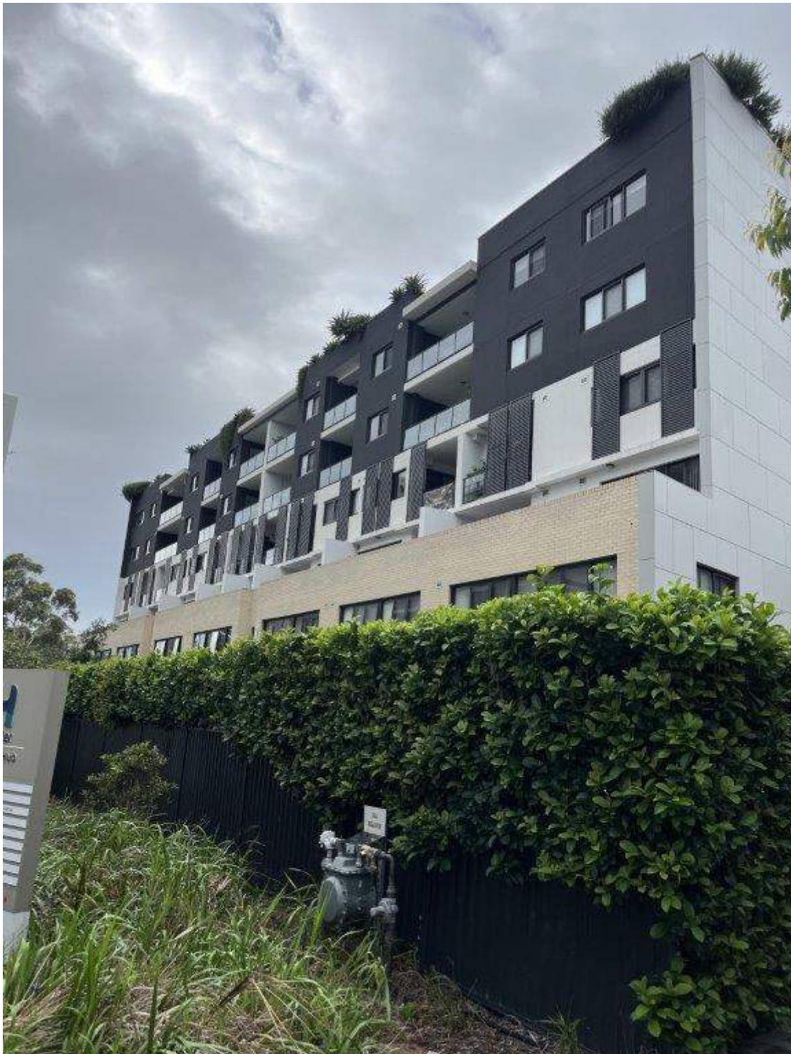
Photo 3 - Hinkler Avenue - Existing condition of external façade
