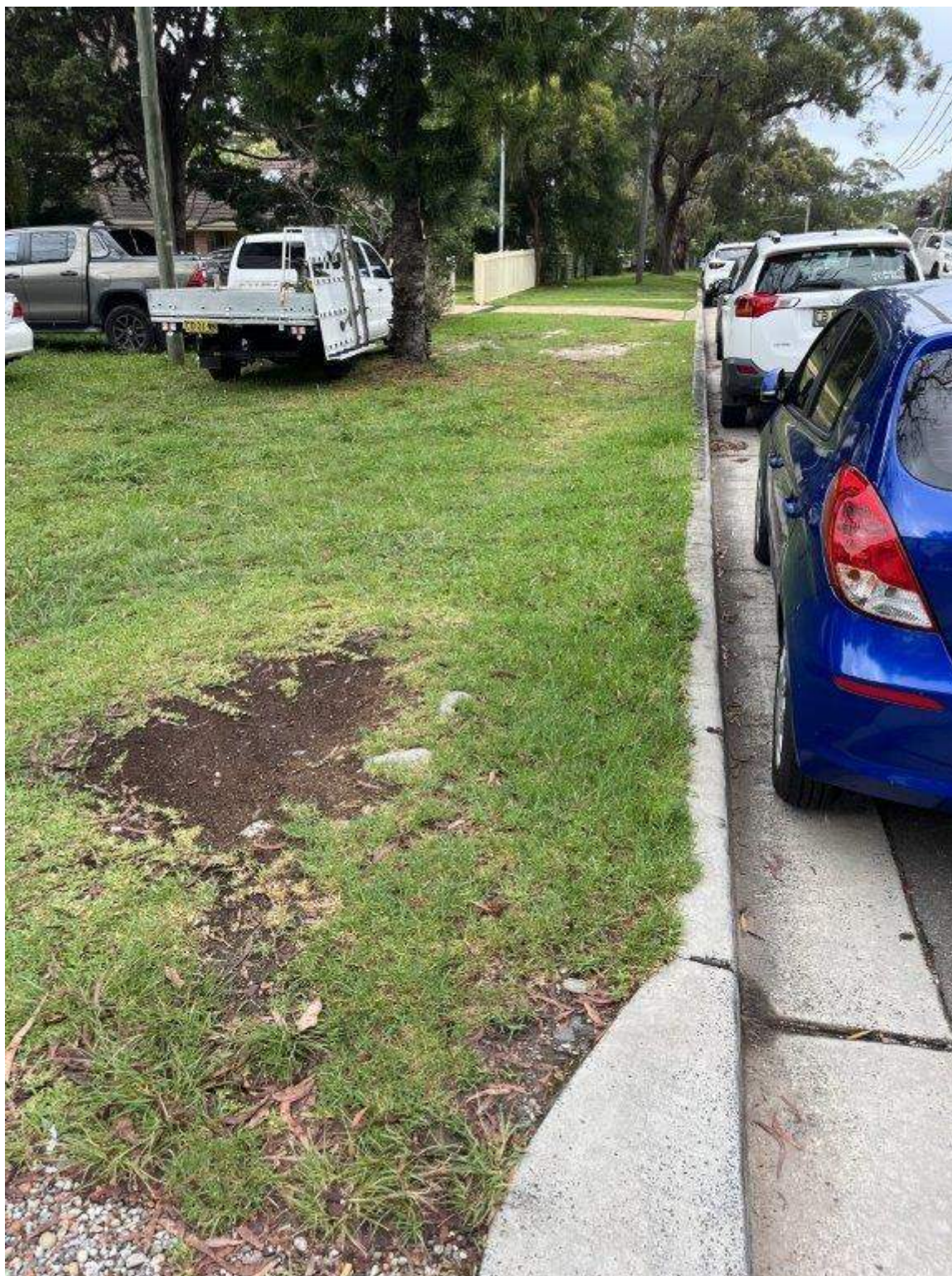
Photo 53 - Hinkler Avenue - Existing condition of pavement and vegetation
