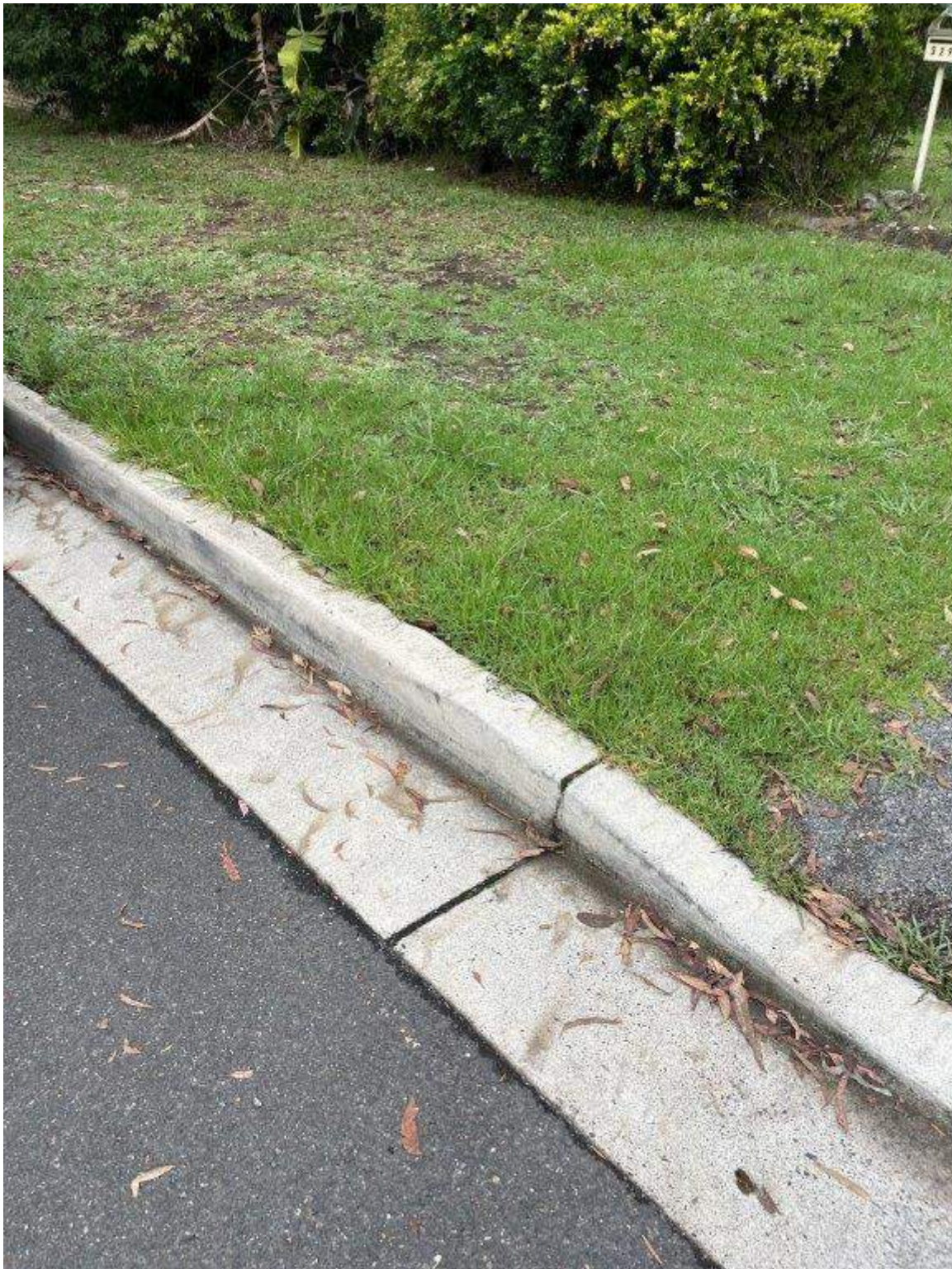
Photo 182 - Taren Point Road - Existing condition of pavement and vegetation
