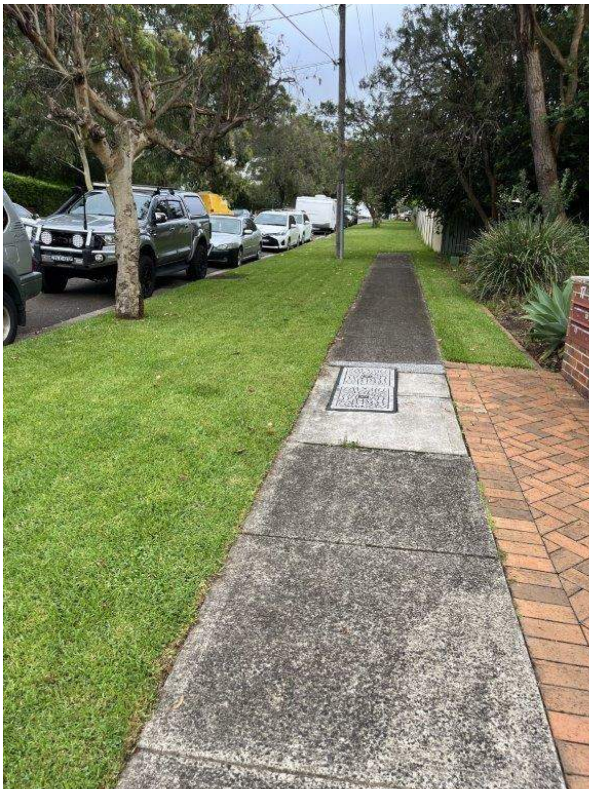
Photo 156 - Taren Point Road - Existing condition of pavement and vegetation
