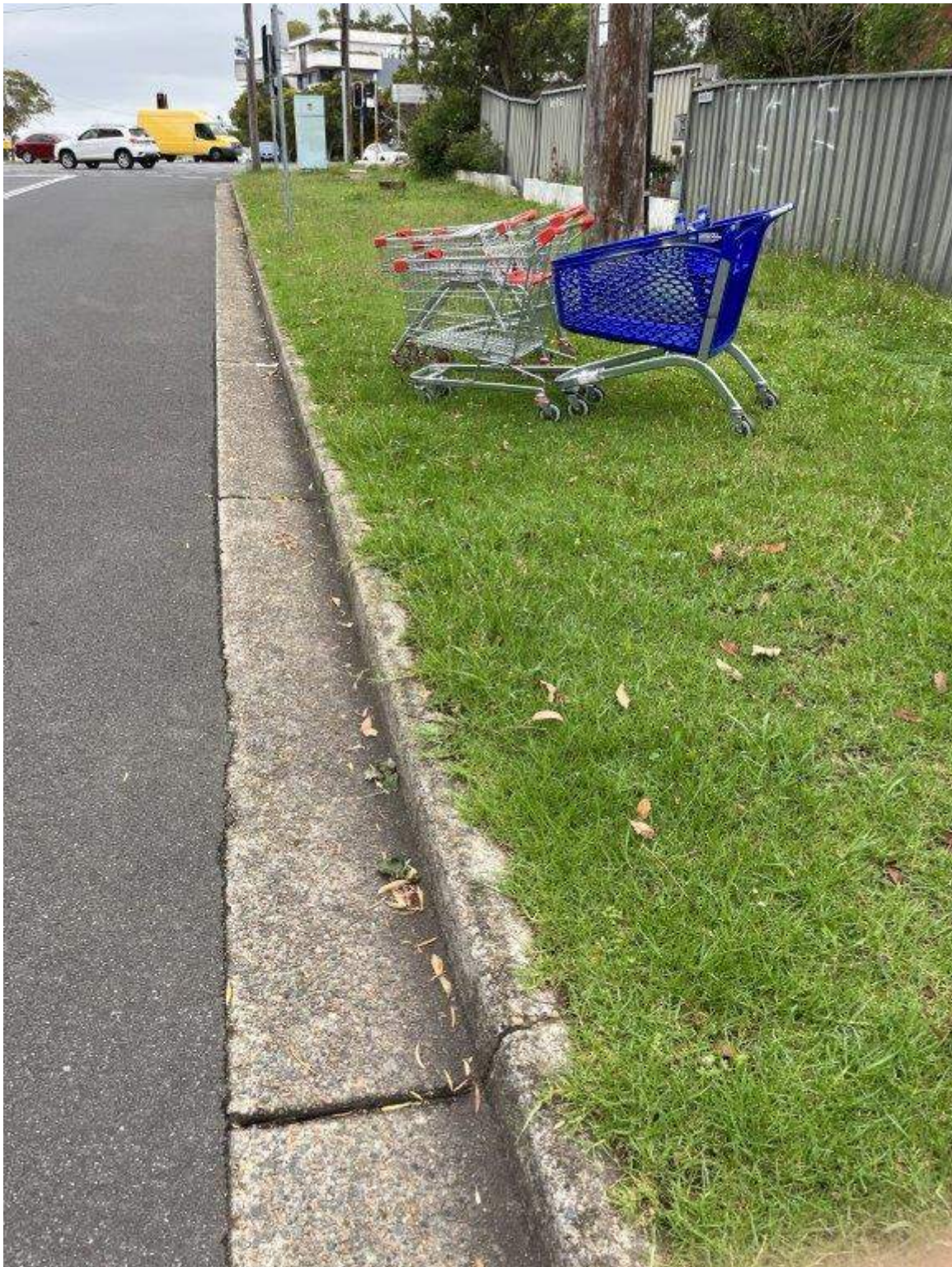
Photo 230 - Taren Point Road - Existing condition of pavement and vegetation
