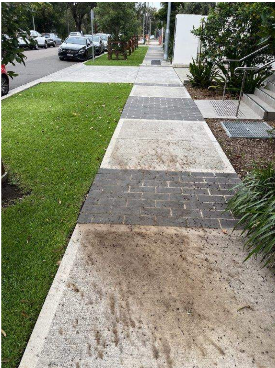
Photo 47 - Hinkler Avenue - Existing condition of pavement and vegetation
