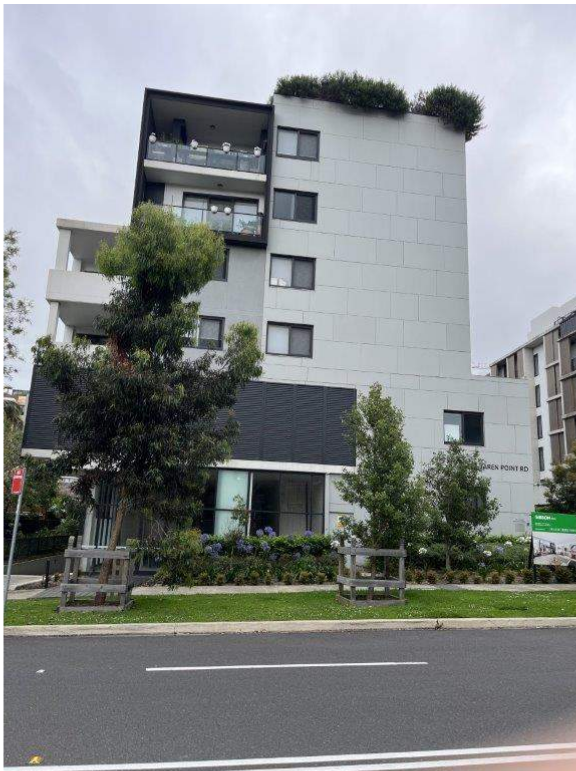
Photo 233 - Taren Point Road - Existing condition of external facade
