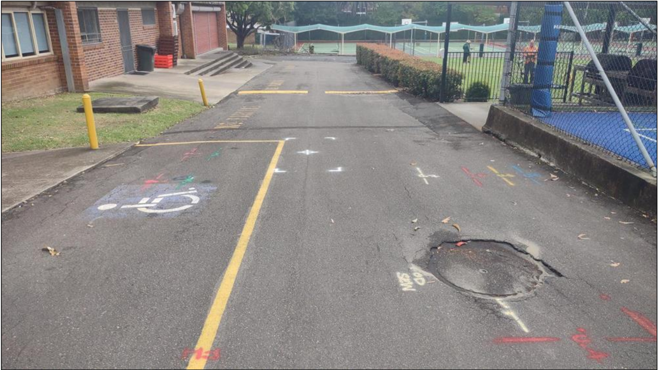
Figure 2: View of the development site, looking north
