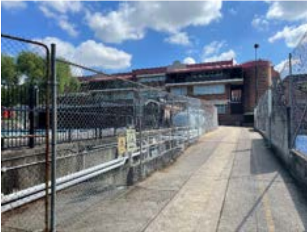
Figure 22 – Level change evident between existing pool (left) and multi-purpose courts (right)
