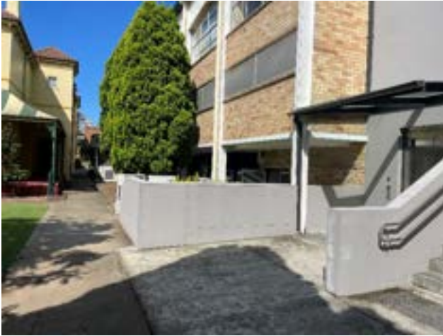
Figure 16 – View east showing pathway between Siena Hall (right) and Rosary Lodge (left)
