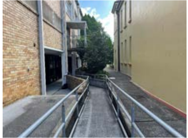
Figure 23 – Level change evident between Siena Hall (left) and Rosary Lodge (right)
