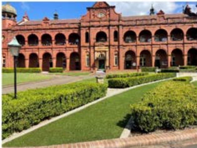
Figure 14 – View south of landscaping to the east of Siena Hall (building in background is outside area of proposed impact)
