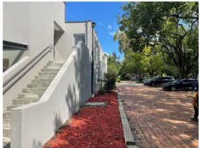
Figure 15 – View south of paved roadway, landscaped garden bed and underground service location to the west of Siena Hall
