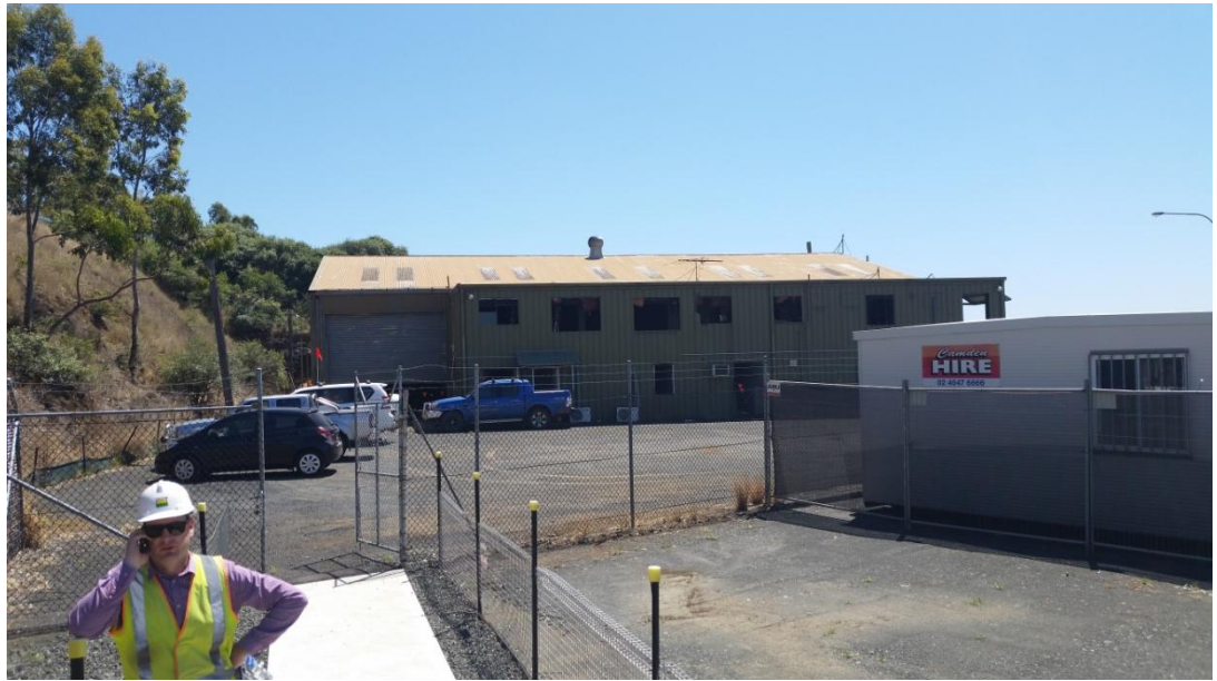
Figure 5: The ACR Shed to be demolished as part of previous approvals.
