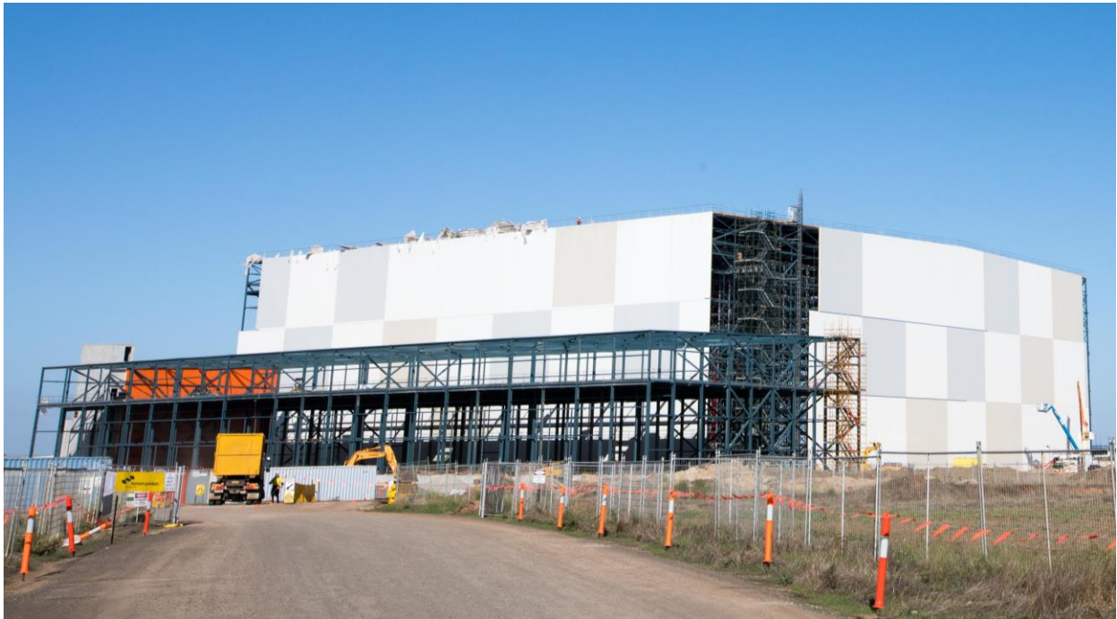
Figure 2: NewCold MB01 projects as at 28 March 2017 (view from construction access trail).
