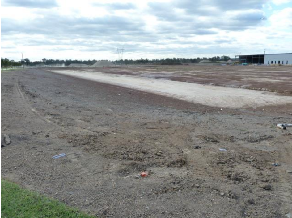
Figure 4 – Photograph of the site from the southwest Source: JBA
