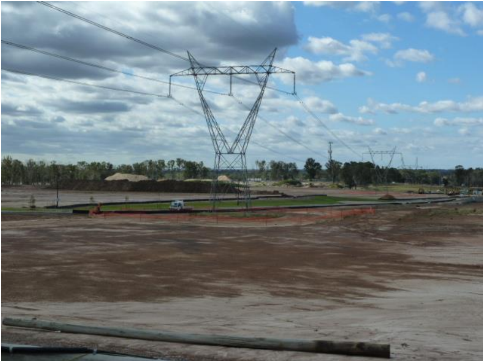
Figure 5 – Transgrid easement transmission towers Source: JBA
