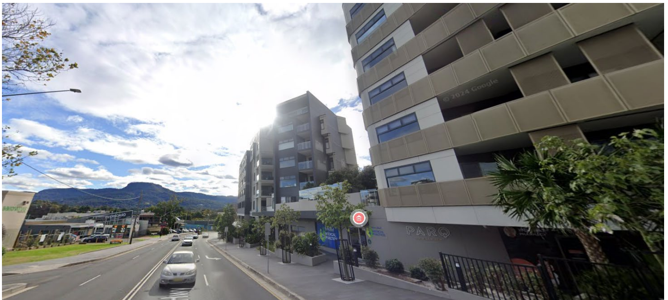
Figure 20 View of Mt Keira seen from the adjoining part of the Princes Highway
