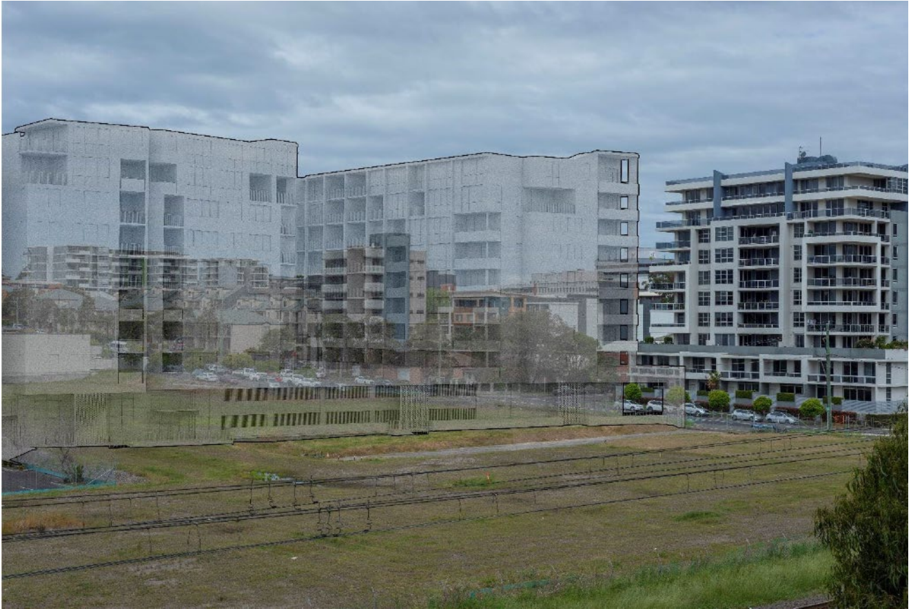
Figure 3 View of the approved development from the Throsby Drive Overpass
