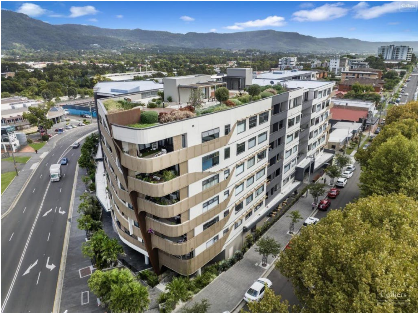
Figure 18 Aerial photograph of the new public space at the north-east corner of the Princes Highway, Smith Street and Keira Street
