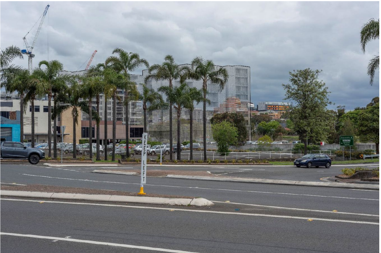
Figure 4 View of the approved development from the Prince Highway
