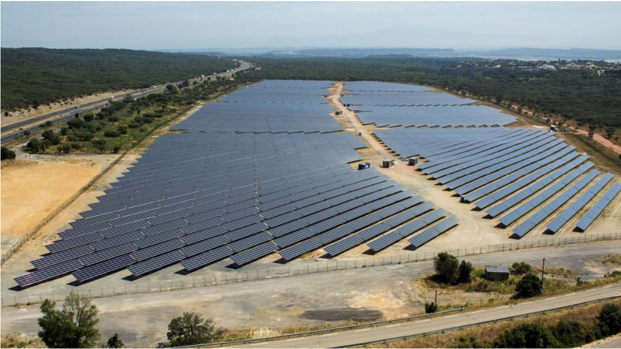
Figure 1-3 11MWp solar project constructed in Rochefort du Gard, France (Source Neoen Australia, 2014)
