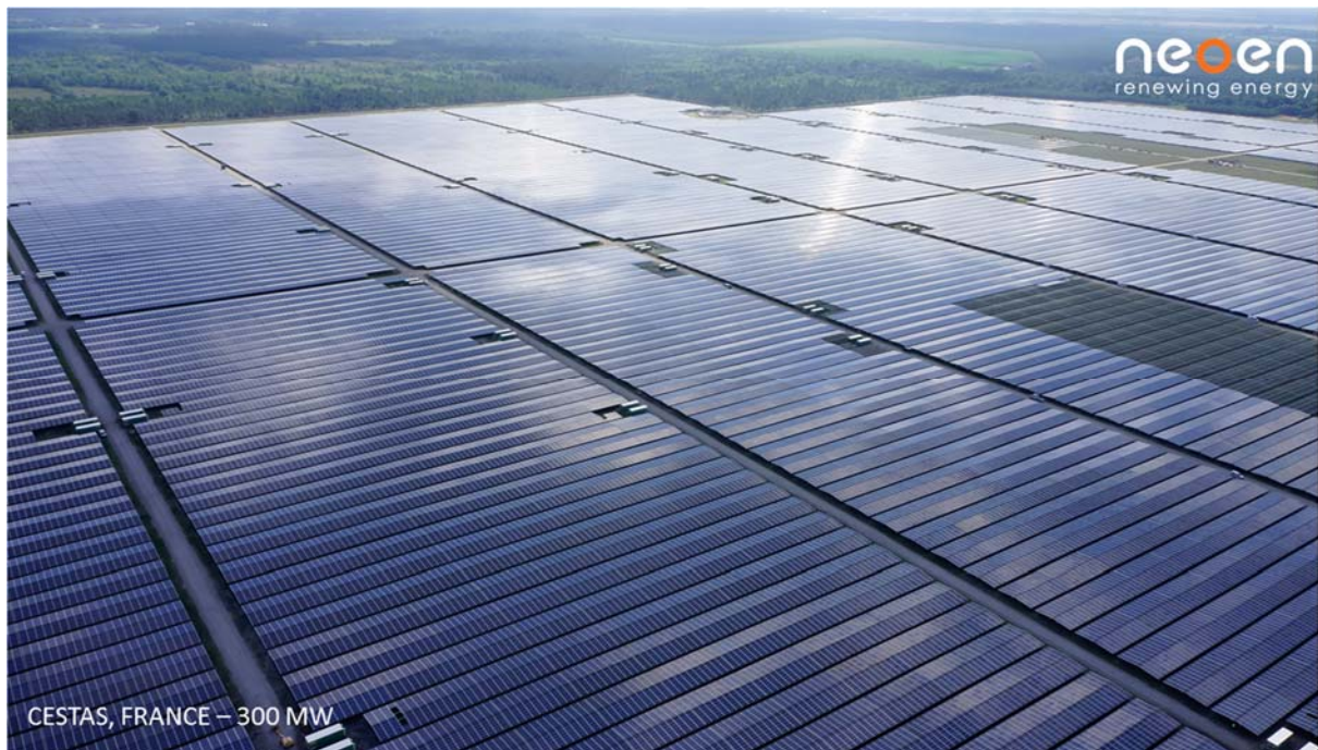
d) Example of east-west facing fixed-tilt mounting system with multicrystalline modules.
