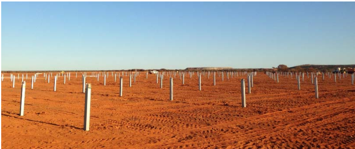
a) Driven piles, during construction.
