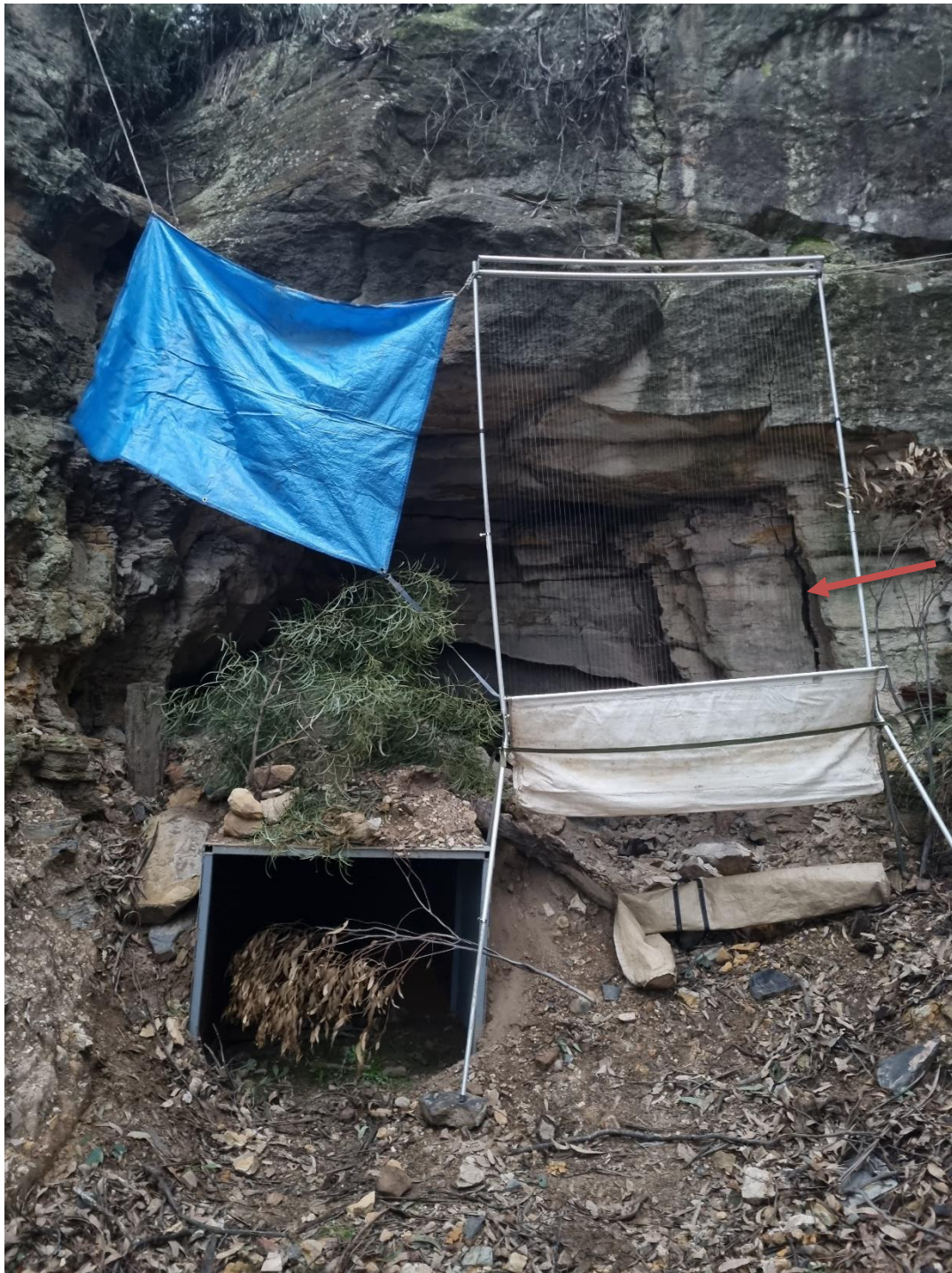
Plate 5-C: Monitoring photos of adit entrance 15 months after installation (July 2024). Harp trapping was conducted to get an update on roost status (species present, sex ratios and recapture of banded individuals). Large crack forming on western side shown with red arrow.
