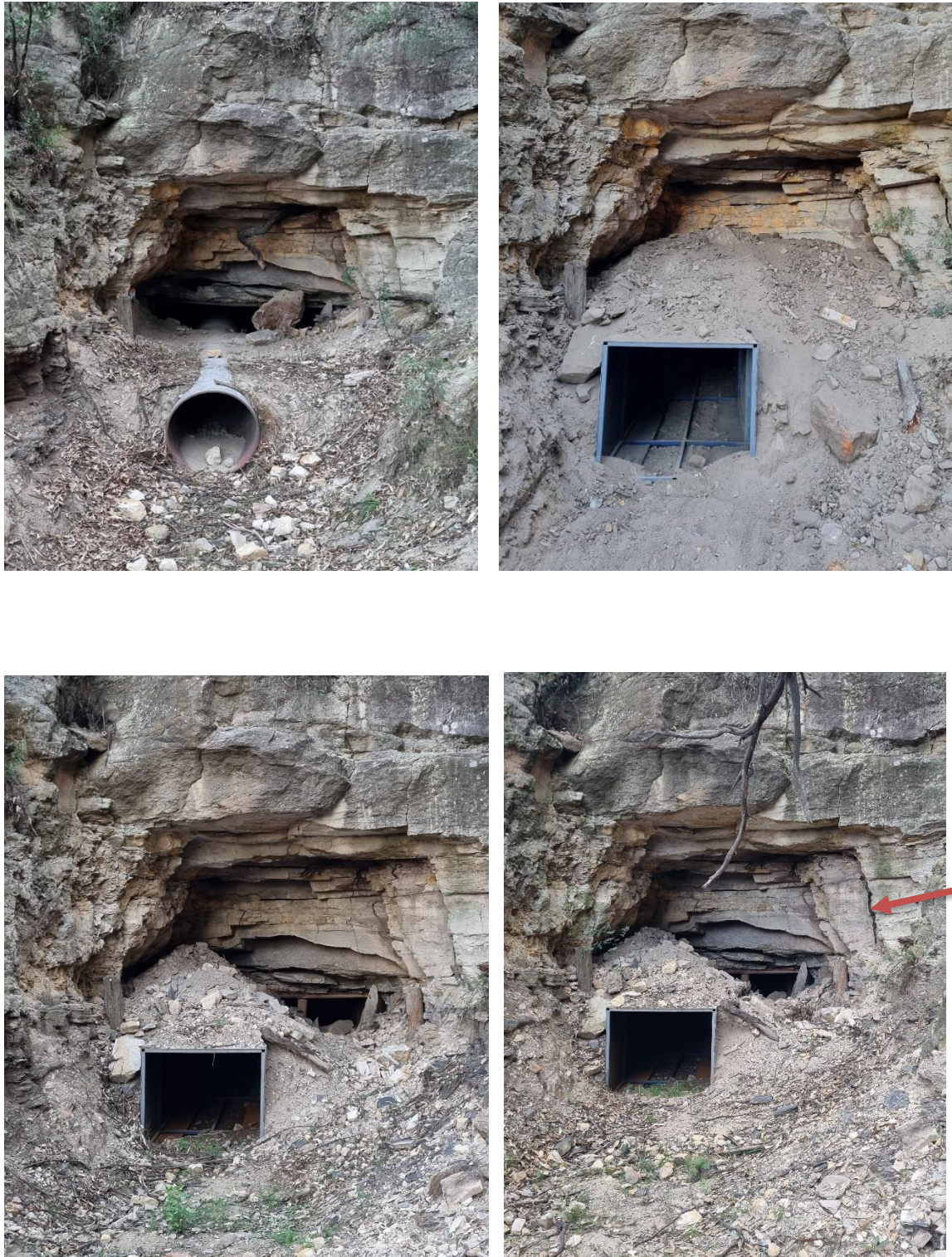
Plate 5-B: Monitoring photos of adit entrance pre culvert installation (March 2023 – top left), afternoon of installation (April 2023 – top right), nine months after installation (January 2024 – bottom left), and 20 months after installation (December 2024 – bottom right). This shows progression of pipe to tunnel with small aperture, tunnel with large aperture. Large crack forming on western side shown with red arrow.
