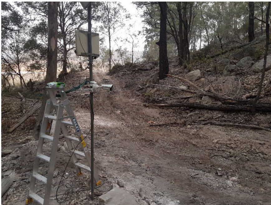
Plate 2-1: Slate Gully adit entrance prior to installation of steel pipe to maintain opening in the event of a collapse (mid 2019), also prior to installation of steel box tunnel (Apr 2023). Detector and solar panel setup 20m in front of adit.
