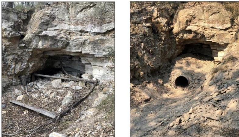
Plate 1 Culvert Support of the Oil Shale Adit 2019
