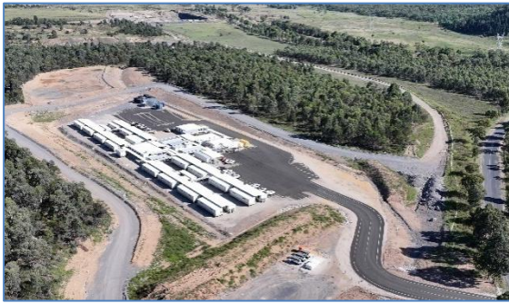
Plate 4: Temporary Accommodation Camp
