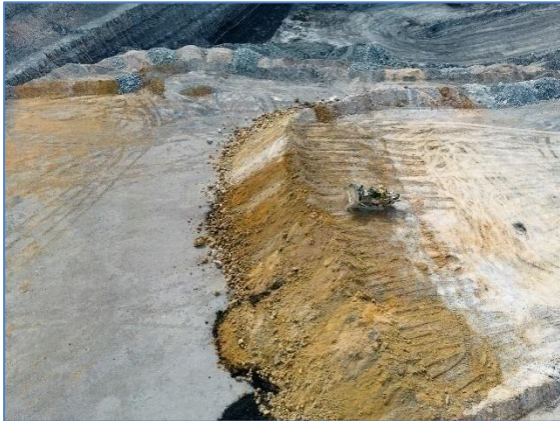
Plate 10: Dozer Working on In-Pit Emplacement
