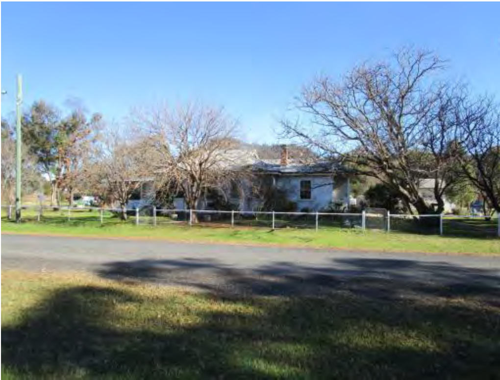
Plate 83. View of former police station.
