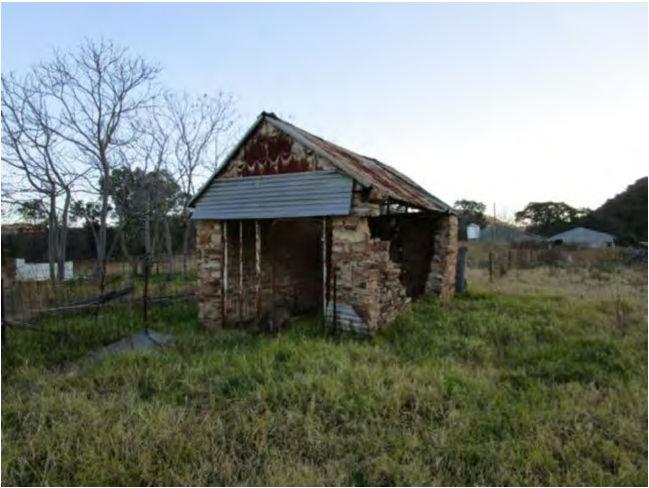
Plate 39. Sandstone shed on Hillview Property
