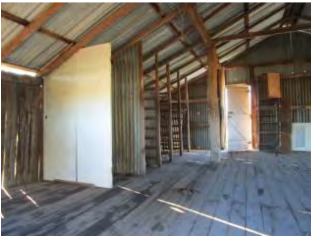
Plate 29. Interior of woolshed.
