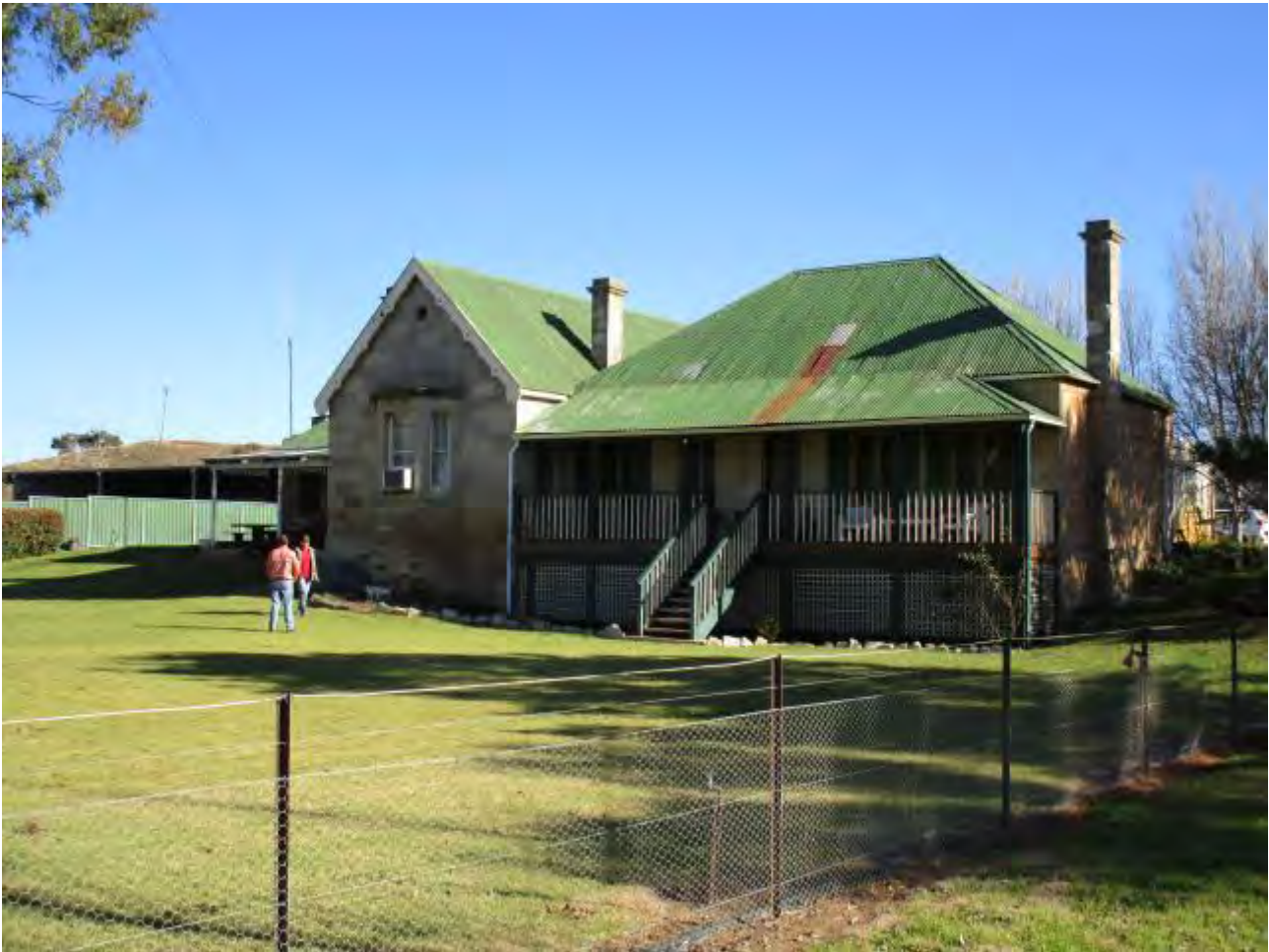
Plate 43. Main residence, northern elevation.
