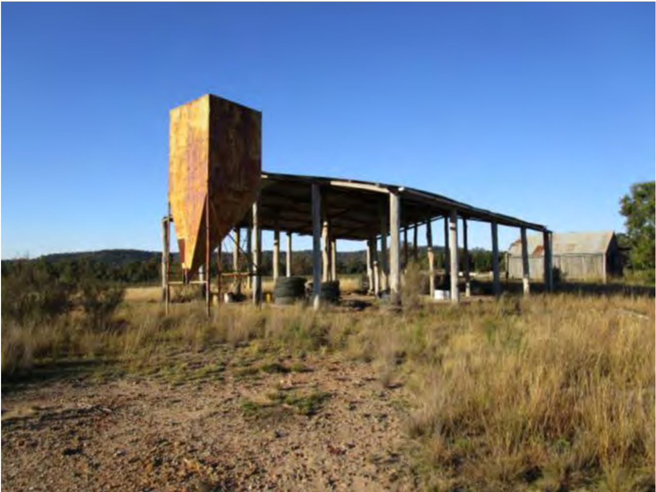
Plate 28. Pine Park grain silo and shed with woolshed in the background
