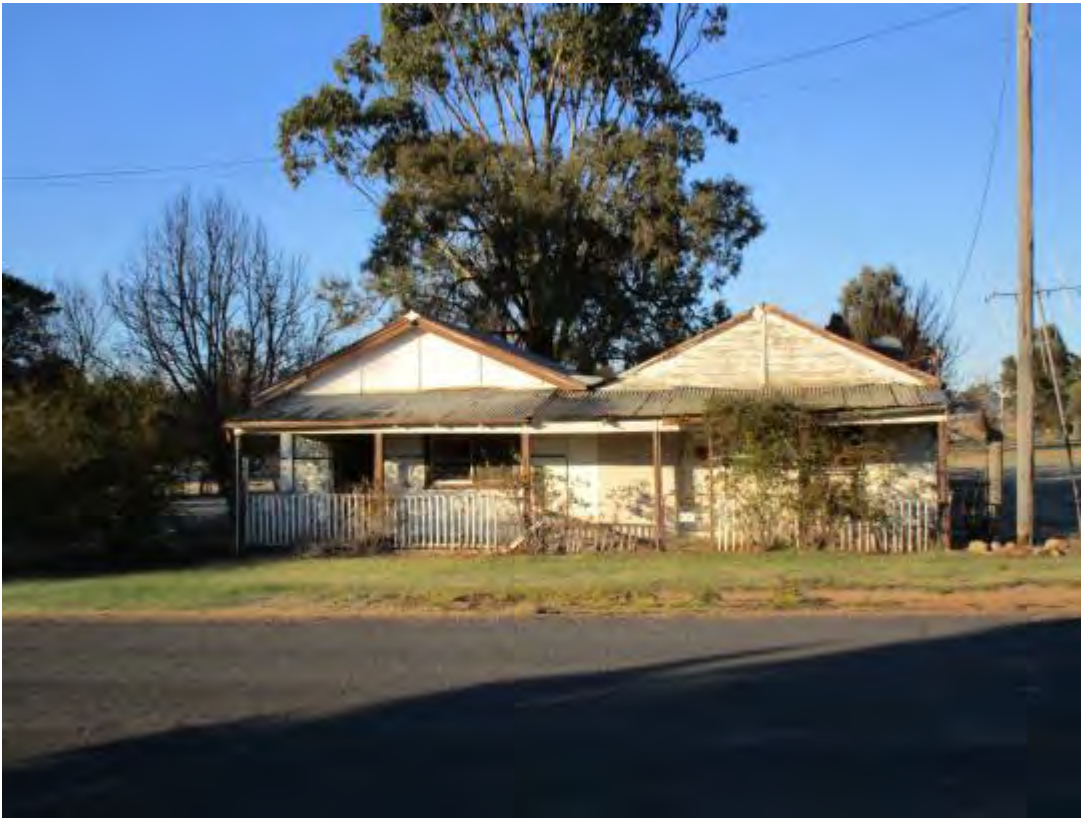
Plate 67. Former butcher and garage.
