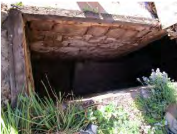
Plate 46. Sandstone lined cellar.
