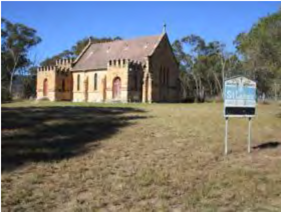
Plate 59. View of the north and east sides of the church.
