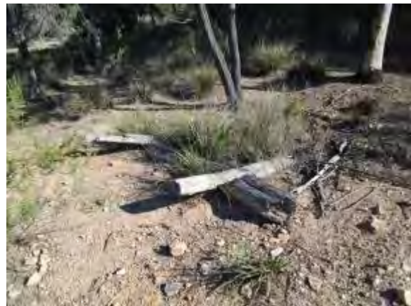
Plate 10. Collapsed post and rail fence.
