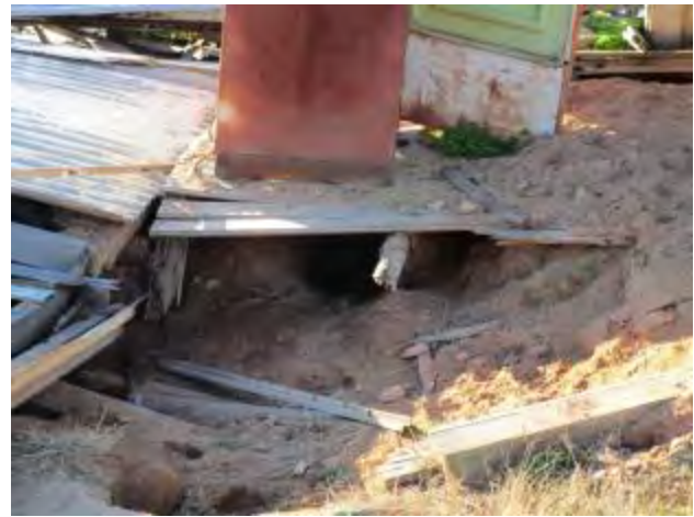
Plate 25. Close-up view of the Cumbo Hut floor foundations.
