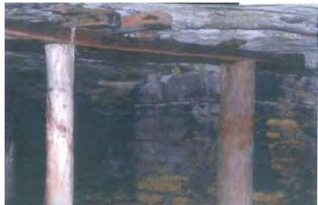
Plate 5. Internal view of Wollar Shale Oil Mine showing support beams, 1997 (Source: Mr and Mrs McDermott).
