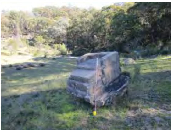
Plate 13. Relocated fireplace from Caretaker's Cottage.
