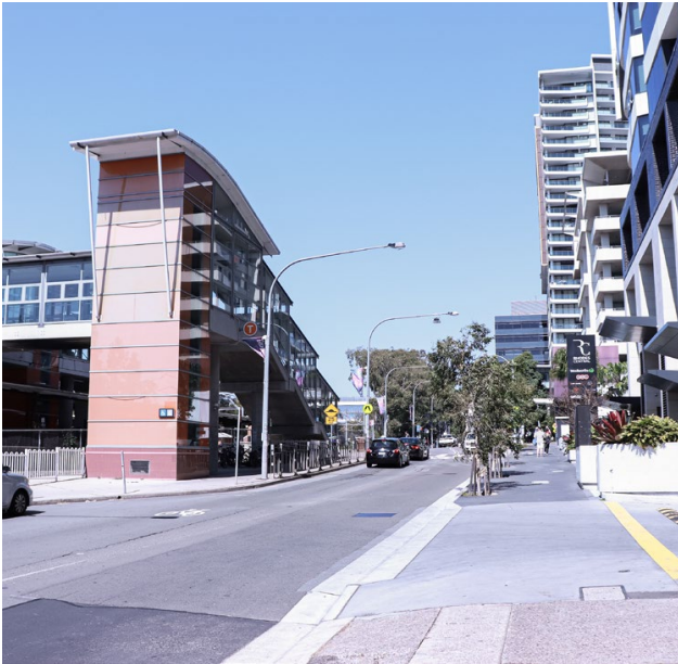
Picture 5 – Rhodes Station on Walker street
