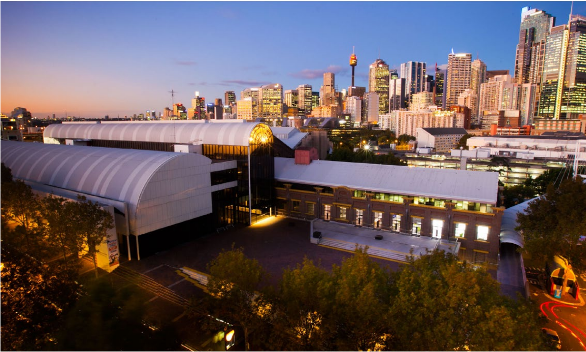
Figure 6 Wran Building and Powerhouse building viewed from Harris Street
