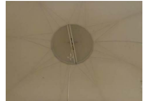
Room316 internal view of top of dome
