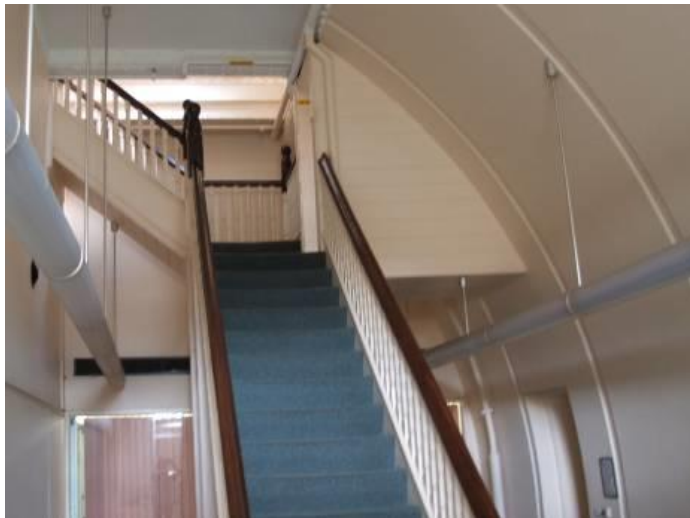
Timber stair eastern dome
