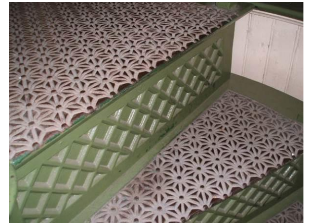
Typical cast iron treads to stair
