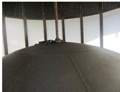
Adjustable steel umbrella at top of dome in domed roof light
