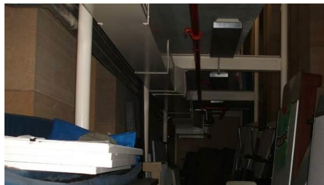
Steel supports for mezzanine slab room G17b
