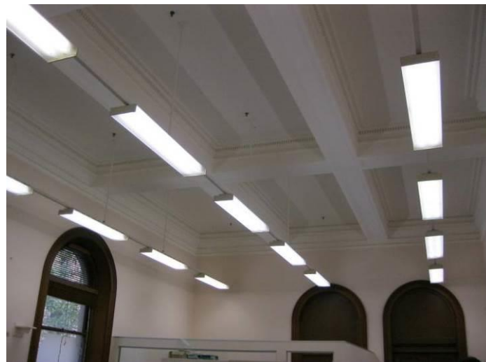
Uni strut / chain Suspended 2x65W T12 luminaires with prismatic diffusers.
