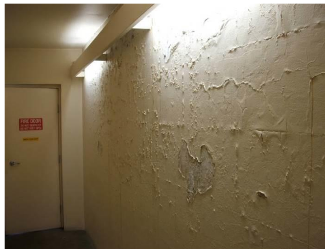
Service corridor at Level 4
