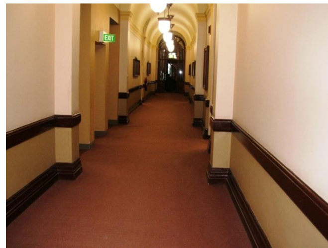
Typical corridor Upper Floors
