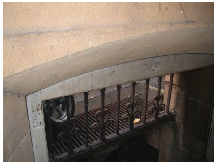
View of footpath grates into moat
