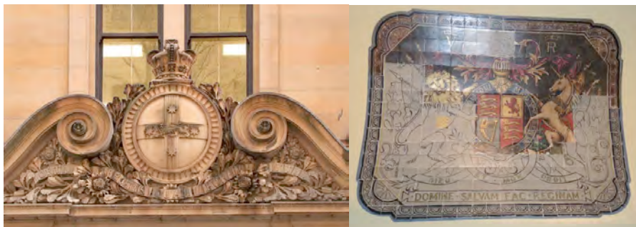
Figure 5: Externally James Barnet adorned the Loftus Street façade with the heraldic insignia which would subsequently be adopted by the NSW government as its heraldic symbol on its coat of arms (left). Inside, sovereignty to Queen Victoria was expressed in the Royal coat of arms in tile work, embedded into the fabric of the building (right). (Photos C Betteridge 2013)
