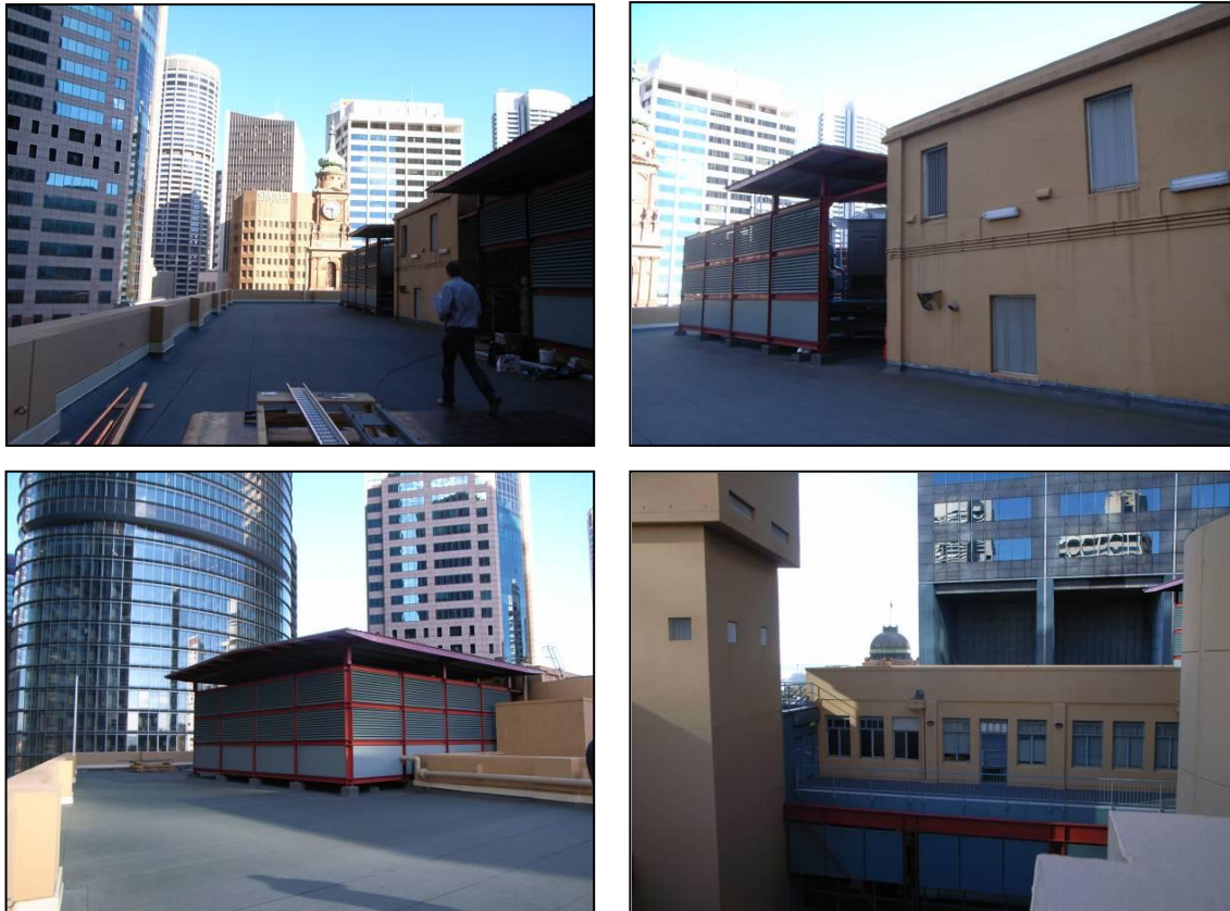
Figure 4.28: Rooftop with steel framed plant rooms and view onto internal courtyard towards Level 8
