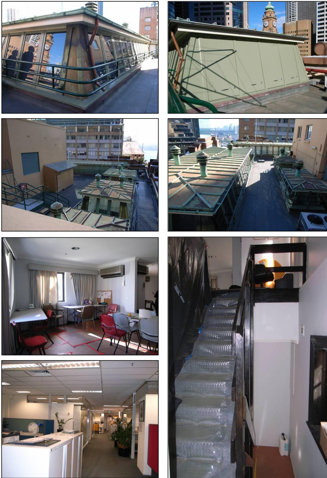
Figure 4.25: Internal views of Level 8 rooftop with sky lanterns, guest teacher accommodation (caretaker's flat) above the 1915 Department of Education building section, and office fit-out above the 1930 Department of Education building.
