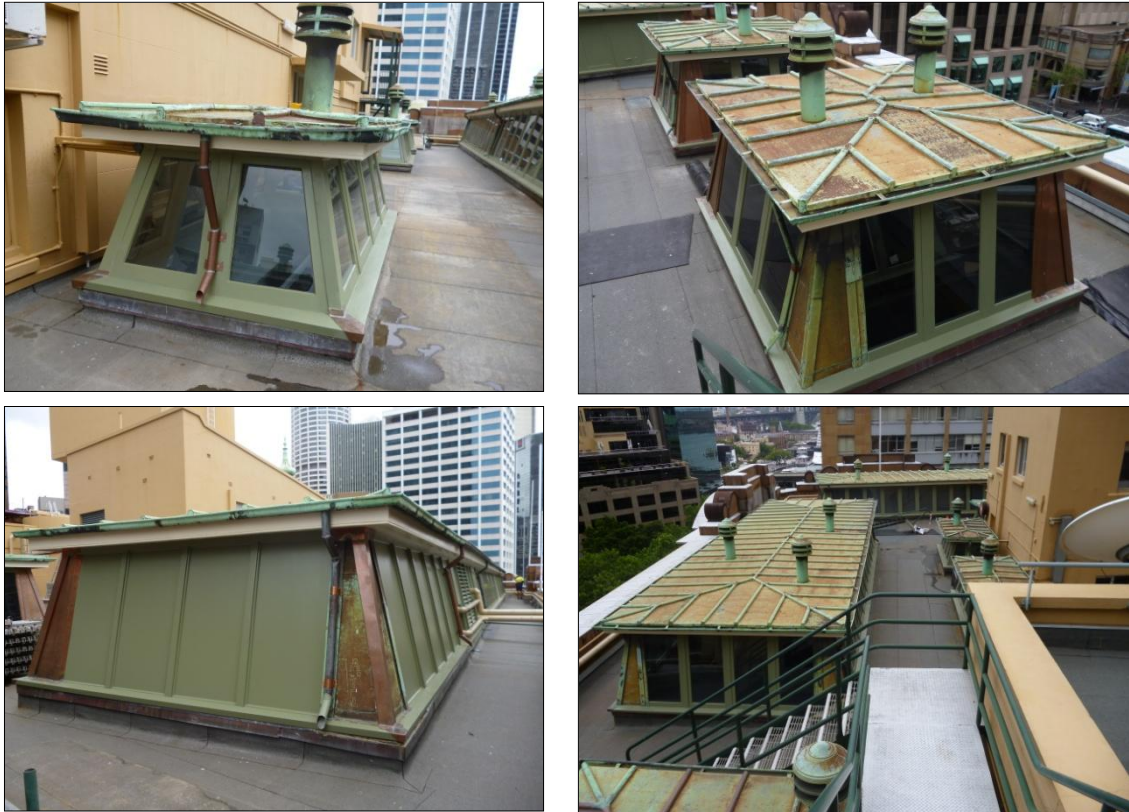
Figure 4.26: Sky lanterns after completion of repair and conservation works
