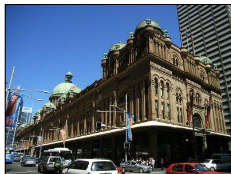
Figure 6.4: Queen Victoria Market Building, view from Town Hall (Source: NSW Heritage Division, Claudine Loffi)
