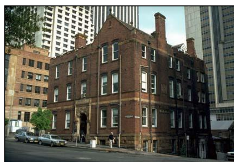
Figure 6.11: Health Department Building at 93 Macquarie Street
