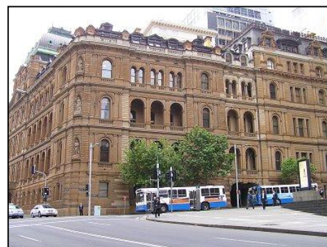
Figure 6.8: Chief Secretary's Building at 121 Macquarie Street corner with Bridge Street (Source: State Heritage Inventory, Stewart Watters)
