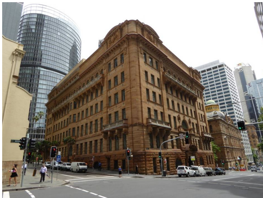
Education Department Building with Lands Department in the background (GBA)
