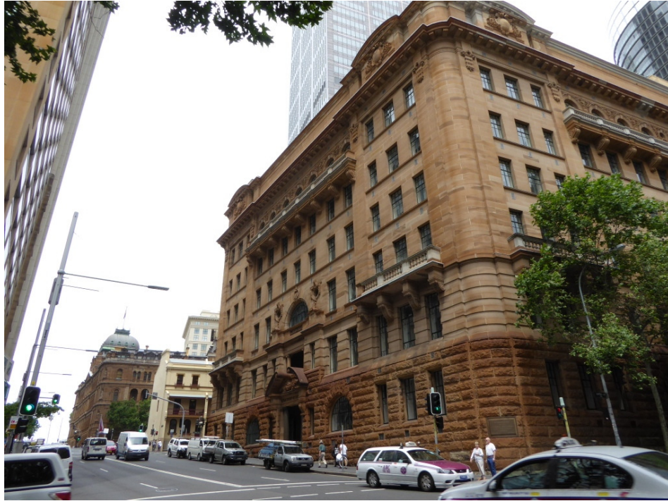
Education Department Building looking east along Bridge Street towards the Young Street Terraced Houses and Chief Secretary's Building in the distance. Only the Young Street buildings are sufficiently close to the Education Department Building to potentially be affected by the potential roof top addition. (GBA)
