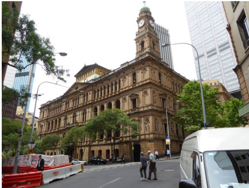
The Lands Department Building, with its distinctive corner tower and richly decorated sandstone façade, viewed from Spring Street (GBA)
