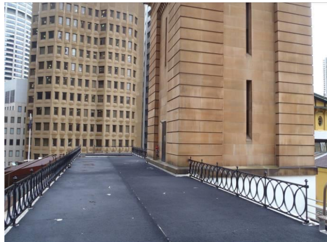
Southern membrane roof adjacent tower
