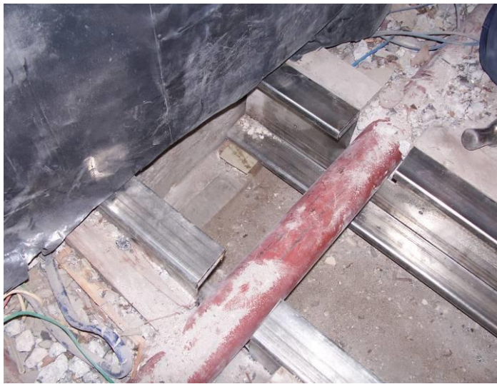
Room 219 stabilisation of timber floor
