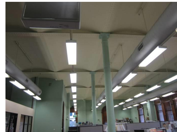
Room 302: Vaulted ceilings: High Significance.
