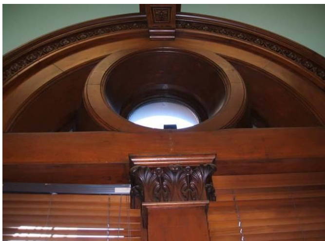
Window joinery on level 1 Room 104
