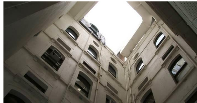
Part of northern lightwell
