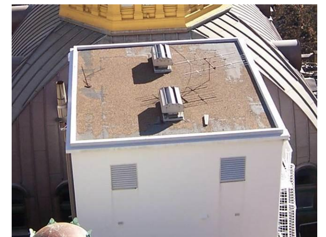
Lift motor room membrane
