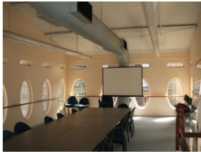
Interior of upper floor in pavilion
