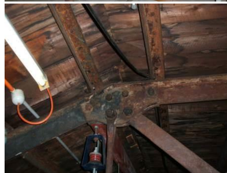
Timber boarded underlay
