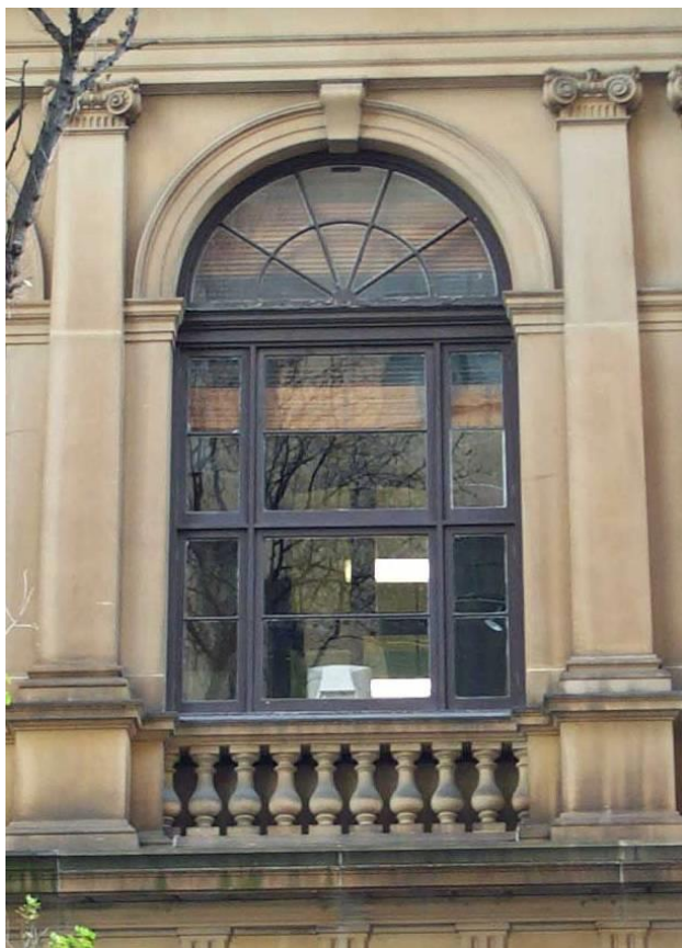
Sills cracking, some rot & failing paint
