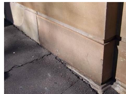
Typical stonework condition at footpath
