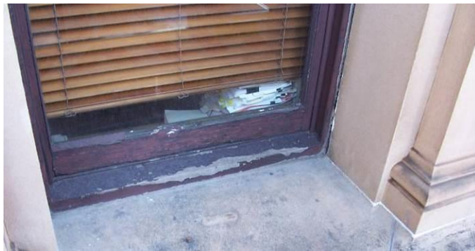
Sills cracking, some rot & failing paint
