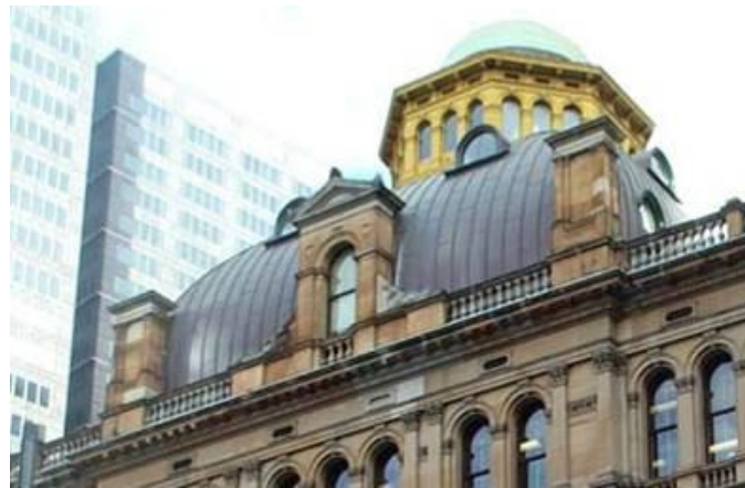
Northern dome chimneys at northern corners
