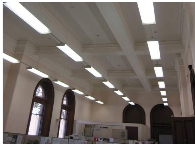
Room 105: Coffered ceiling: High Significance
