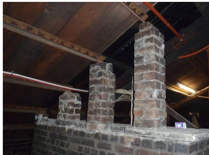
Chimney terminated in roof space
