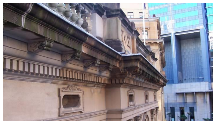
Projecting cornice stones with brackets below
