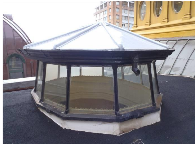
Viewed from south
