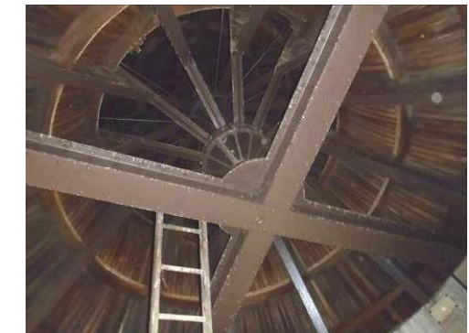
Inside tower dome
