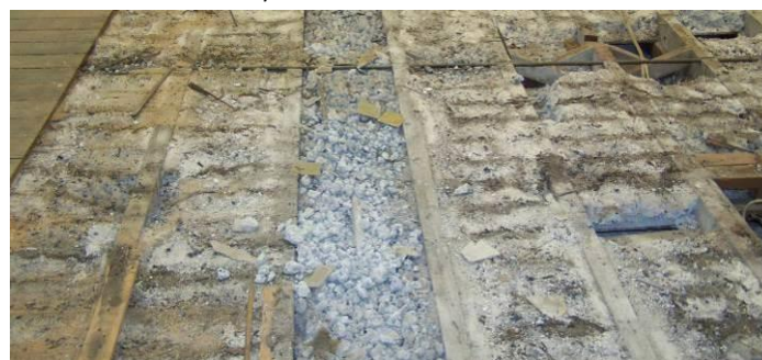
Room 219 lightweight concrete between floor joists
