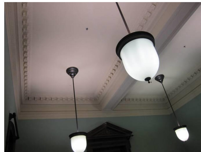
Room 207: Decorative moulded ceilings. Exceptional Significance
