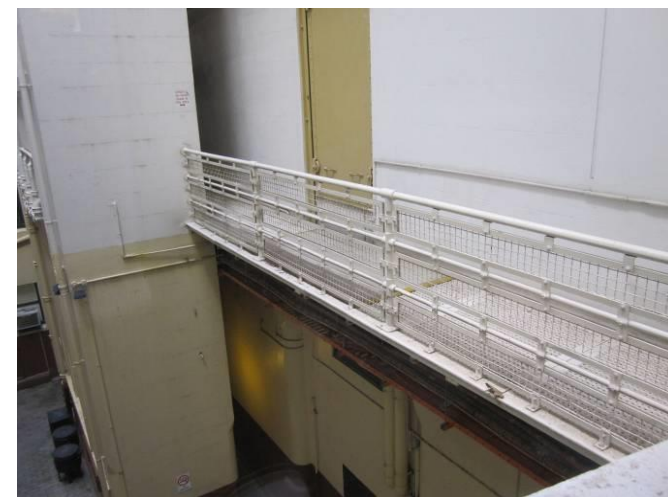
Suspended walkways to toilets
