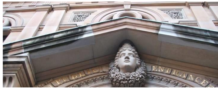
view of bridge street entrance stonework with past stone replacement
