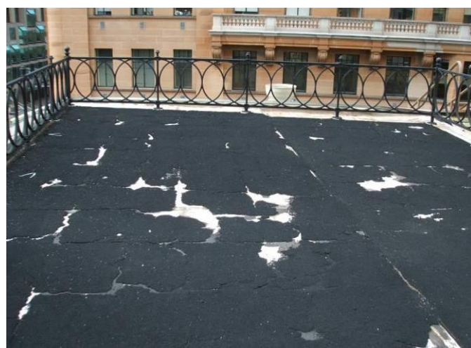
Membrane east of northern dome
