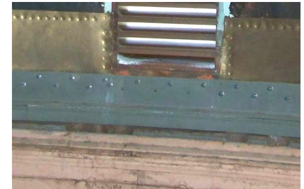
Copper dome track with cannon balls
