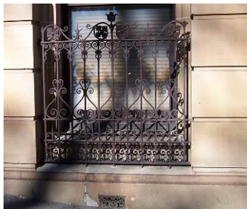
Bridge Street stage 1 Window grilles
