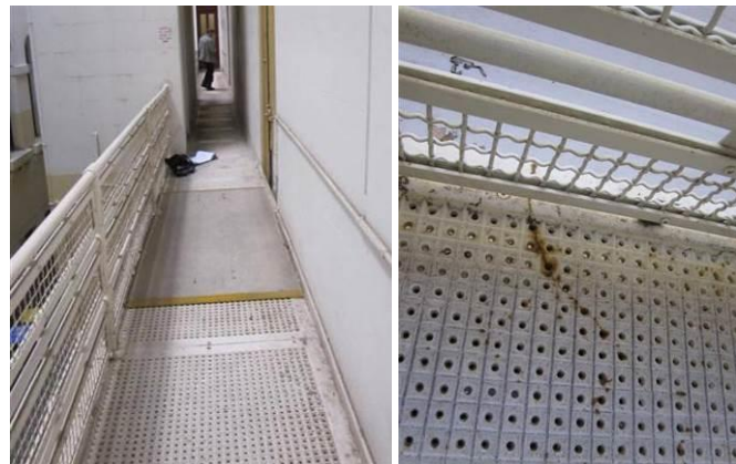
Cast iron catwalks
