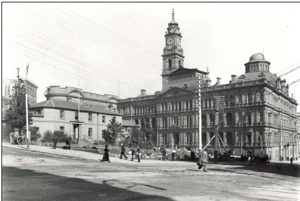
Figure 3.5: Work begins on the site for the new offices of the Department of Public Instruction in the front garden of their existing offices, where the Moreton Bay fig has been cut down.
