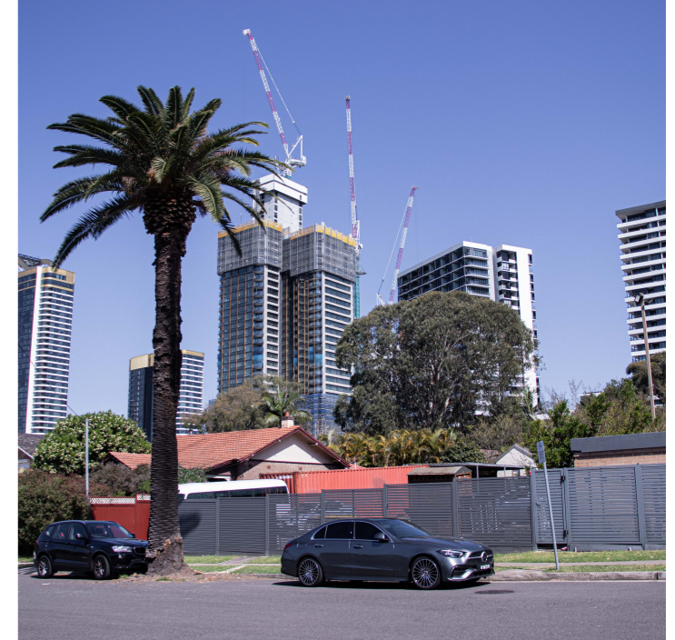
9. North East corner of site
