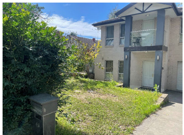
Figure 22 – View of the subject area along Blaxland Road. Note the terracing of the lot to accommodate the multi-storey residential building.
