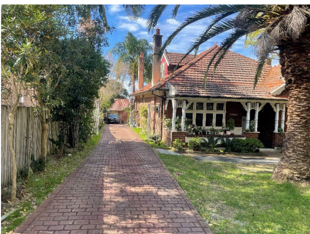
Figure 21 – View of the subject area along Blaxland Road.
