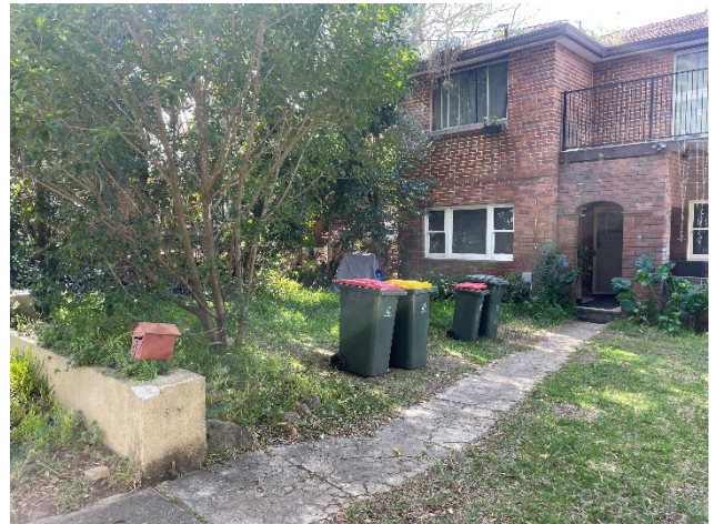
Figure 20 – View of the subject area along Blaxland Road.
