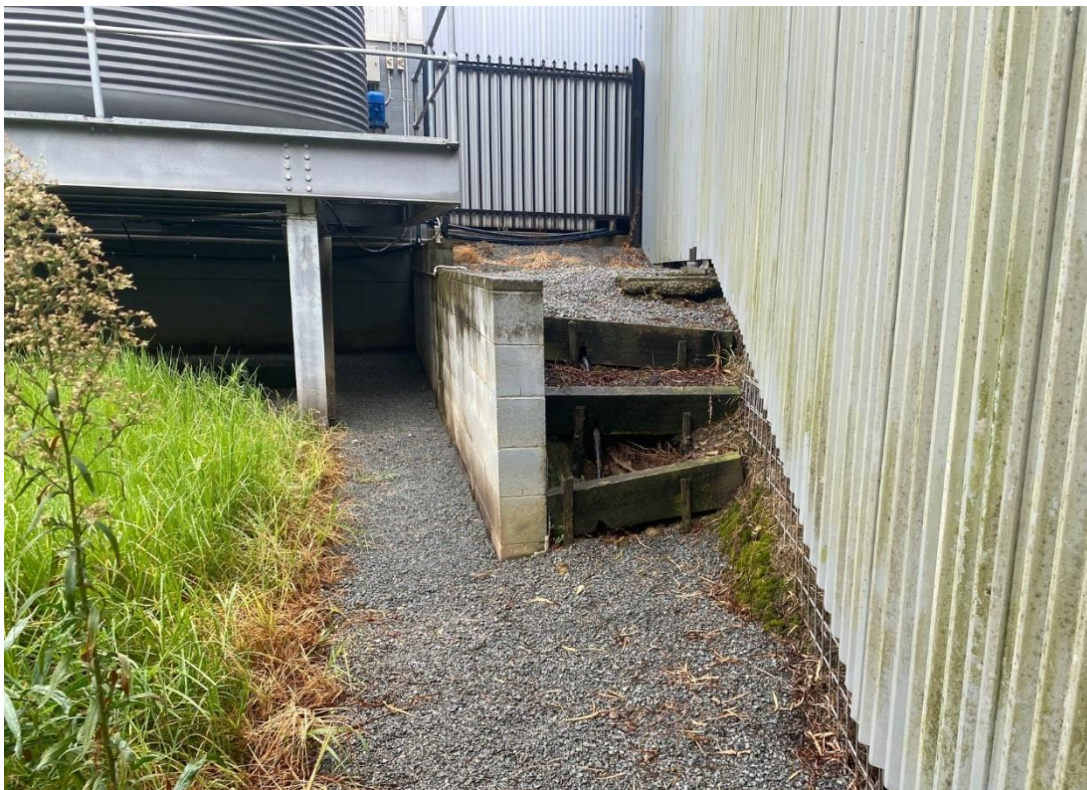
Photograph 4.3 Example of potential shelter habitat within the green patch, and gaps at the base of the fence
