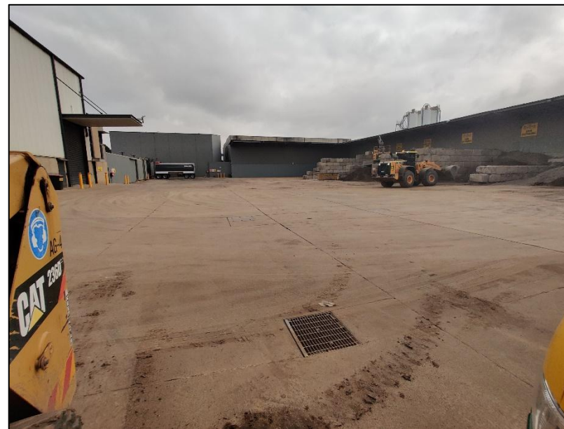
Photograph 2: Hardstand area of the site and material bays. Facing west.
