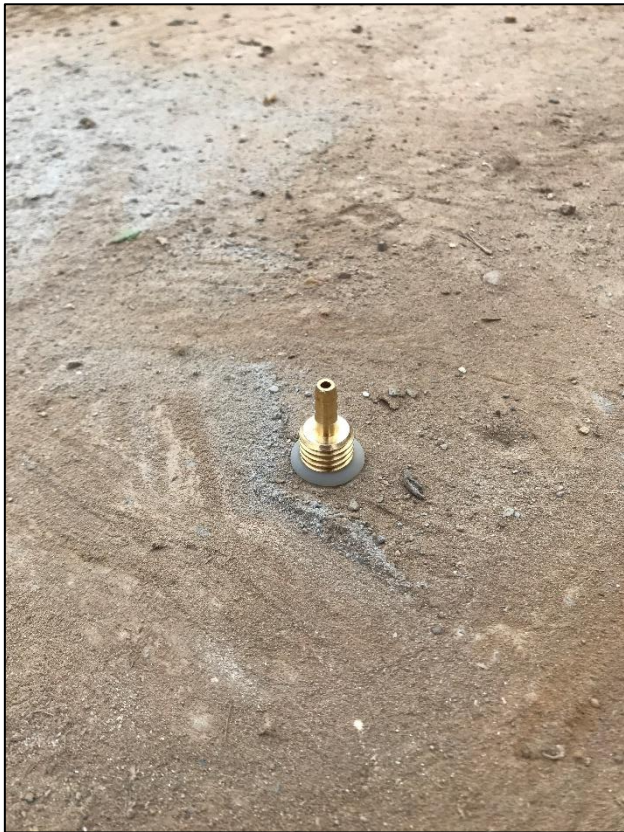
Photograph 8: Temporary Vapor Pin and silicon sheathing
