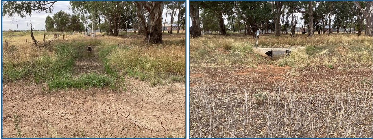
Image 6: Facing east from the farm distribution channel on the eastern boundary of the site, pipe under Hulme Road and Yanco Substation and water authority irrigation channel in the background (left); area where sample was taken outside of first gate on the farm distribution channel on the eastern boundary of the site where water is released onto the site (right).
