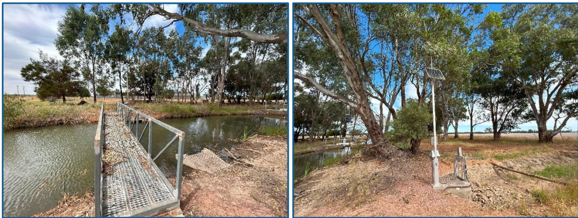
Image 4: Water authority irrigation channel running parallel to Yanco Substation (left); slide gate to channel that enters a pipe under Hulme Road into the farm distribution channel on the eastern boundary of the site (right).
