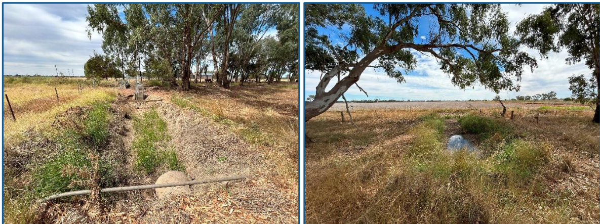
Image 5: Slide gate to channel and pipe under Hulme Road (left); facing west onto the site, water sitting in the channel at exit of pipe under Hulme Road to farm distribution channel on the eastern boundary of the site (right).
