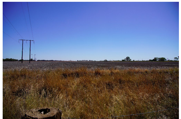
FIGURE 5-4 TRANSMISSION LINES CROSSING PROPOSAL SITE
