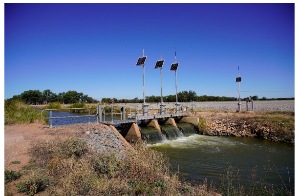
FIGURE 5-3 IRRIGATION CHANNEL NORTH OF PROPOSAL SITE
