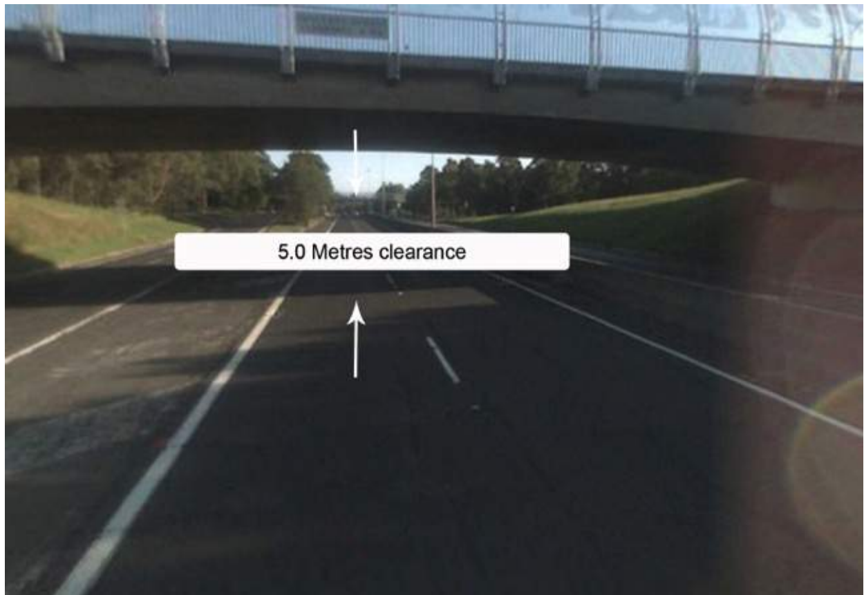
Figure 10 - University Overbridge on the Southern Freeway
