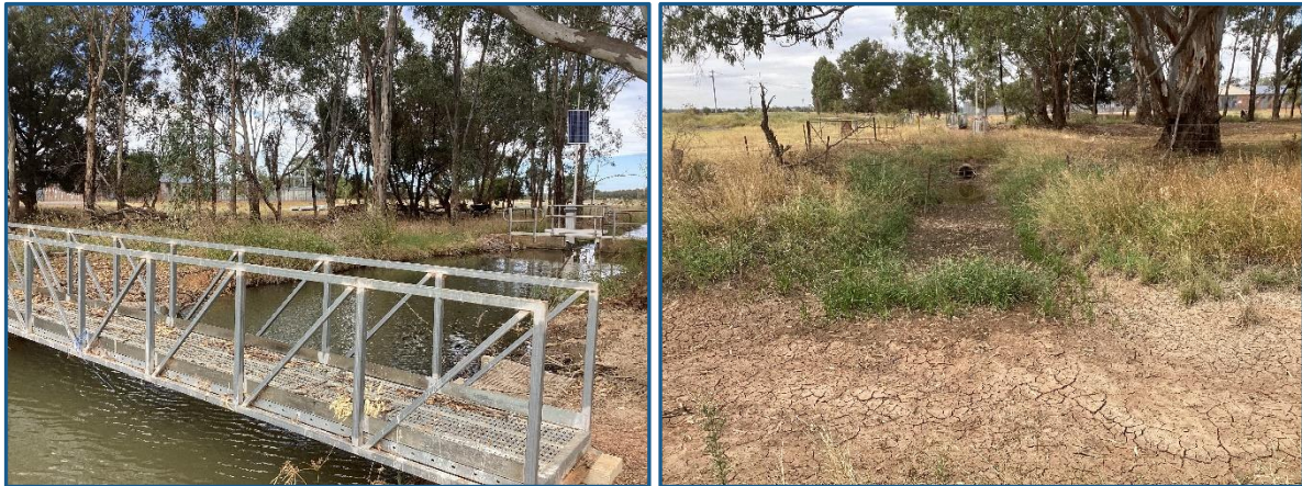
Image 7: Water authority irrigation supply channel parallel to eastern boundary of the site and Hulme Road adjacent to the Yanco Substation pictured in the background (left); irrigation outlet and culvert allowing water to be released from the water authority supply channel into the farm irrigation water distribution channel along the eastern boundary of the site (right).
