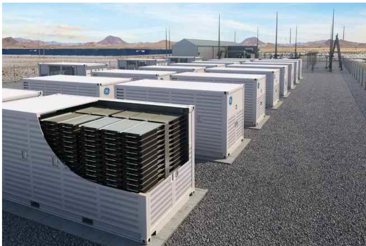
Figure 3-4: Typical BESS Arrangement
