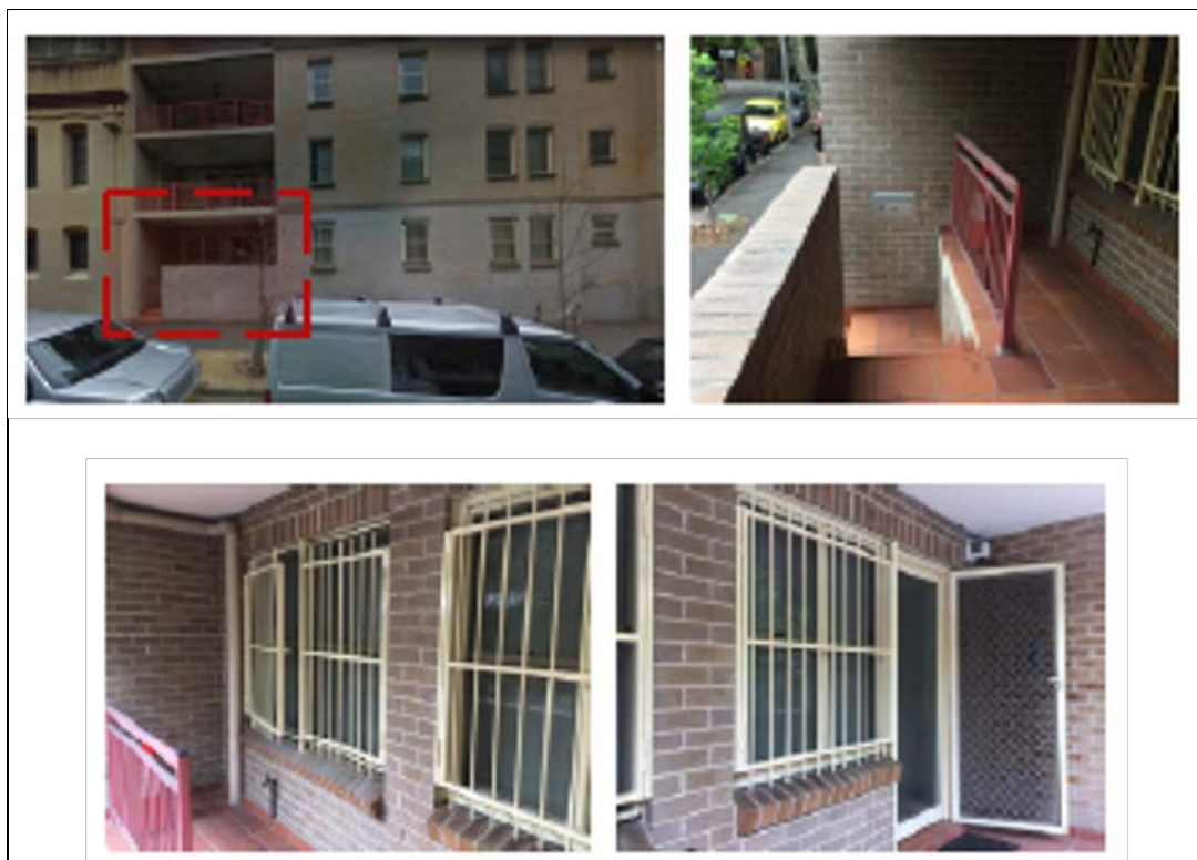
Figure 12 | Unit 29/ 23 Buckland Street, street view, entry porch and windows
