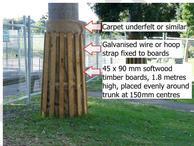
Figure 3 – Detail of Trunk Protection
