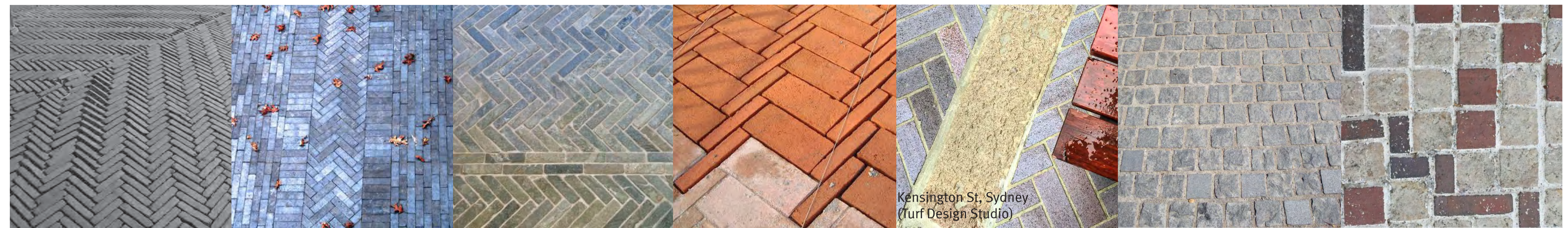
Public domain brick paving | herringbone pattern | stone or concrete inserts | granite stone setts
