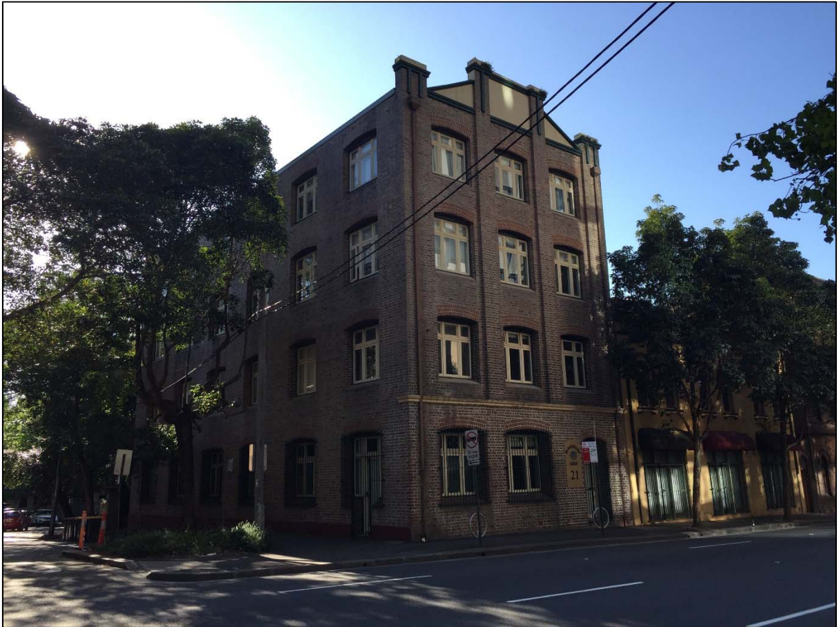
Figure 11: 13-21 Abercrombie Street (source: DPE)
