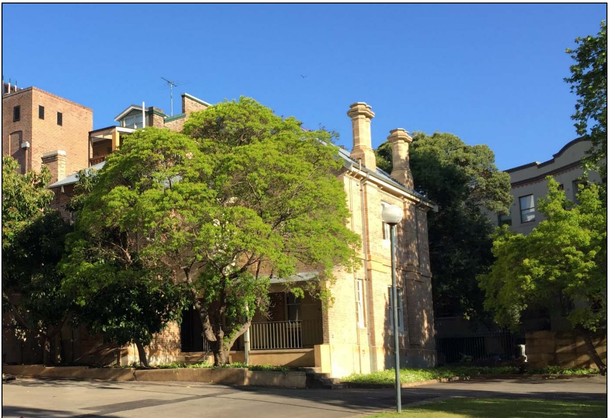
Figure 6: Former Headmaster's residence (CB27) (source: DPE)
