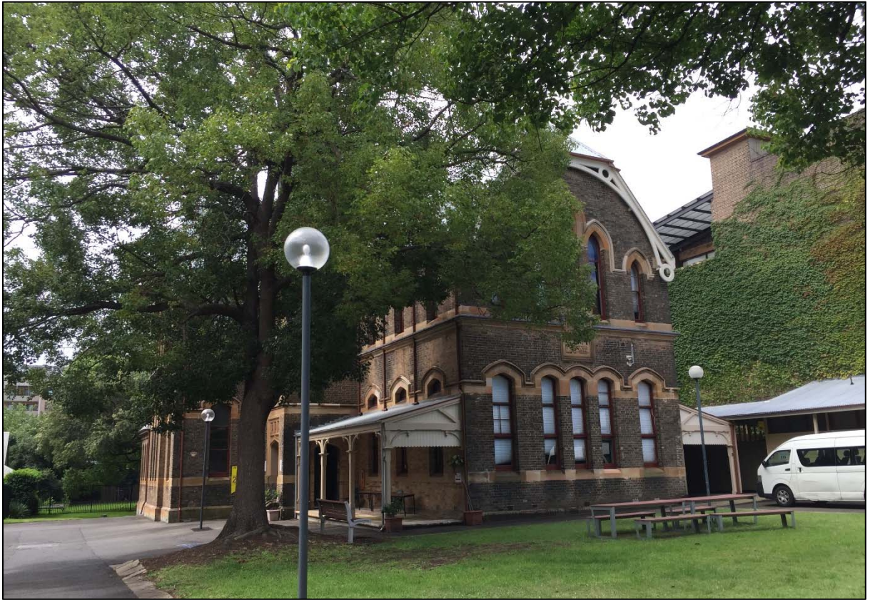
Figure 5: Former Boy's School building (CB25) (source: DPE)
