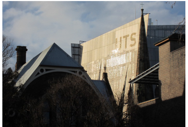
Fig.1. UTS Blackfriars Site with Main Campus UTS Campus in the background and CB25 in the foreground
