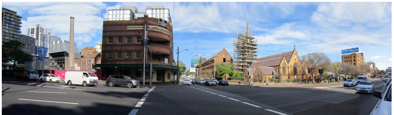
Fig.4. View toward site from the corner of Broadway and Abercrombie Street beside UTS CB11 / FEIT Building
