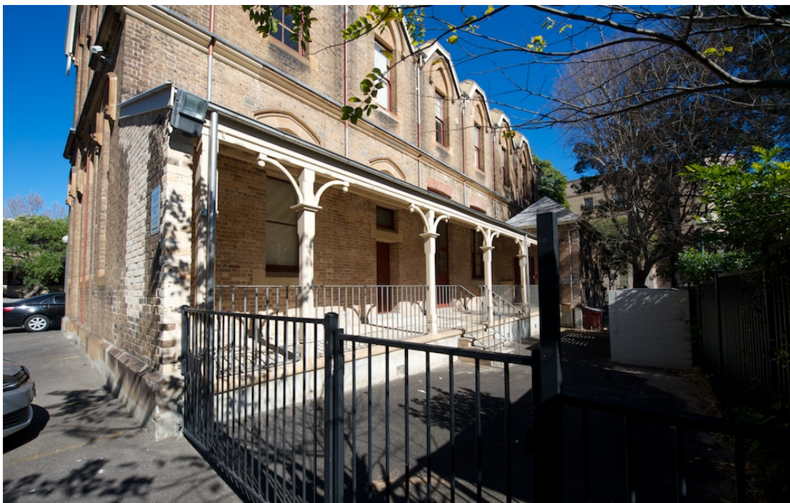
Illustration 16 The façade of one of the school buildings that would front the new development. Sufficient distance is required between buildings to allow the verandah to properly function, for solar access and to create a good outdoor space between buildings that encourages interaction across the area.
