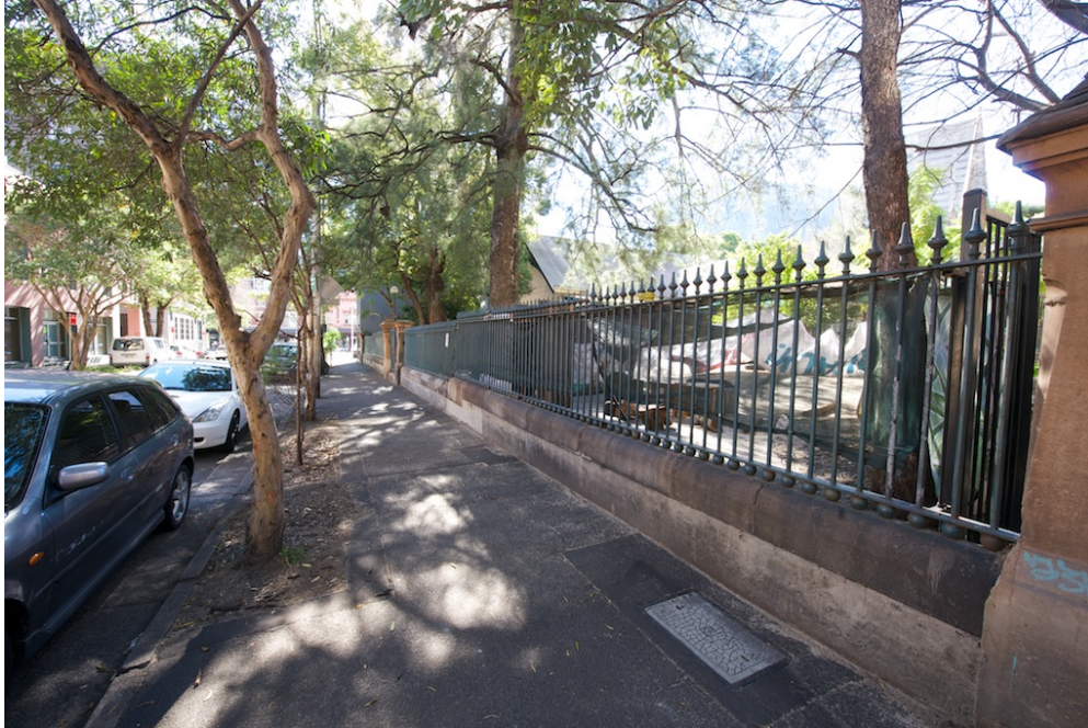
Illustration 9 The site frontage to Buckland Street. The setback options provide that either most of the fence would remain and the building would be set back so that the green street edge and openness of the street frontage is retained or the building could be built to the street edge interpreting the fence plinth and alignment. A new major site entry is proposed in the immediate foreground.
