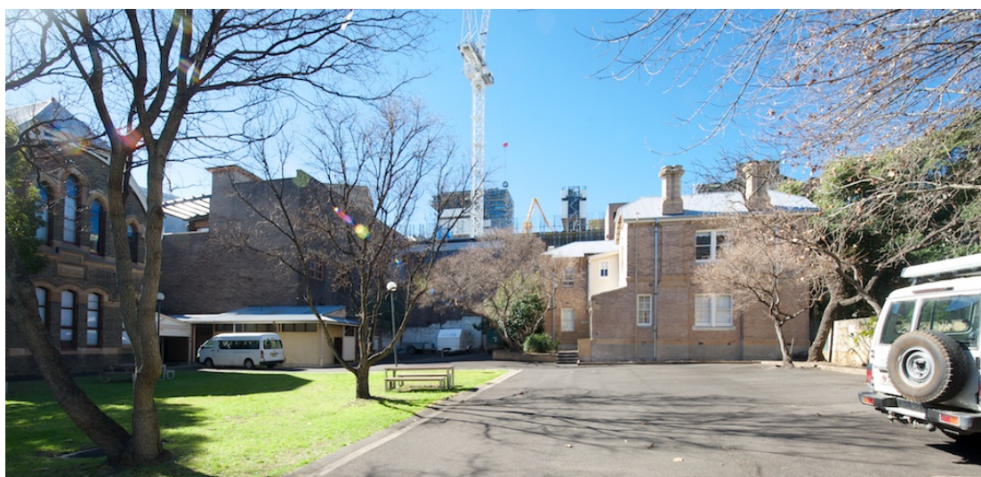
Illustration 12 View from within the site looking east with Central Park rising in the background. The backdrop of high-rise in this location removes any sense of an open sky view across the site. The proposed building will sit comfortably against the much higher scale of Central Park. This is the location of the approved single storey child care centre.
