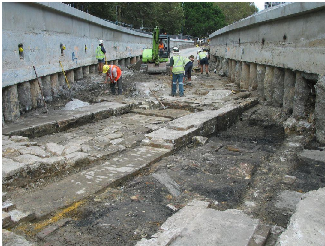
Figure 3.3: Foundations of Barker's Mill, uncovered during archaeological investigations by Casey & Lowe in 2004.
