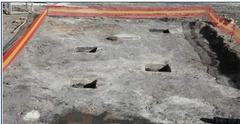
Figure 2.4: Test excavations in alluvial sands and silts at the Dr Chau Chak Wing Building
