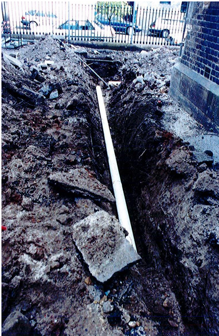
Figure 4.19: Trench 4, southwest corner behind Girls school showing sandy deposits. Photo taken looking west, BLKF 5.11.
