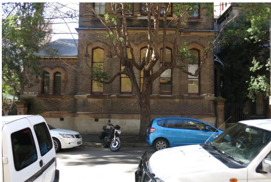
Figure 4.2: Detail of Girls and Infants School Building, showing height above Buckland Street. Looking east.
