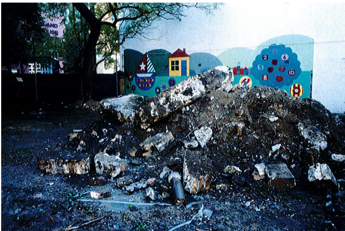
Figure 4.24: Mounds of dirt containing brick and concrete slabs that formed the footings of the toilet block. Photo taken looking northwest, BLKF 3.36.
