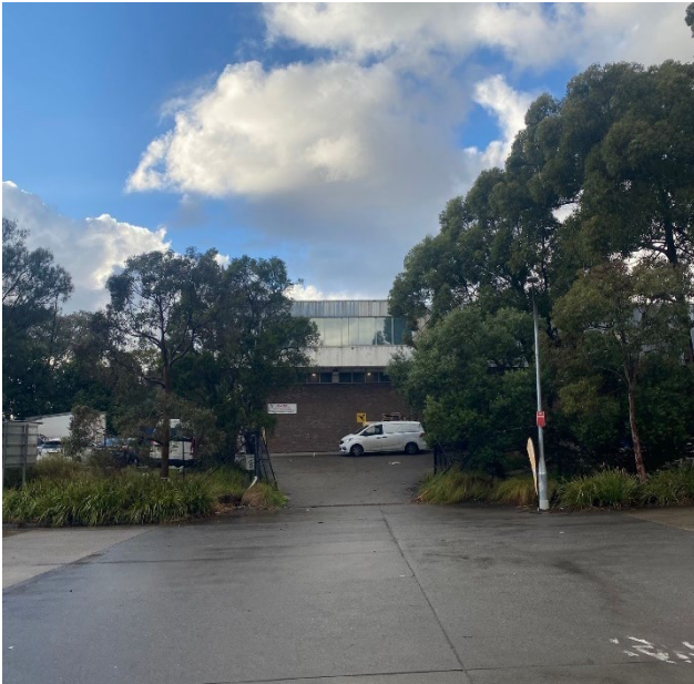
Picture 1 Western edge of site on Blaxland Road
