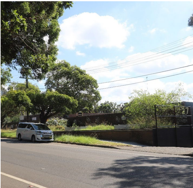
Picture 3 South-east corner of the site
