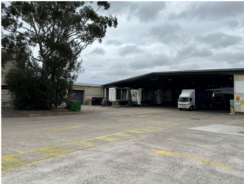
Figure 1.19 South-west view of the truck bays at the centre of the subject site on Percival Road. South-west facing.
