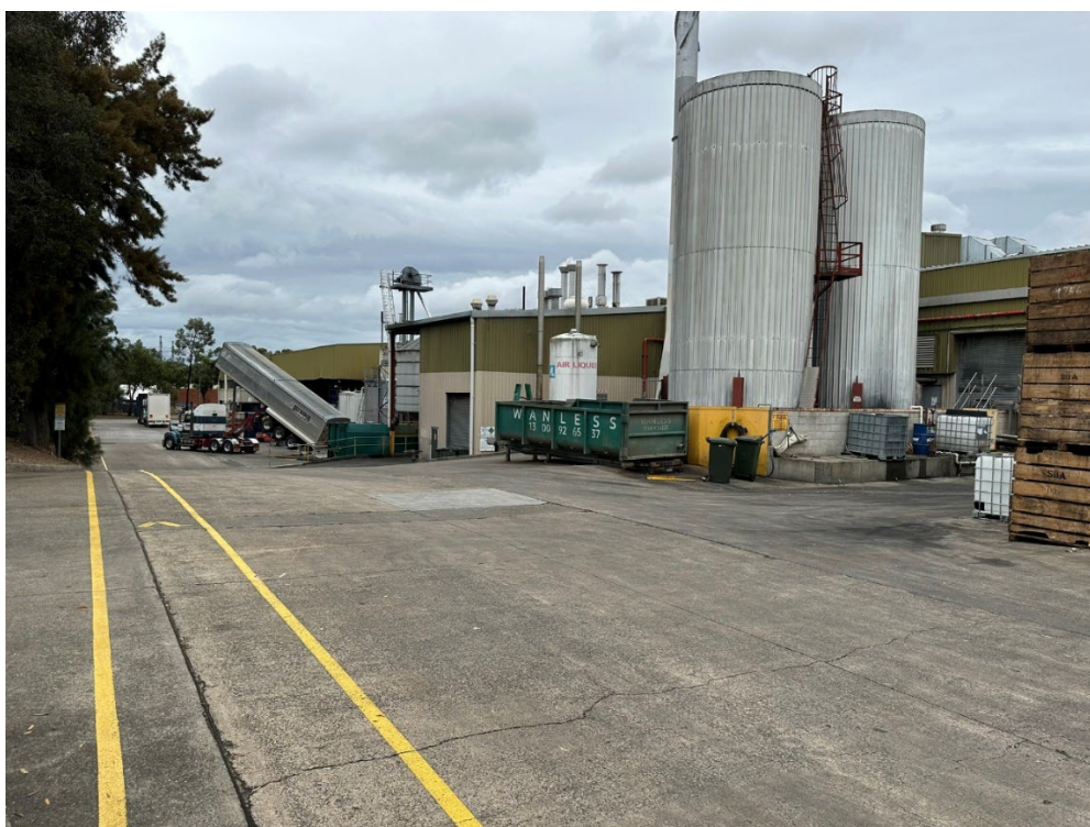
Figure 1.14 South-west truck drive along the eastern side of the Snack Brands building on Britton Street.
