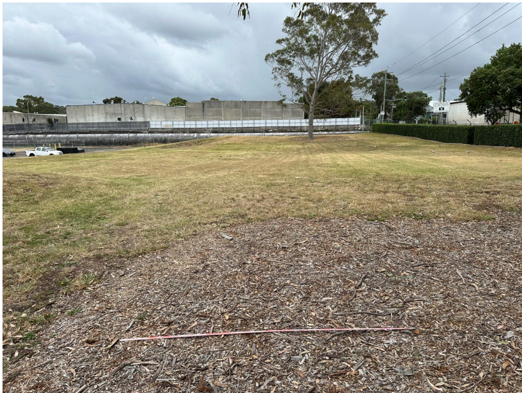
Figure 1.21 North facing view of the pipeline that is part of the Lower Prospect Canal Reserve Heritage Item adjacent to the Percival Road subject site (2m scale).
