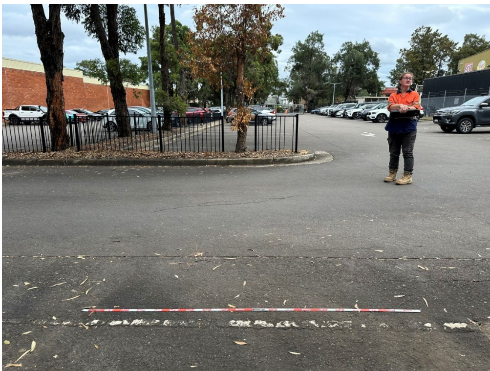
Figure 1.13 West facing view of the parking area at the southern end of the Britton Street subject site (2m scale).
