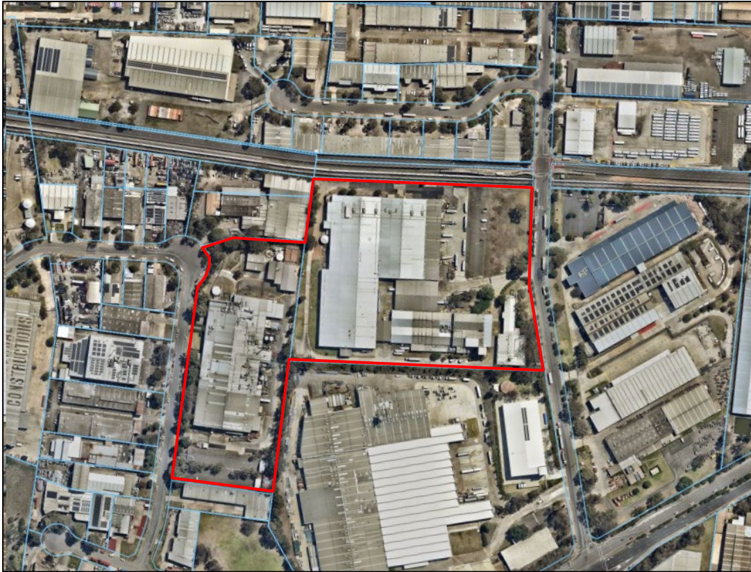
Figure B: Existing Site Context and Surrounding Area (Source: NearMap, 2023)
