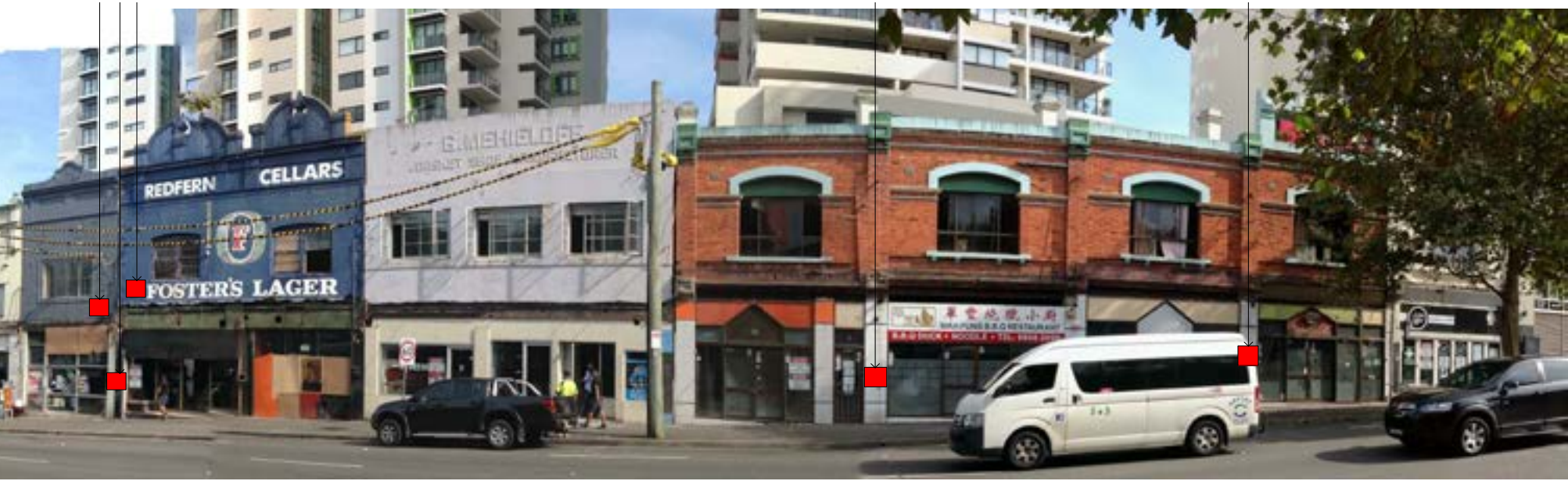
PHOTOGRAPH OF REGENT ST EXISTING FACADES
