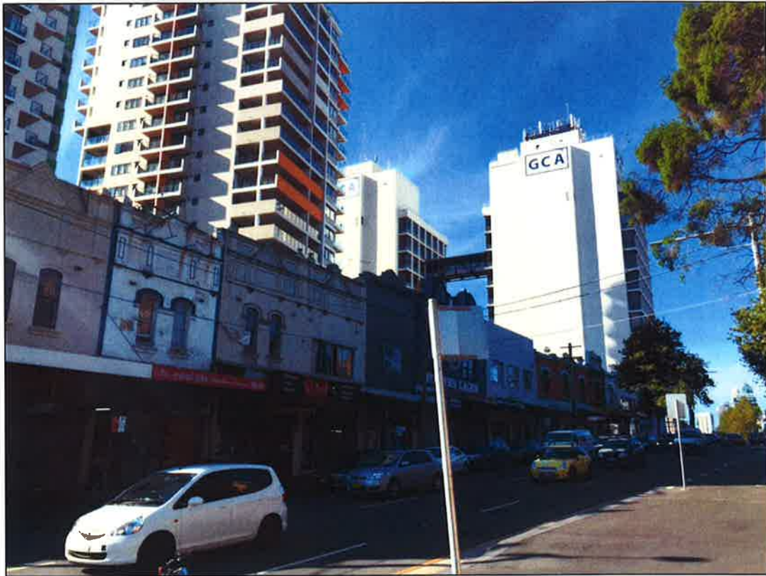
Facades sought to be retained from Regent Street.
