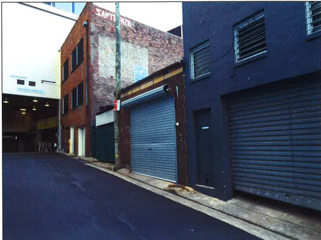
Location of rear loading dock and entry to 157 Redfern Street
