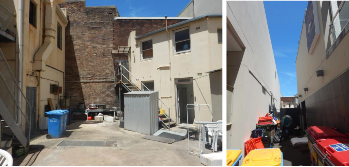
Figure 15: Rear of 68 Regent Street contains an external bathroom.
