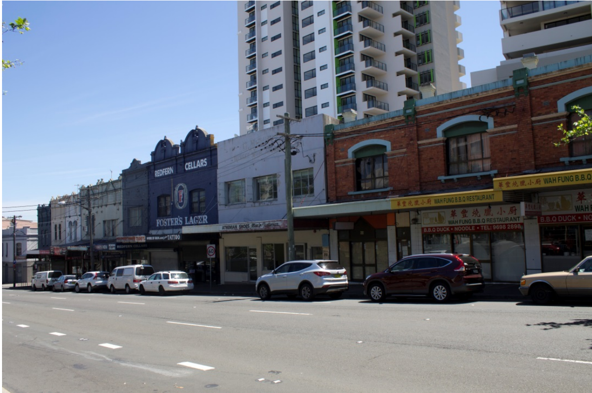
Figure 7 – Site (extending from far right to Redfern Cellars) viewed from Regent Street Source: JBA
