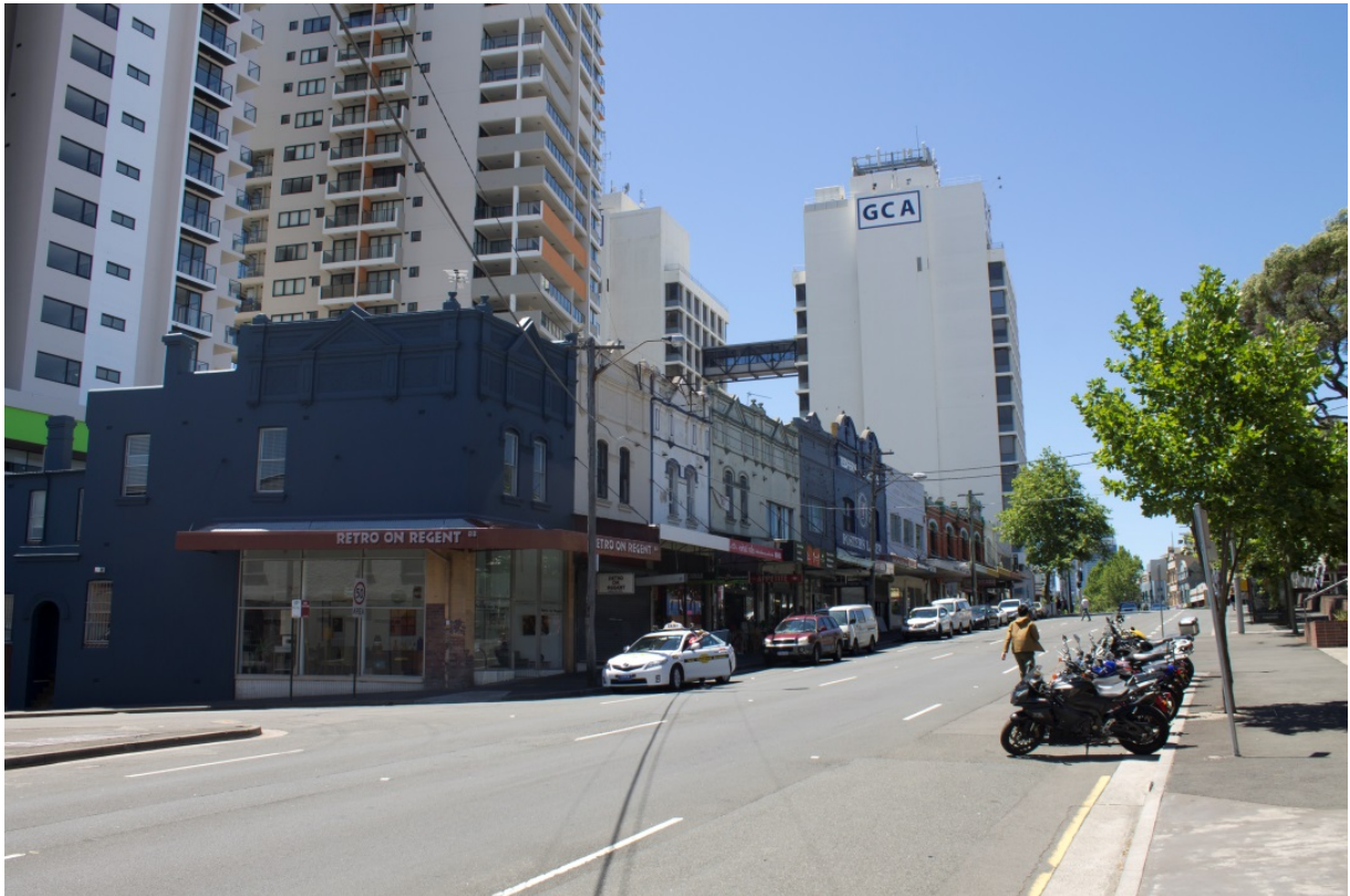
Figure 9 – Development on Regent Street, with Site and adjoining towers in background Source: JBA
