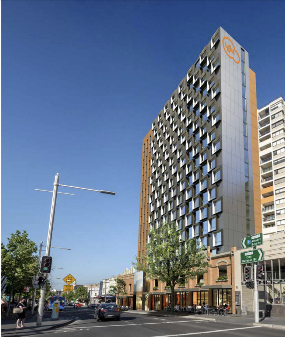
Figure 19 – Photomontage of proposal viewed from Regent Street/ Redfern Street intersection Source: Bates Smart
