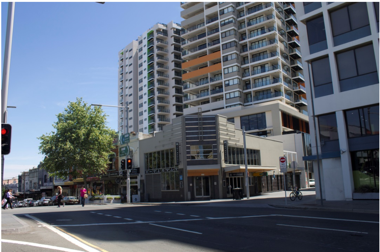
Figure 10 – Regent Hotel viewed from north, with site and adjoining towers in background Source: JBA
