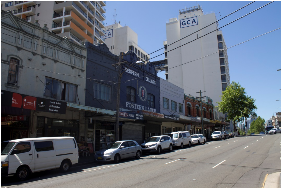
Figure 6 – Site (extending from Redfern Cellars to the right) viewed from Regent Street Source: JBA
