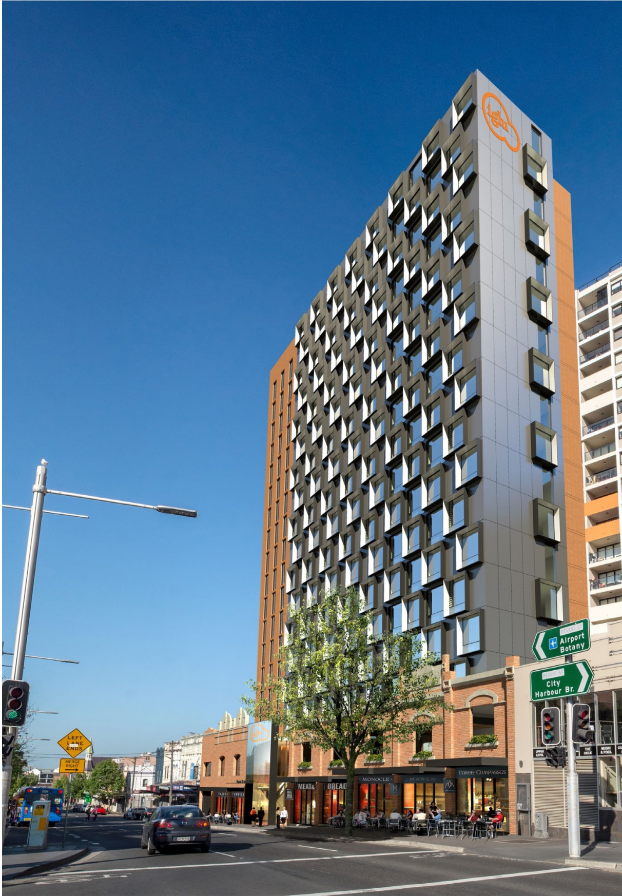
Figure 12 – Photomontage of proposal viewed from Regent Street/ Redfern Street intersection Source: Bates Smart
